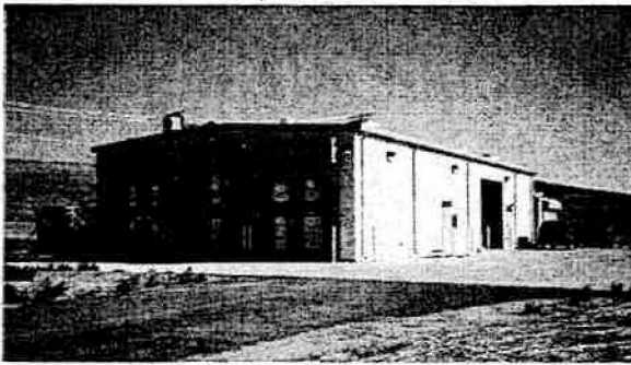
Figure 6 New Onsite Water Treatment Plant
