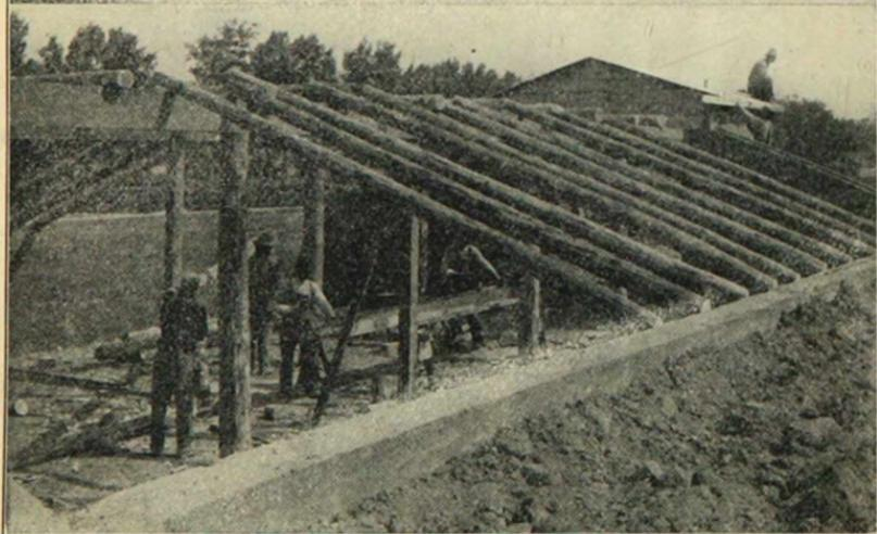
PLATE, XVI.—The Station Cellar. Excavation. Braced Concrete Forms. Framing the Roof.
