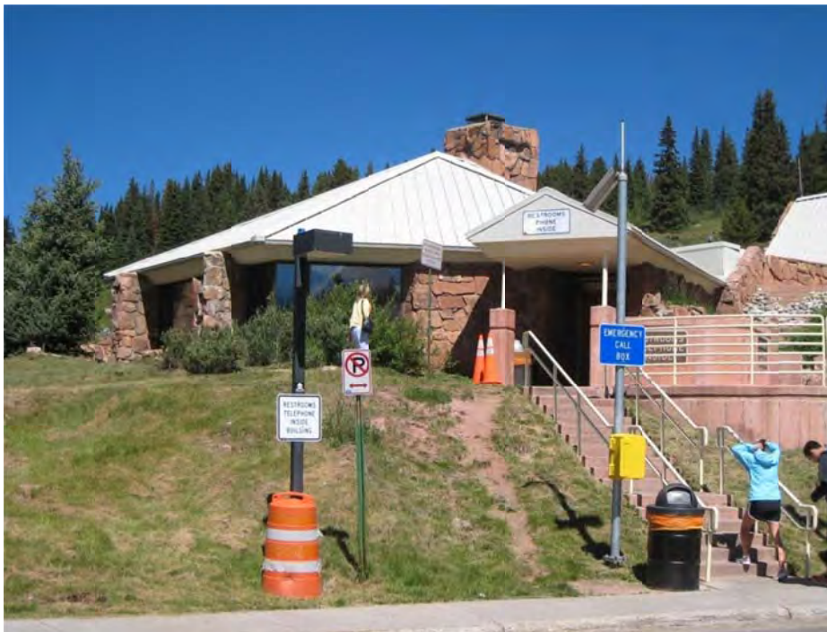
Figure 18. Vail Pass Rest Area Restroom Structure
