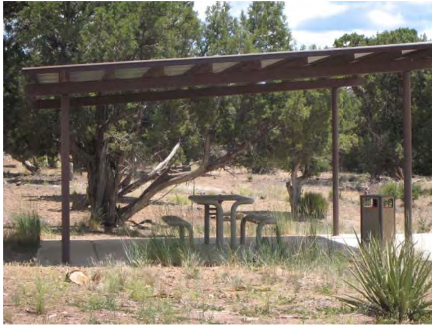
Figure 29. Sleeping Ute Mountain Rest Area Example of Picnic Shelters in Rest Area
