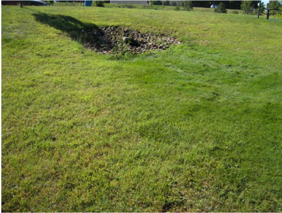
Figure 4. Sterling Rest Area Stormwater Basin
