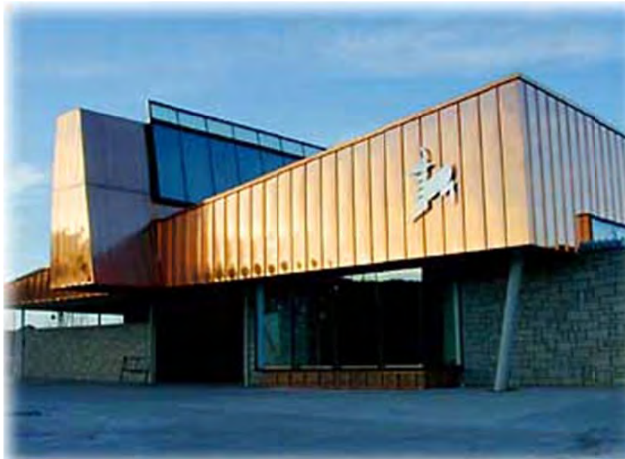
Figure 22. El Moro Rest Area Entrance Area with Copper Siding and Roof
