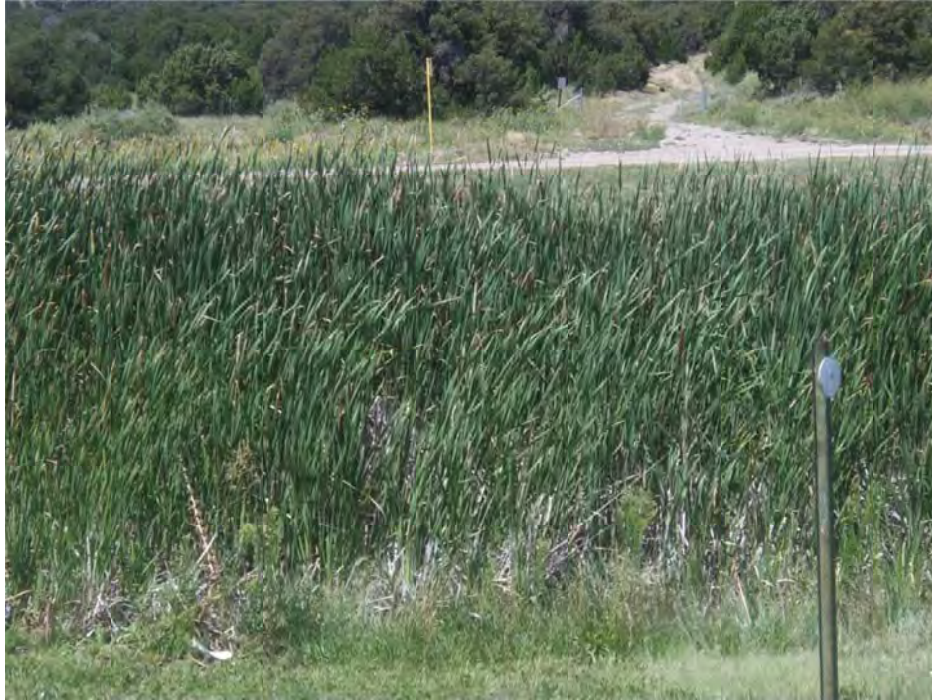
Figure 25. El Moro Rest Area Stormwater Ponds with Wetland Vegetation
