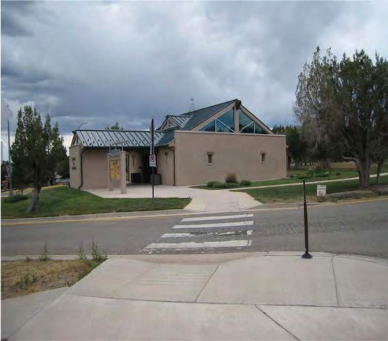
Figure 28. Sleeping Ute Mountain Rest Area Restroom Structure
