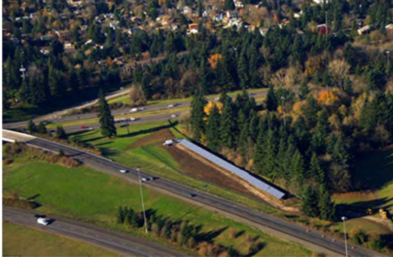
Figure 31-h. Aerial view of ODOT 'Solar Highway' Site at I-5/I-205
