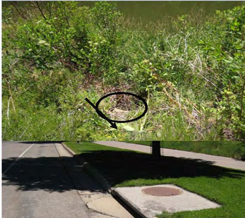
Figure 14. Hanging Lake Rest Area Unprotected Stormwater and Vegetated Ditch
