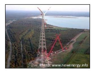
Wind speed increases as one gets further away from the ground. Bushes, trees, and relief in the landscape create turbulence that slows down the wind. In general, for flat land covered with most crops, a turbine with a hub height of 30 m will produce about 20% more power than a turbine set at 20 m.
