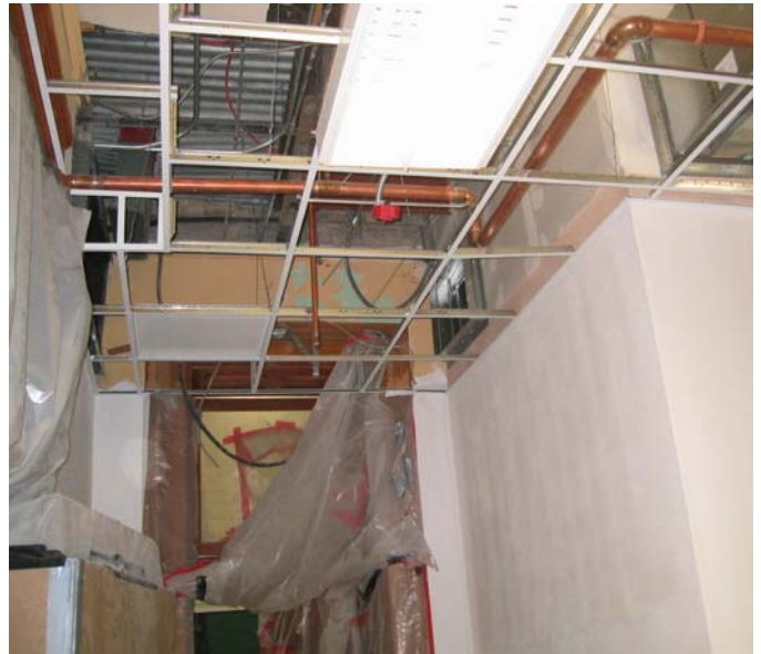
033 Construction photo showing the metal decking of a former patch
