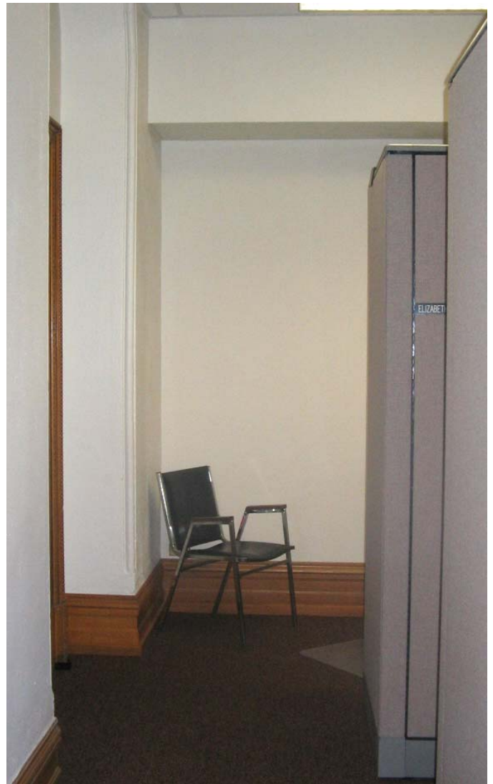
036 Soffit illustrates difference between former and new east wall
