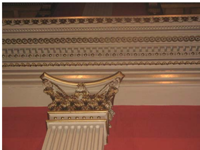
Supreme Courtroom Chamber plaster cornice detail
