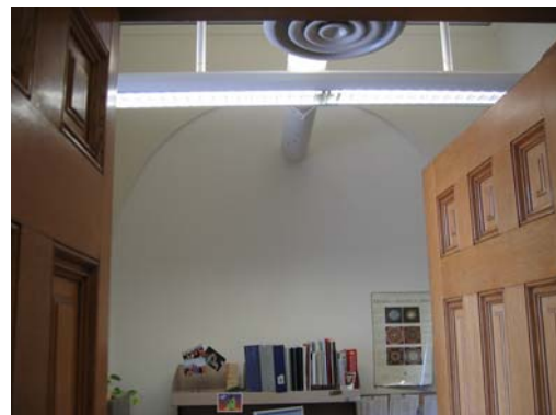
085A View of in-filled archway on west wall
