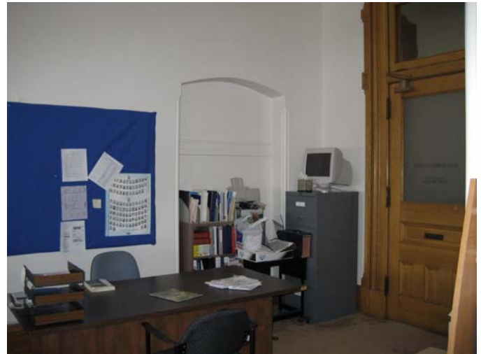
223 View of northeast corner and in-filled arch
