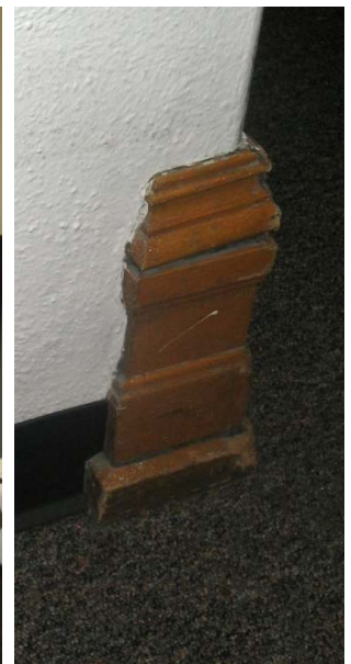
060 Base transition and at former vault door
