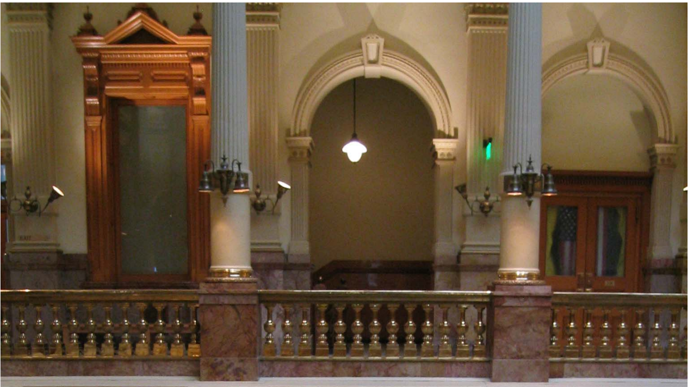
Overall view of the Third Floor Arcade, north side, showing in filled arched opening with relocated original doors
