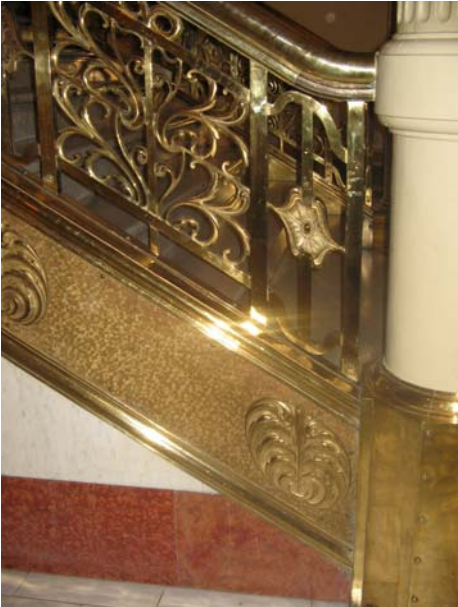
Basement Rotunda stair brass railing
