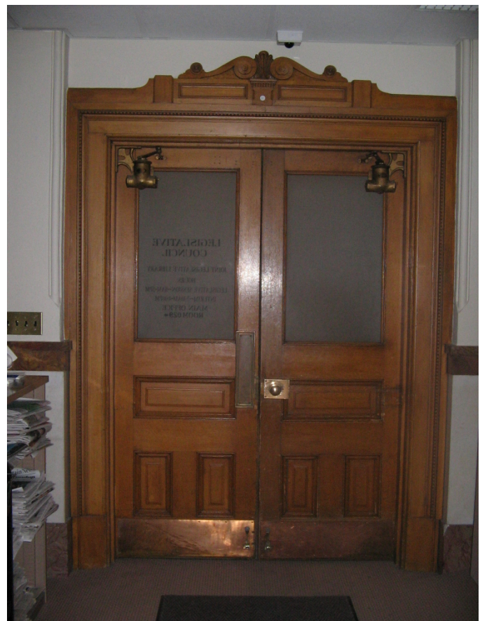
048 Relocated door in Rotunda archway
