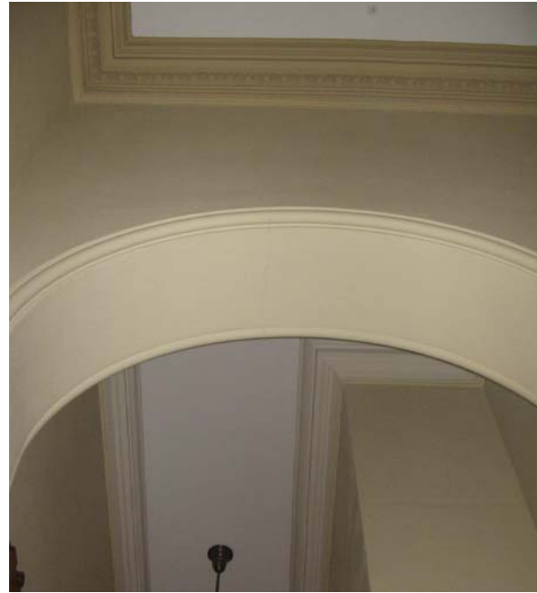
315 Corridor ceiling and corded arch detail
