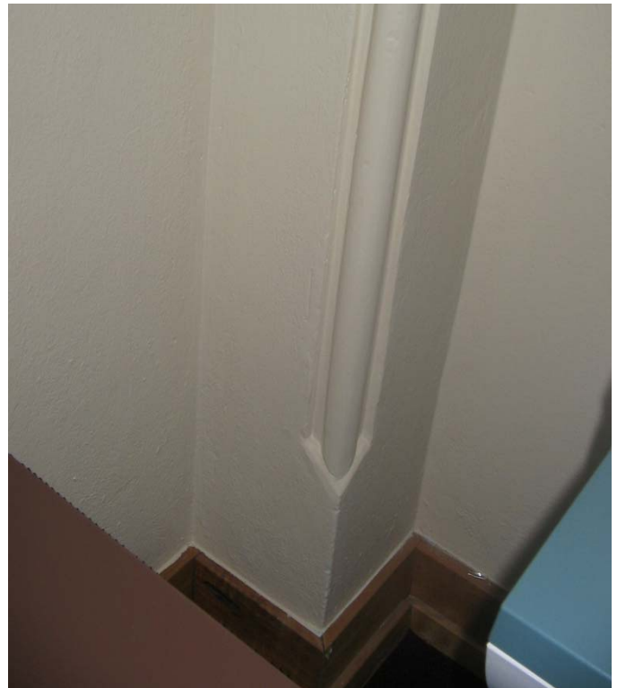
158 Corded corner at southeast
