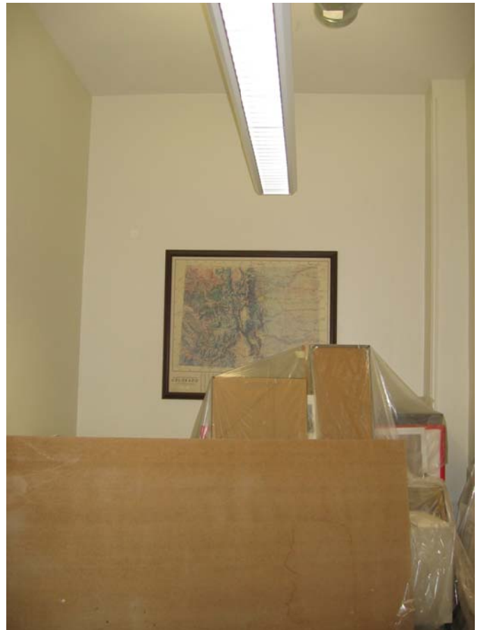
0106 View of south wall and original archway
