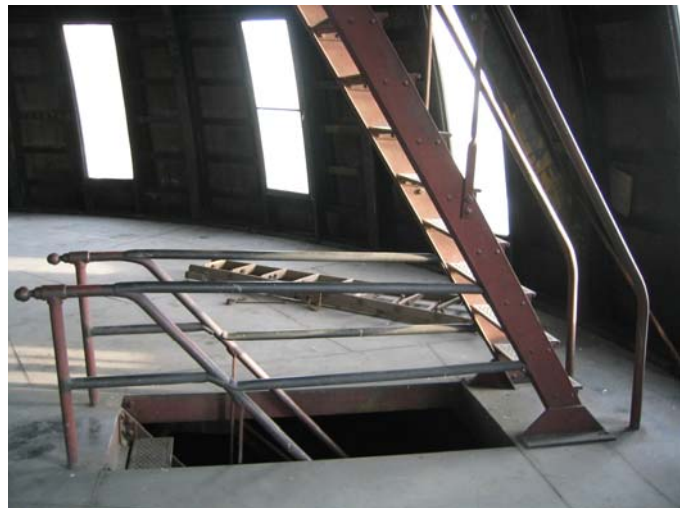
Upper Dome access
