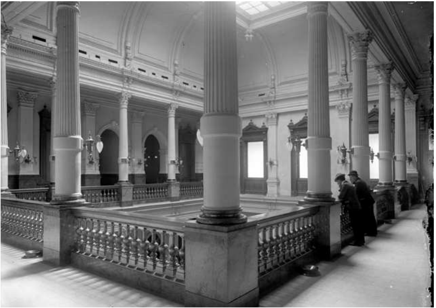
Historic photo of overall view of the Third Floor Arcade, south side, showing no stained glass, original lamp shades and double arched opening shown
