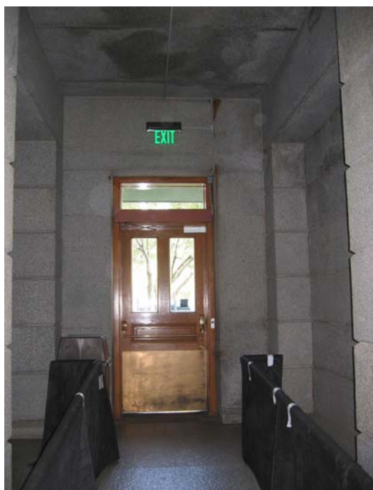
Basement exterior doors
