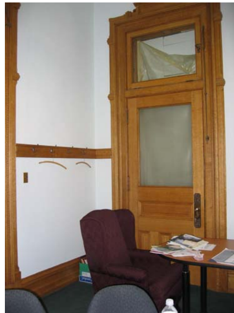
341 Northwest corner with inoperable door to Room 342
