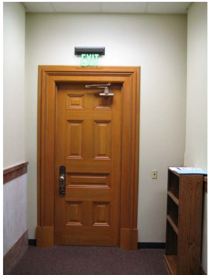
039 New door and frame, hardware installed in 2005
