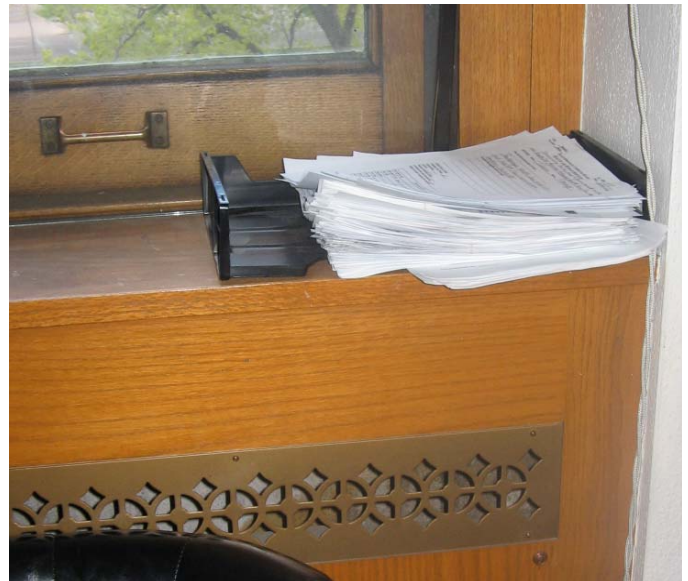
263 Modified window trim and non-original radiator panel detail
