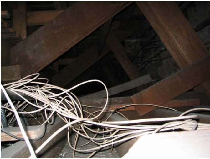
Space above the House Vestibule ceiling
