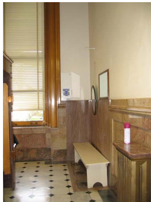
129 View south with original flooring and men's toilet basins
