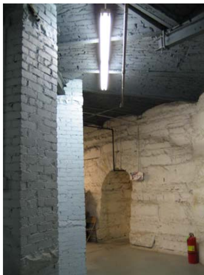
Sub-Basement Rotunda walls
