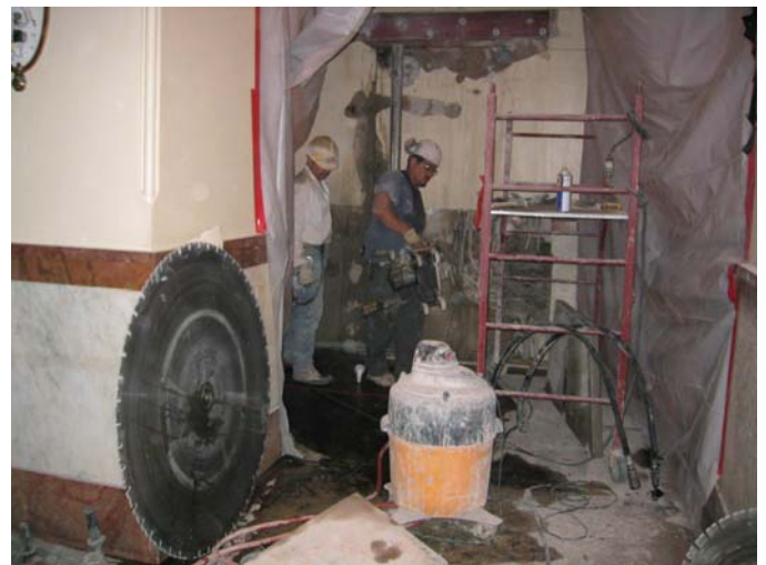
Cutting opening in Basement masonry wall for Northwest Stair
