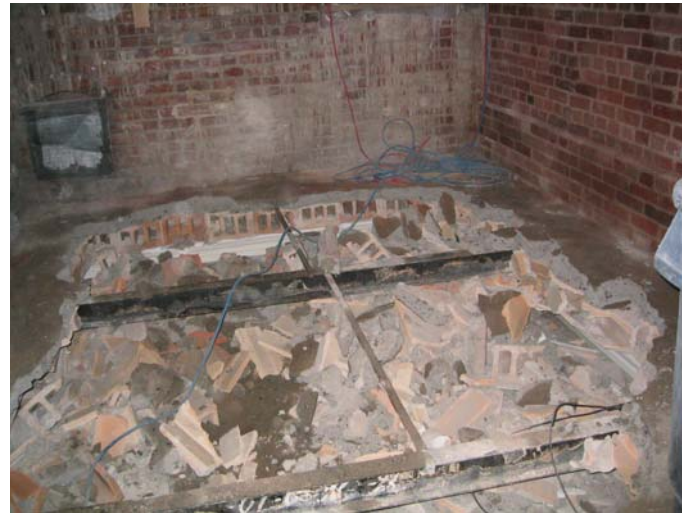
Removal of attic floor for extension of Northwest Stair
