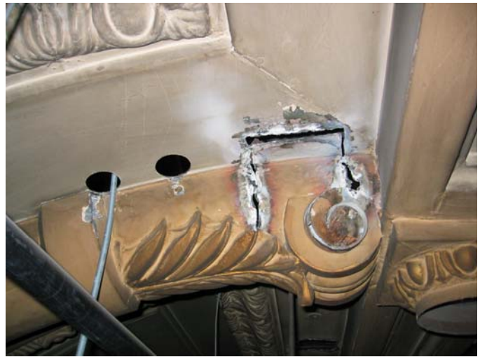
Attic: Senate Chamber skylight, damage from a cutting torch
