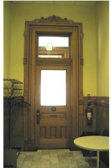
334 Door to Room 332
