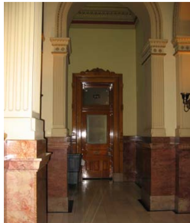
125 View of entry door to Room 125 from Arcade 165
