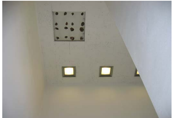
262 Existing ceiling and recessed fluorescent fixtures
