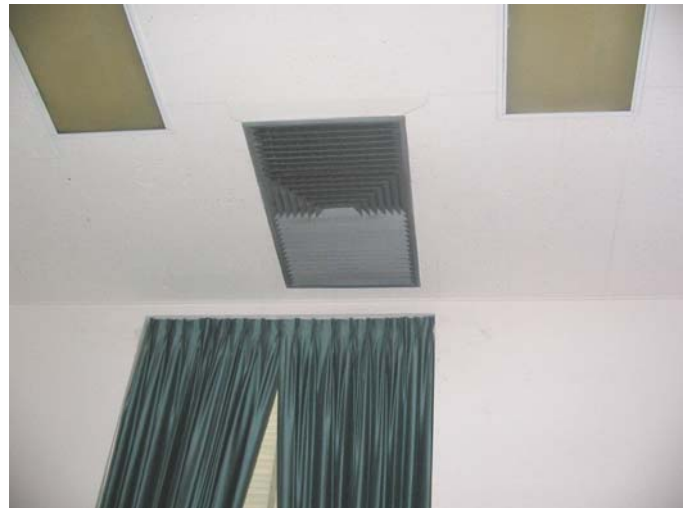
246 Existing ceiling and window detail
