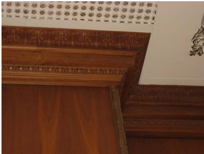
136C Crown molding and decorative plaster ceiling detail
