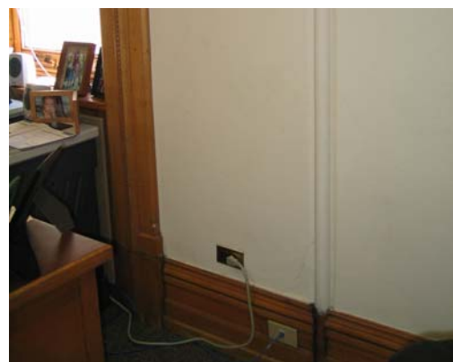
085A Corded plaster on south wall
