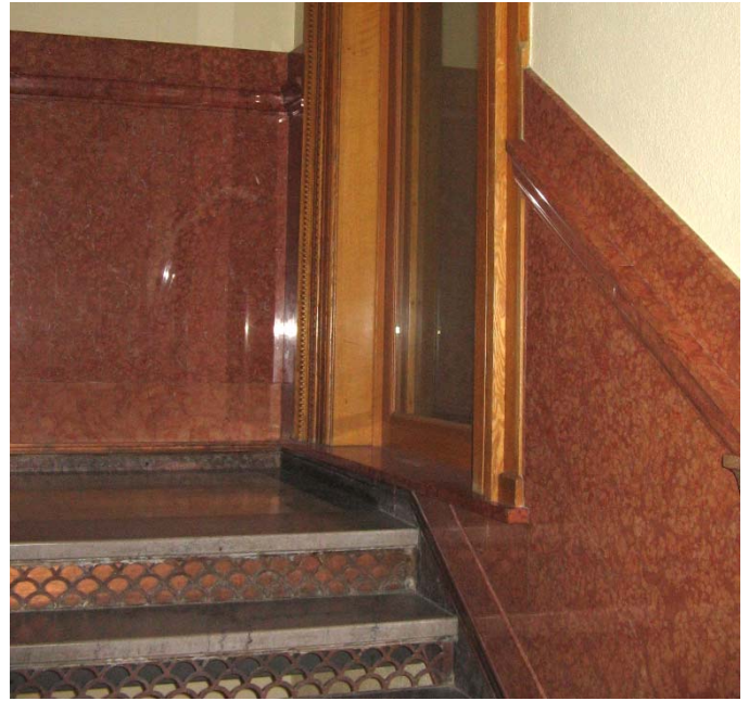
New stone sill and wainscot at Second Floor Northwest Stair
