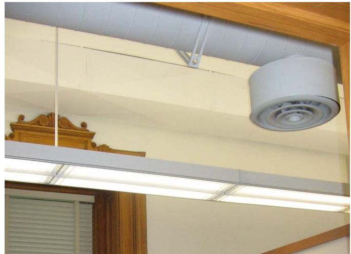
056 Exposed ductwork and partial height wall
