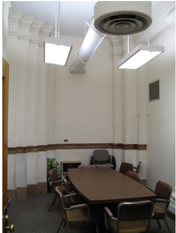
071 View looking north
