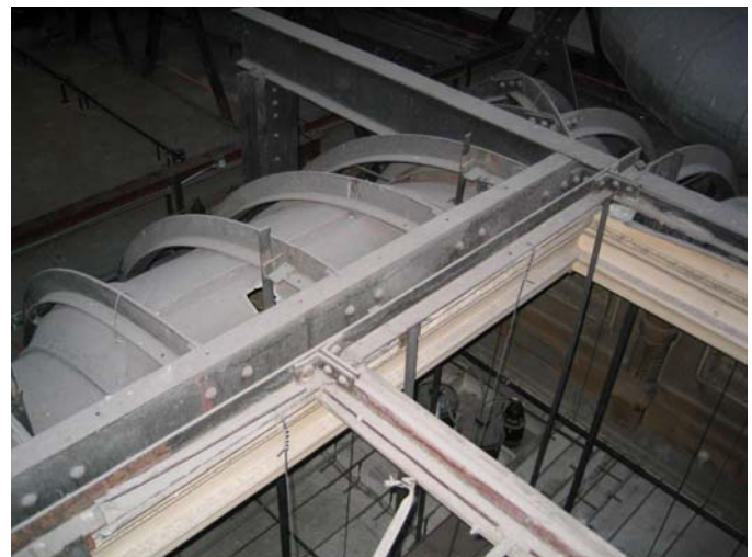
Looking into original House Chamber skylight from Attic
