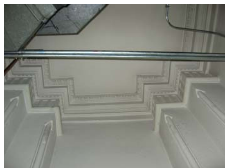
115 Ceiling detail and corded pilasters
