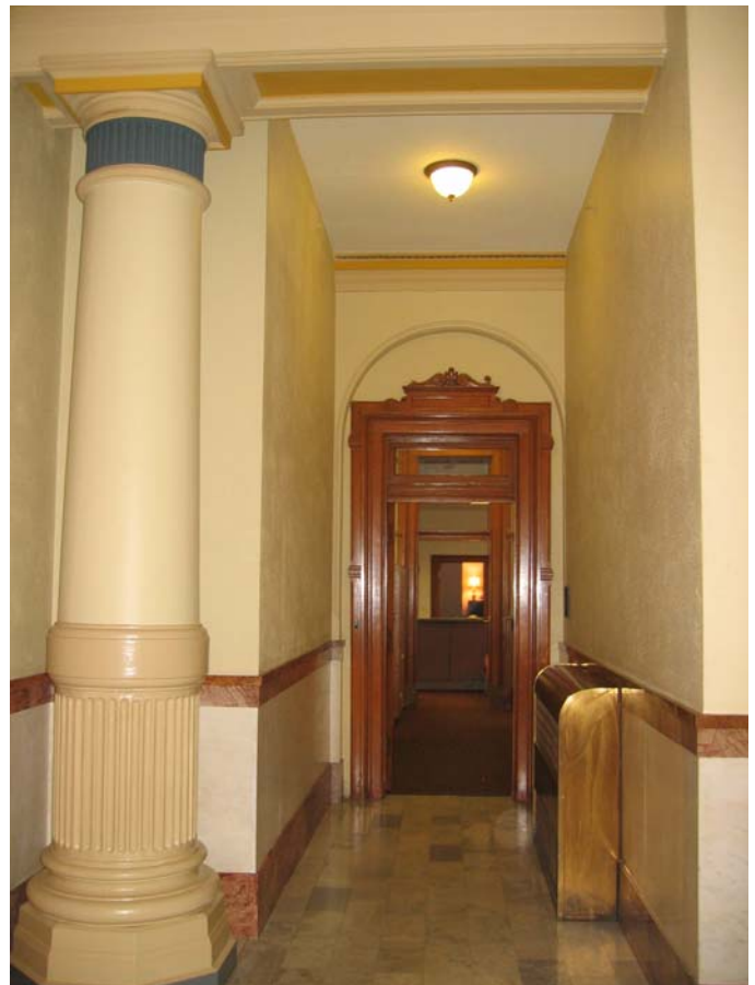
Hallway 029 off North Basement Corridor with original radiator
