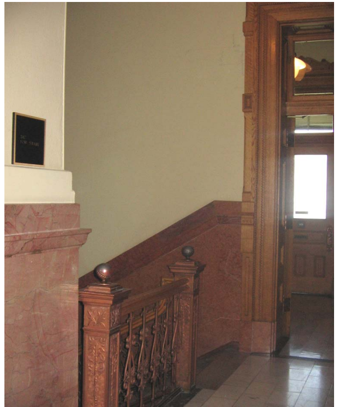
Existing railing Southwest Stair, Third Floor
