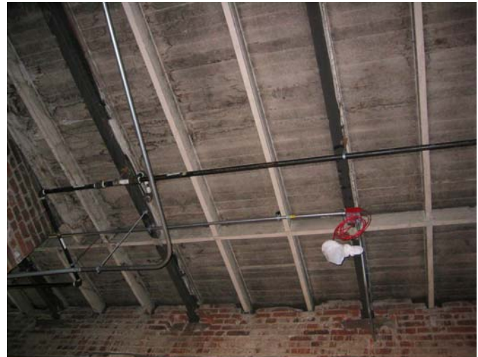
Roof decking and wood purlins
