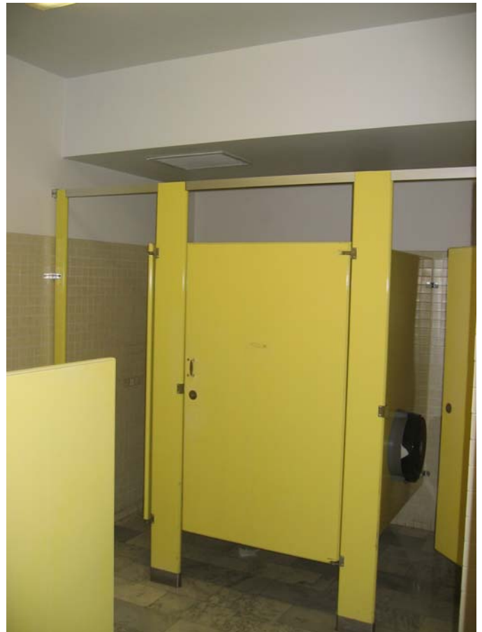
098A View of south wall
