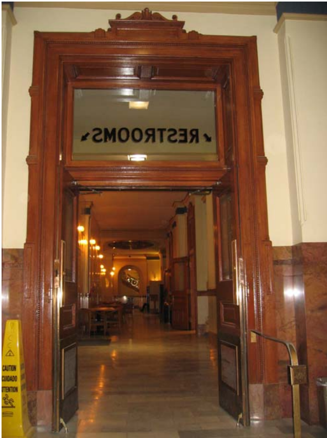
Remaining North Entry Vestibule door
