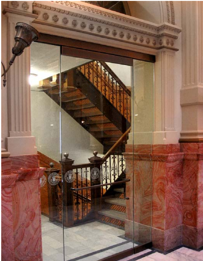
New header and glass door with side lights at Third Floor
