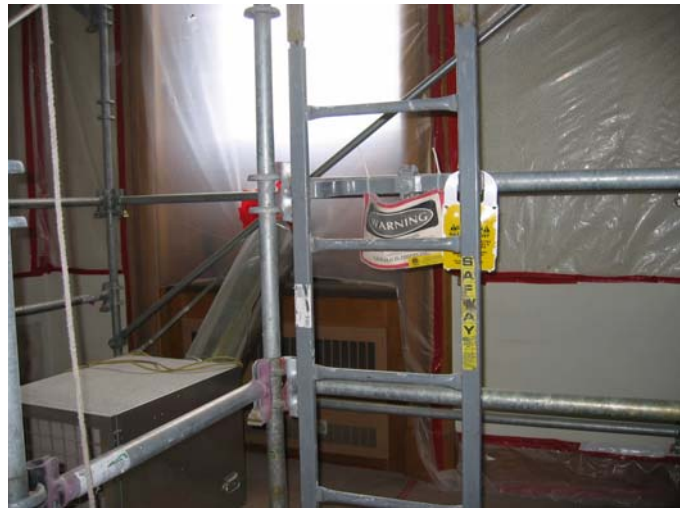
110 View towards exterior window protected during the Life Safety Project
