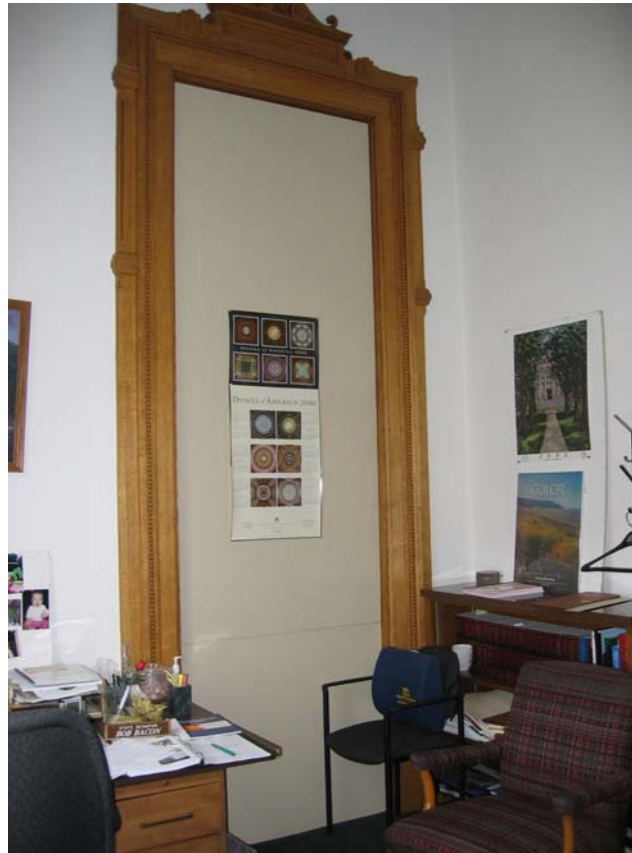
342 In-filled fabric wrapped panel on south wall door to Room 341
