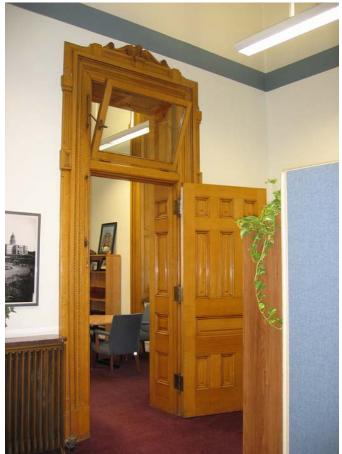
121 Door to Room 121A with freestanding radiator with Cedar marble top
