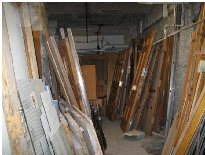
Sub-Basement room of removed trim and doors
