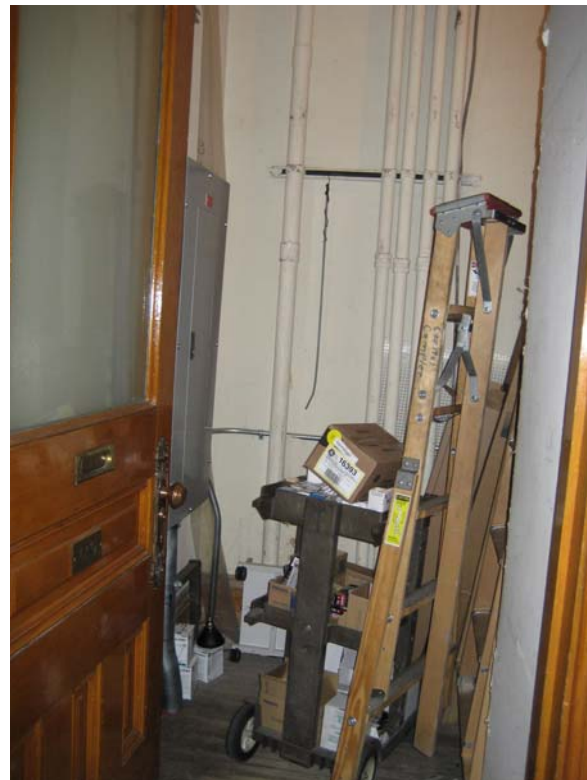
059 View looking in from Arcade
