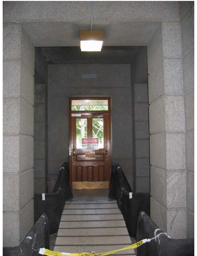
Basement North Entry Vestibule looking west
