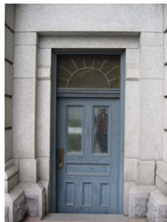
0116 Exterior door from outside
