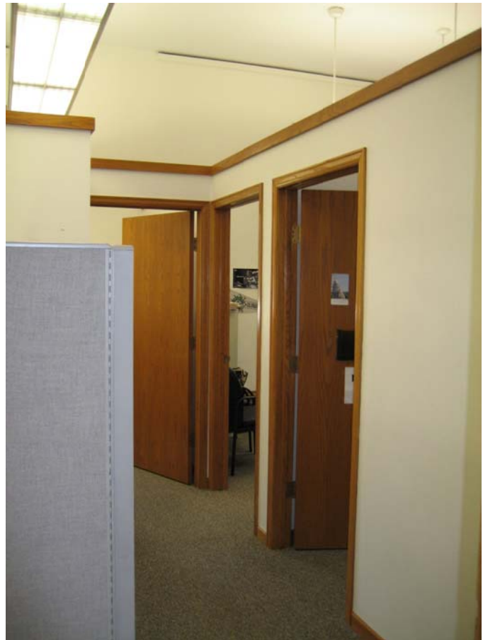
081 View looking south towards 081A, 081B, and 081C
