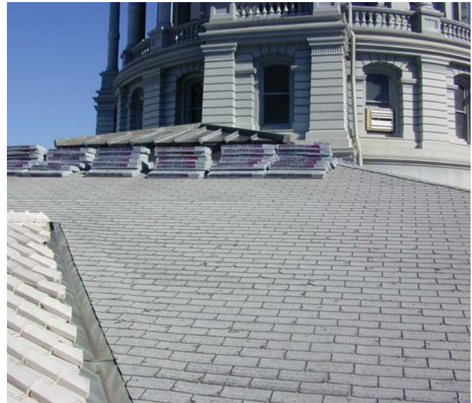
Partial view of roof
