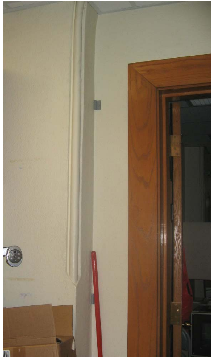
043 Arch with original wainscot removed
