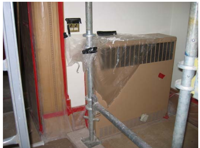
116B Freestanding non-original radiator in the southwest corner
