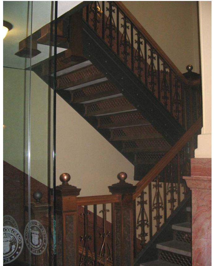
New bronze Northwest Stair at the Third Floor
