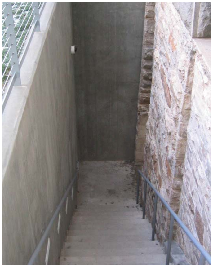
New exterior Northwest Stair
