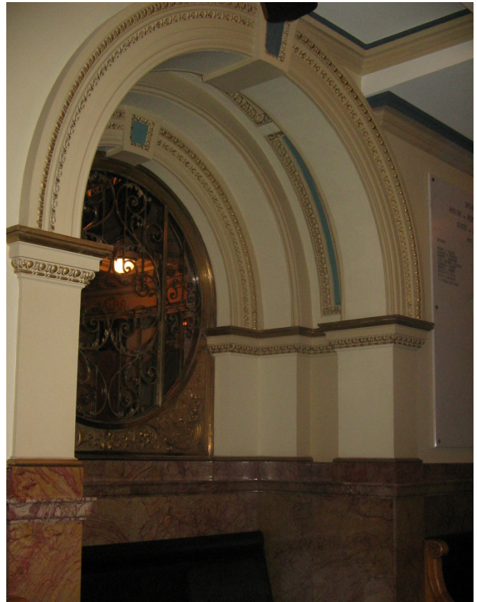
House Chamber bronze grille infill in arch looking into Rotunda
