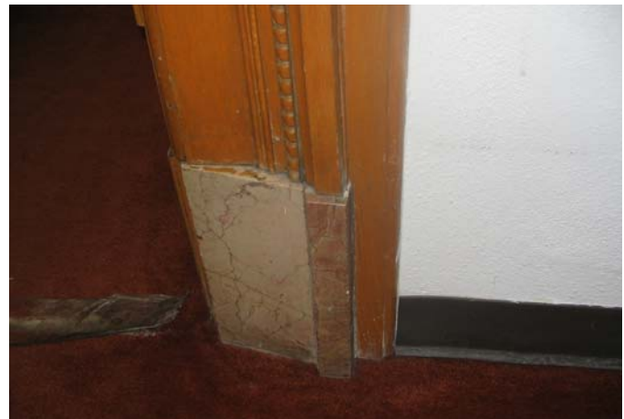
017 Stone plinth on the relocated original door
