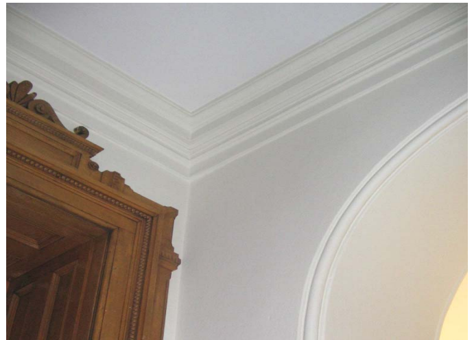
090 Existing conditions at southwest corner
