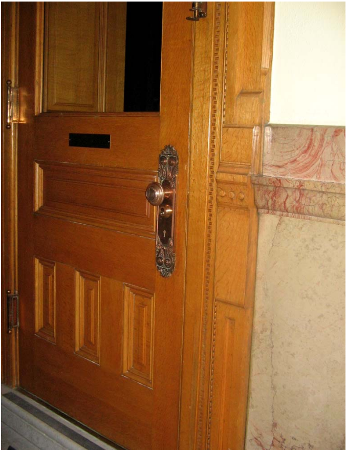
226 wainscot termination detail and typical door hardware
