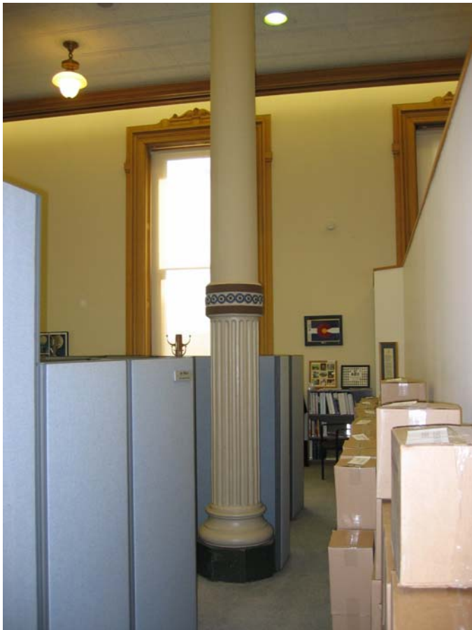
271B Cast iron column
