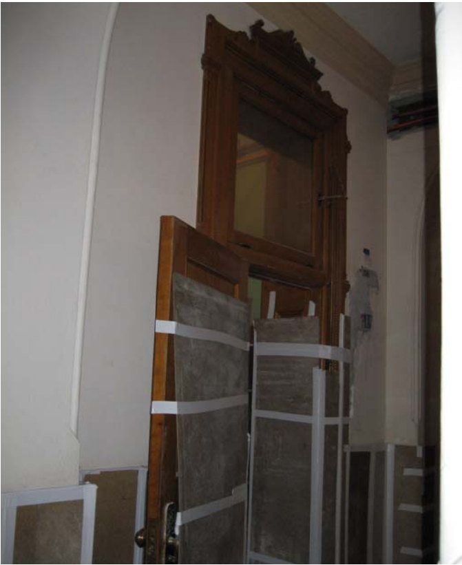
007 View of door to room 018
