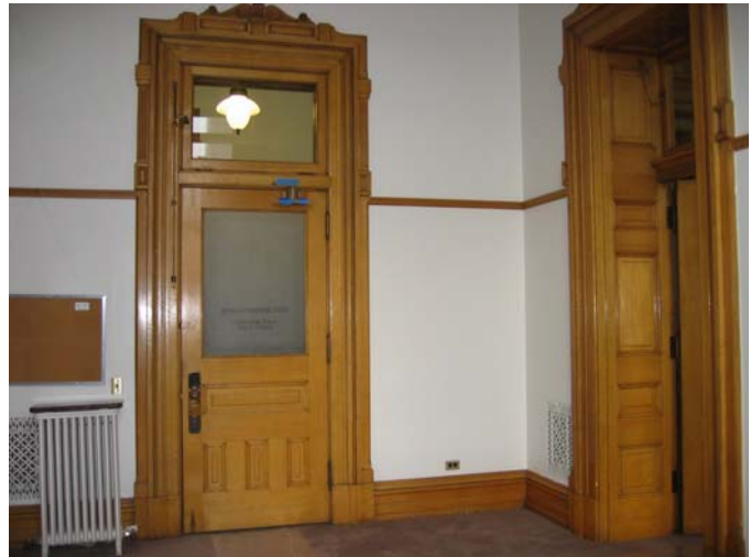
202 Door to corridor
