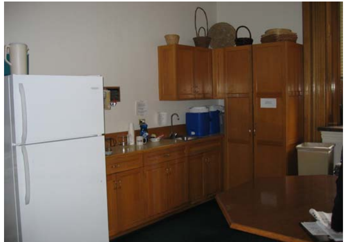
229 Non-original cabinetry in the southwest corner
