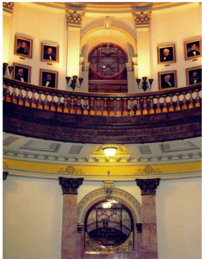
Openings from Rotunda into House Chamber, Second and Third Floors
