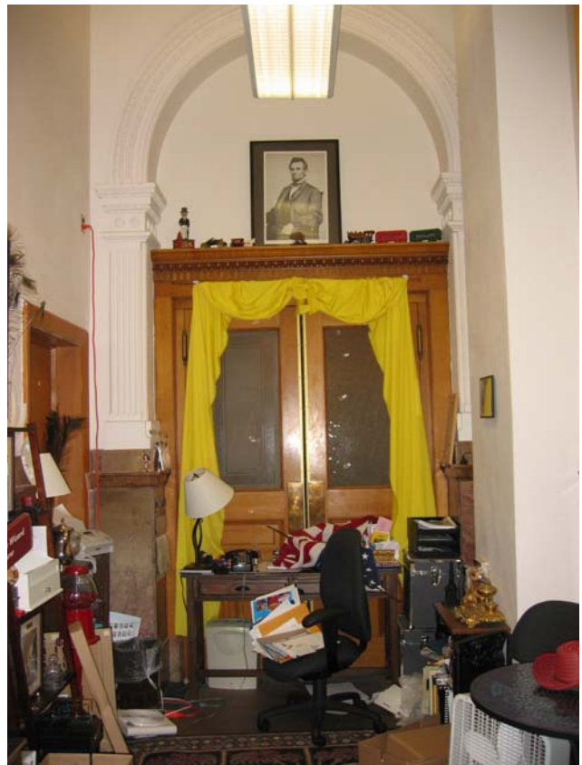
308 Non-original header and door location, west wall
