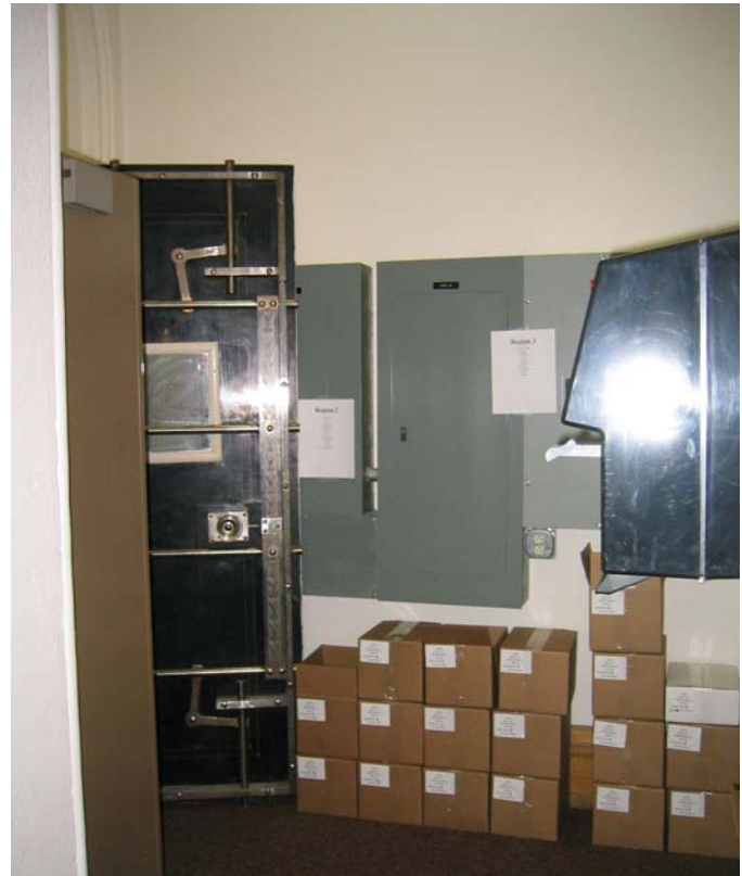
031A South wall showing panels
