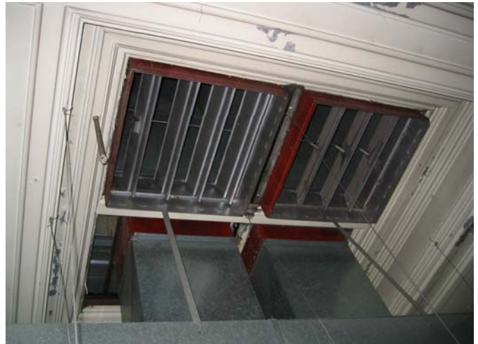
357 Former skylight now serving mechanical functions
