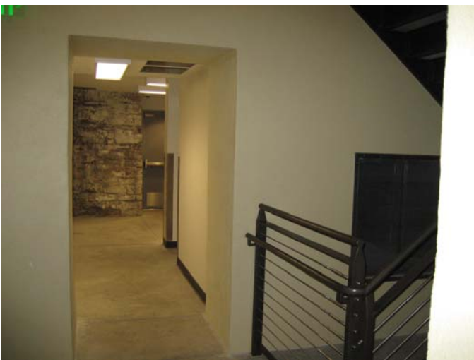
Northwest Stair to Sub-Basement SB99
