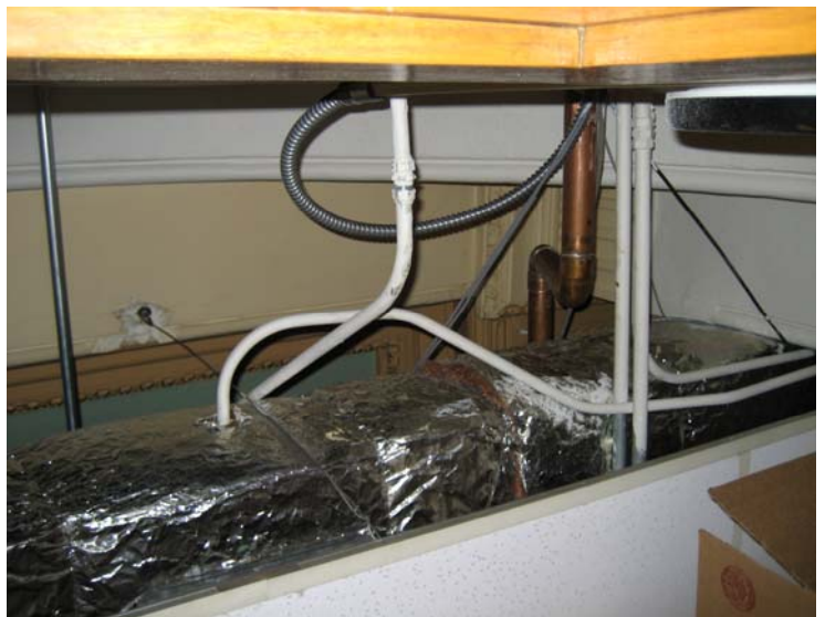
048 View above ceiling showing original ornate ceiling and pilaster capitol
