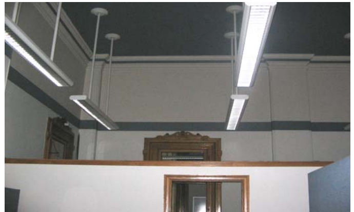
120 View over partial height wall
