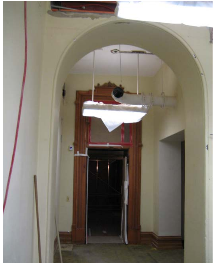
010 Original archway on west wall
