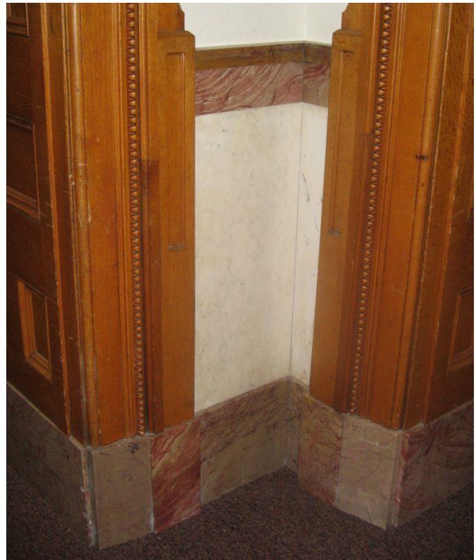
029A Stone wainscot and plinth base at door frames
