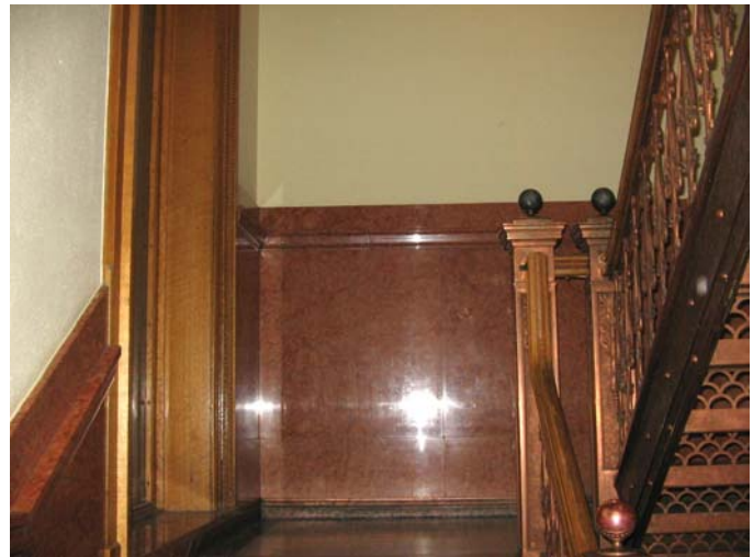
Existing landing at Southwest Stair
