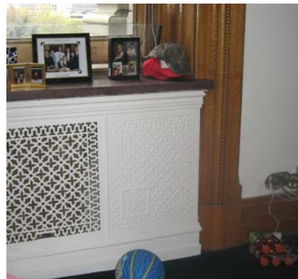
227 Original radiator with cedar marble sill
