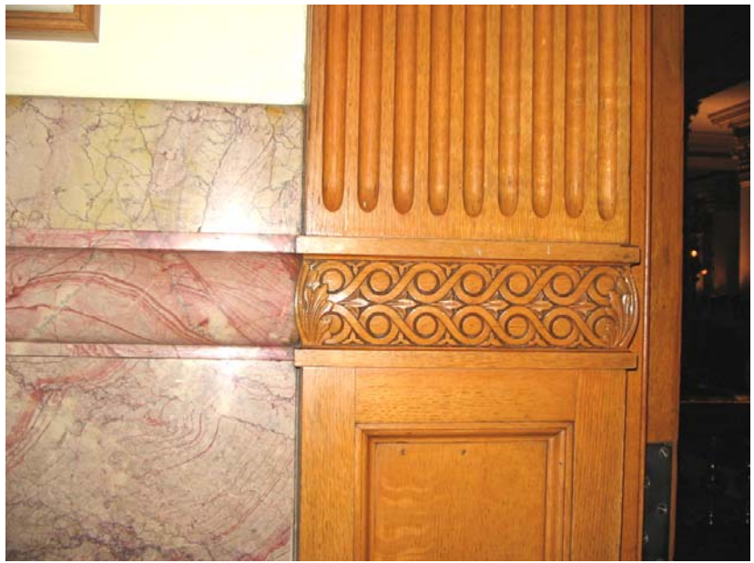
Finish detail at Senate Chamber Vestibule
