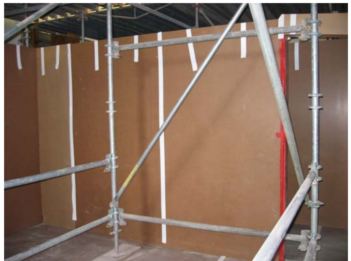
119 South wall protected during construction for the Life Safety Project
