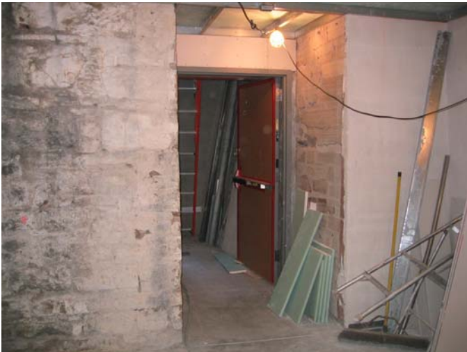
Door to new exterior Northwest Stair at Sub-Basement
