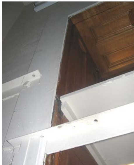
074 Remnants of original stair
