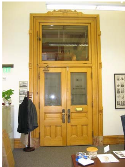
140 South wall entry doors from Arcade
