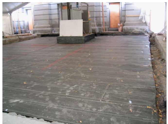
New tunnel lid under construction in 2005 as viewed from street level
