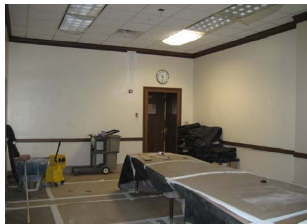
0111 View of south wall
