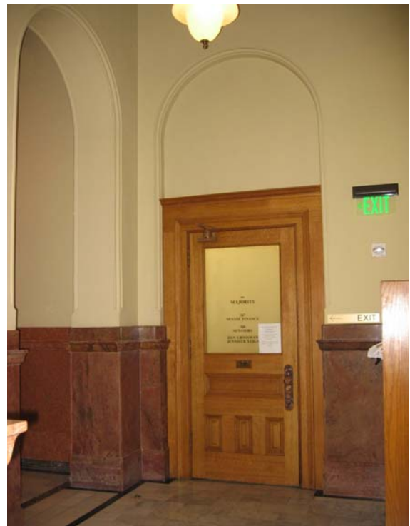
344A Northwest corner to Room 346
