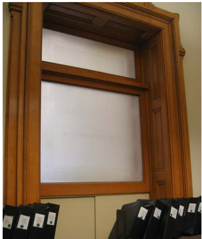
089 Original internal window south wall
