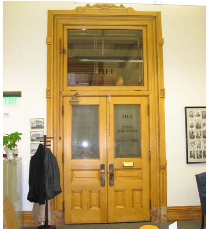
Type D1 doors with transom frame style
