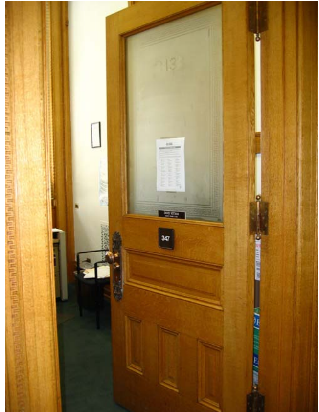
347 Entry door from Room 346
