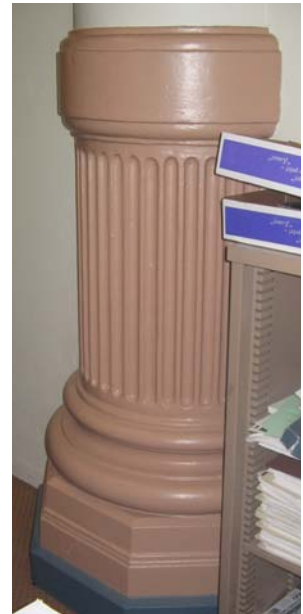
048 Cast iron column base
