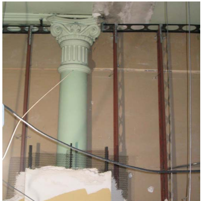
351 Original cast iron column.
