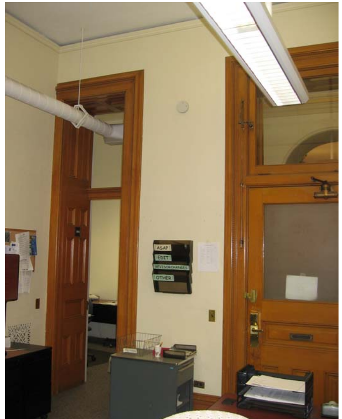
0100 View of west wall
