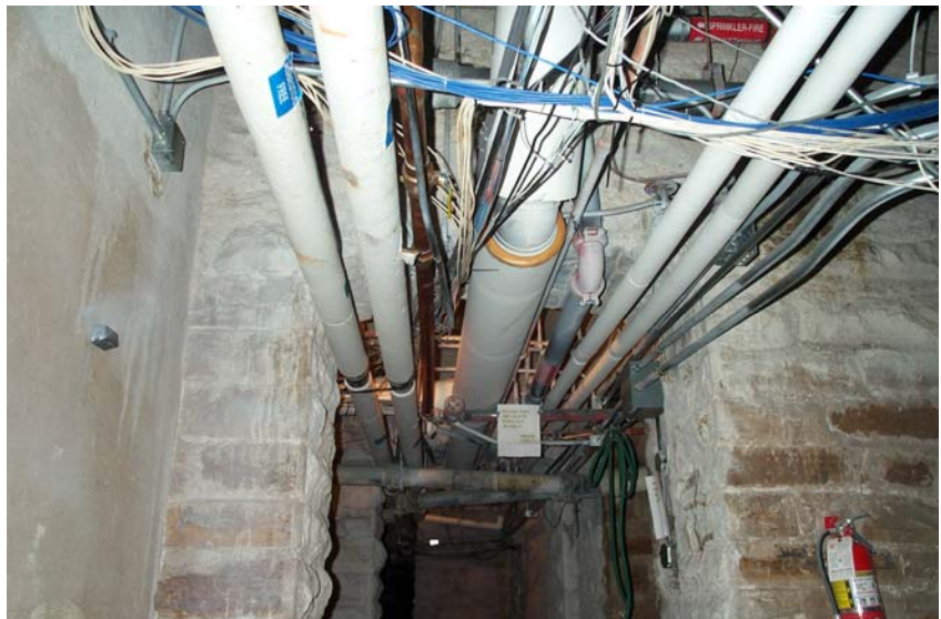
Mechanical and electrical systems being run overhead in the Sub-Basement
