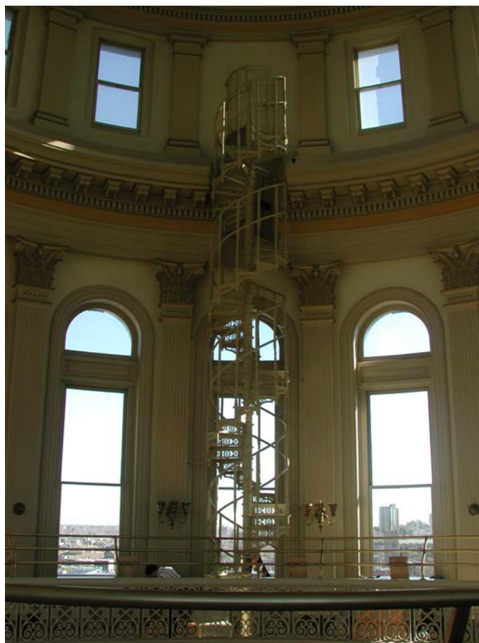
Dome: ornamental spiral staircase leading to the Upper Dome
