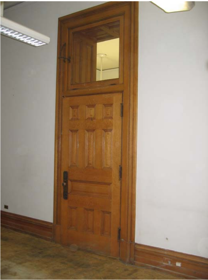
006 East wall showing door leading into room 004
