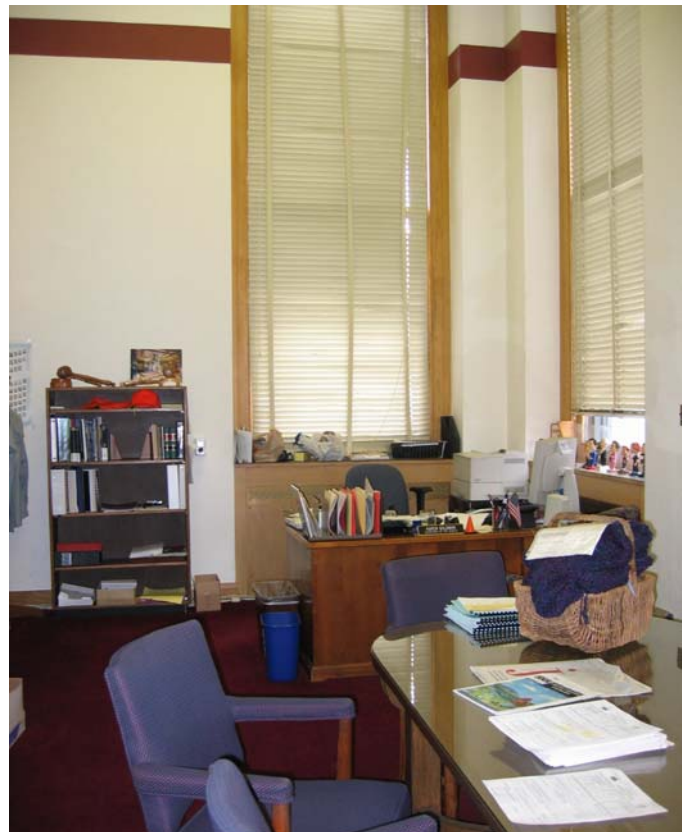
250 Windows in southwest corner with original trim removed
