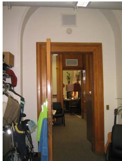
092 In-filled arch looking to 090
