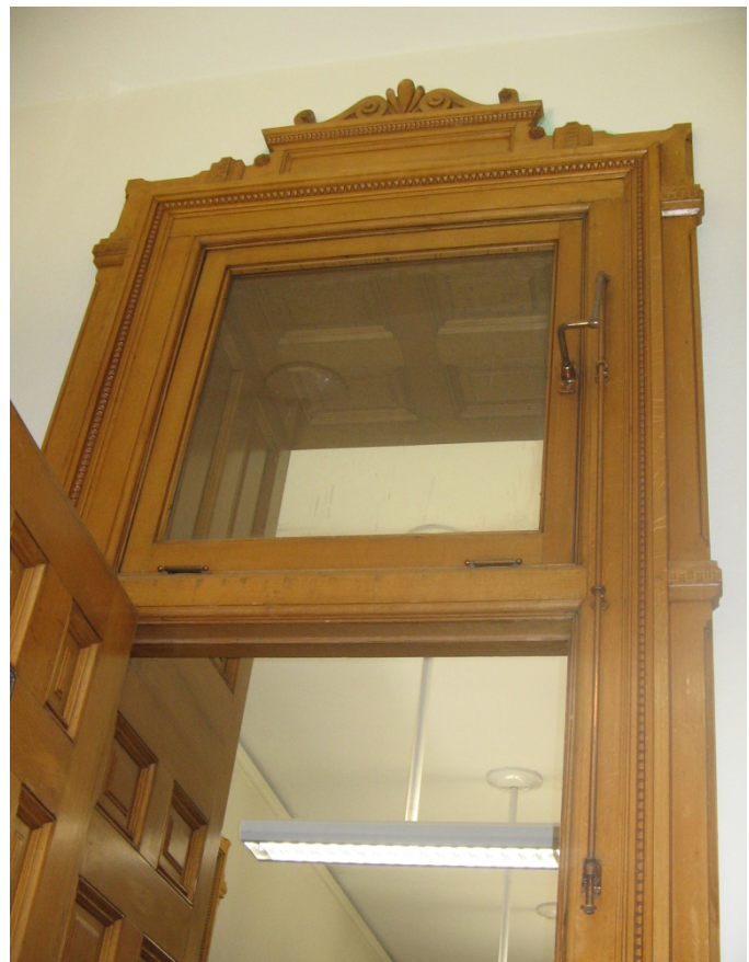
0105 Original door with transom
