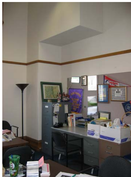
316 Mechanical chase, northeast corner
