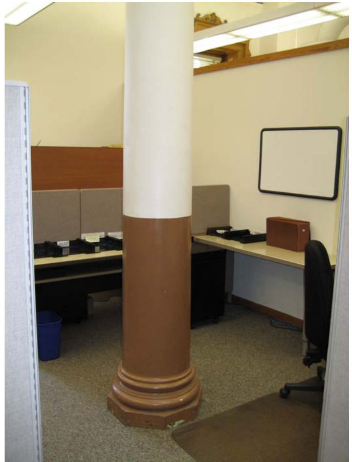
081 Cast iron column
