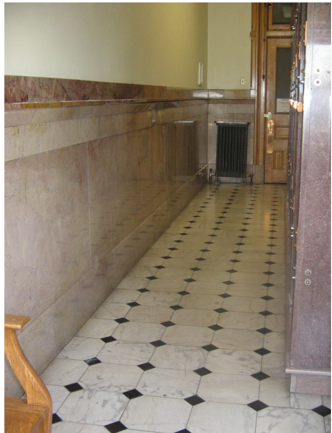
319 Original restroom finishes with radiator on east wall
