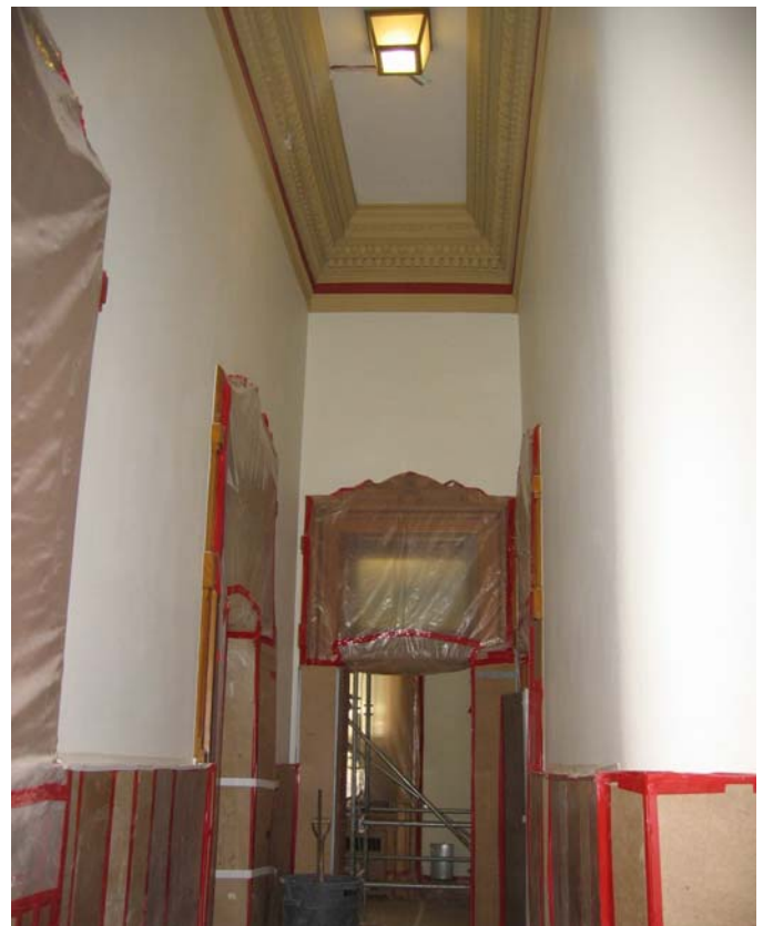
100A Looking east to room 104
