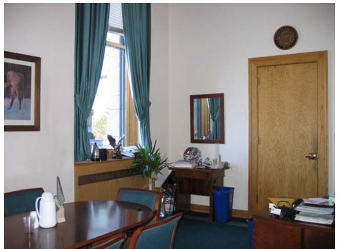
244 Non-original radiator housing and slab door on the north wall
