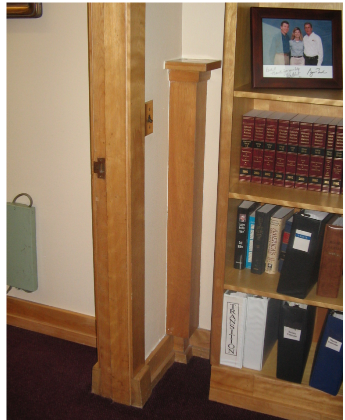
162B Wood detail at door to Room 162
