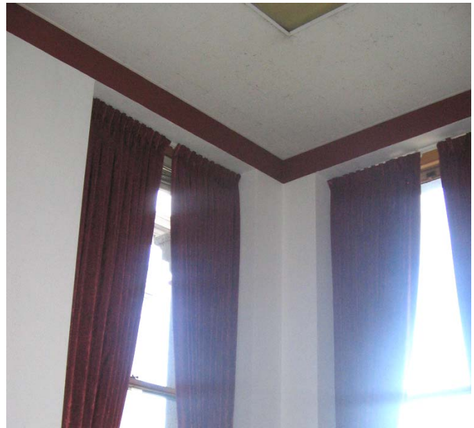
259 Original wood window trim has been removed
