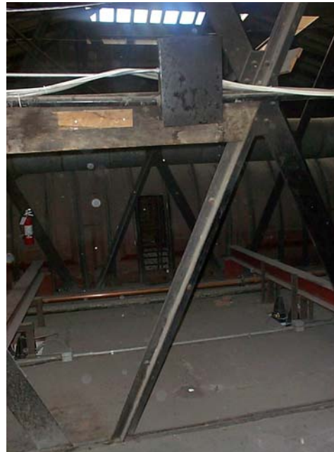
Built-up iron trusses
