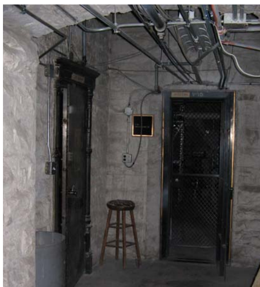
Original Vault doors
