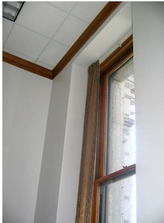
132 Plaster return and non-original window frame detail
