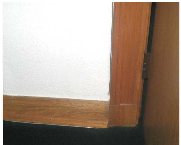
247 Non-original wood trim and base detail
