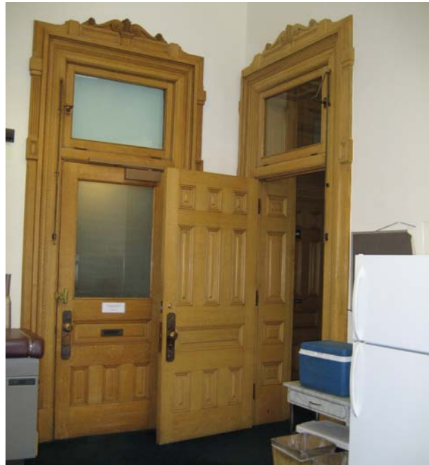
229 Southeast corner and doors to stairwell 228 and hallway 231
