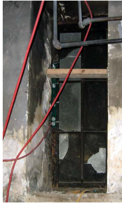
Sub-Basement exterior window
