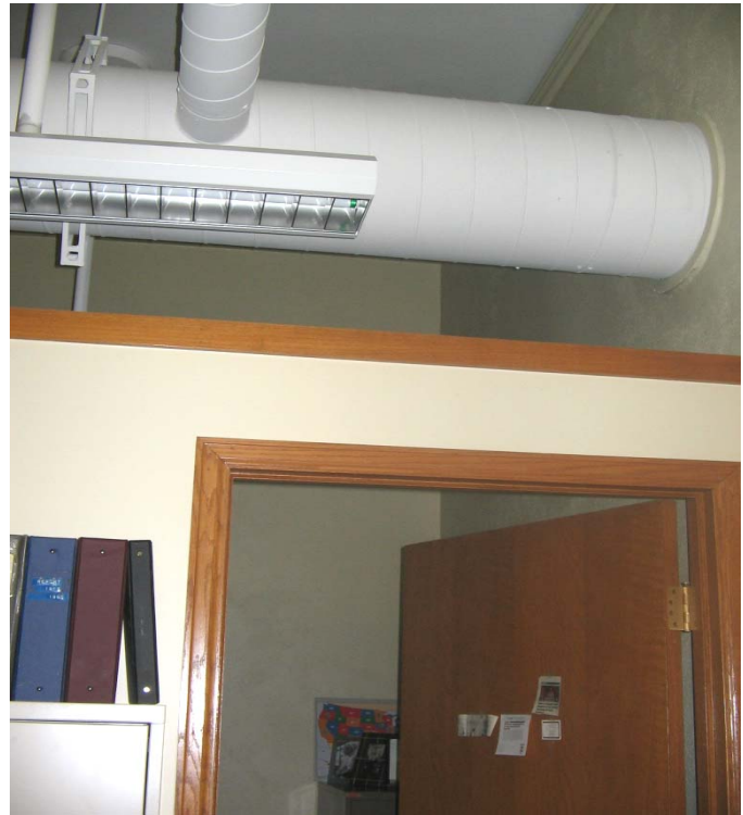
096 Partial height walls and exposed ductwork
