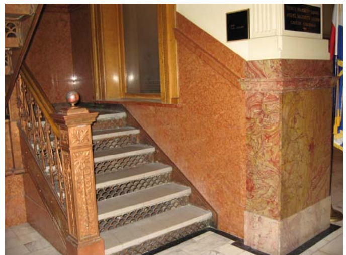
Southeast Stair Second Floor landing
