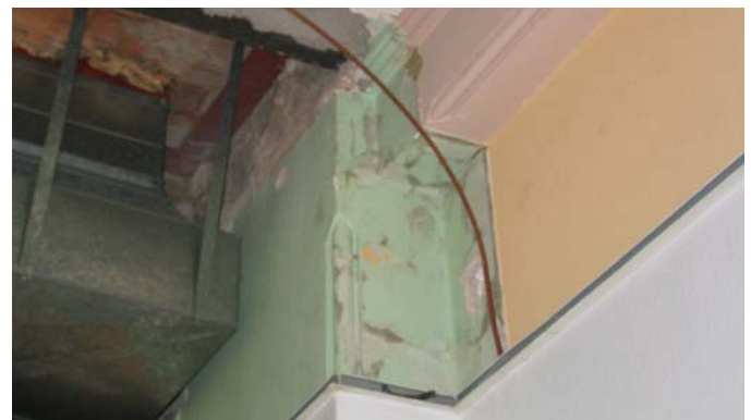
027 Patched-in opening above ceiling in southeast corner
