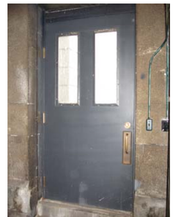
0116 Exterior door from inside
