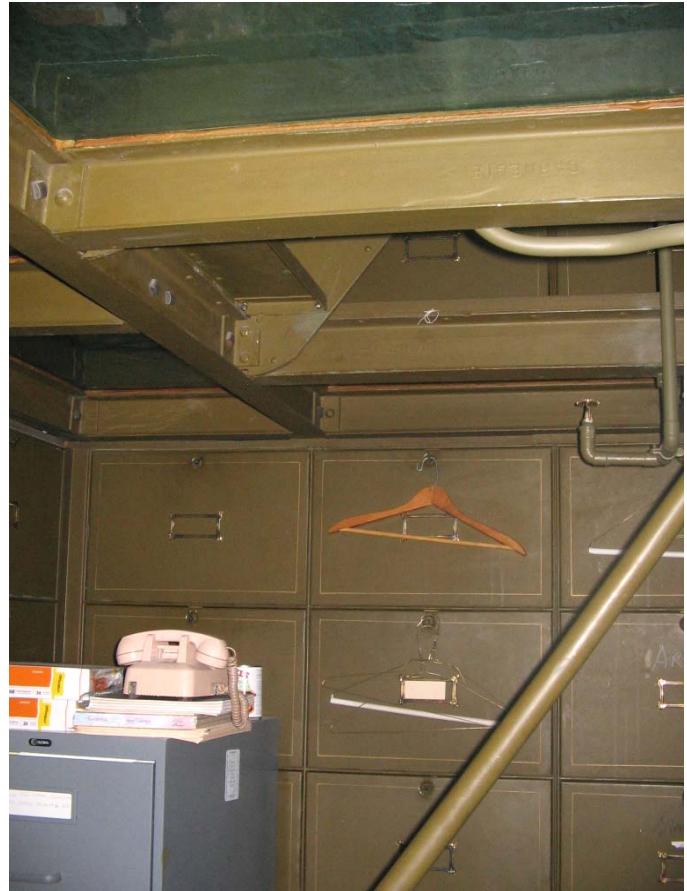
224 Original vault storage with glass flooring above
