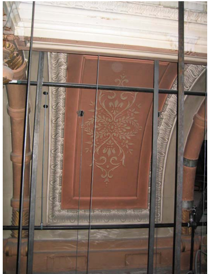
Hand painted pressed tin skylight above Senate Chamber; no longer visible
