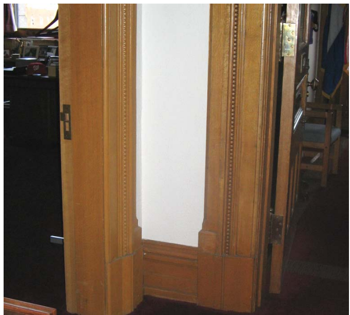
257 Detail of existing trim at doors to Room 258 and Room 259
