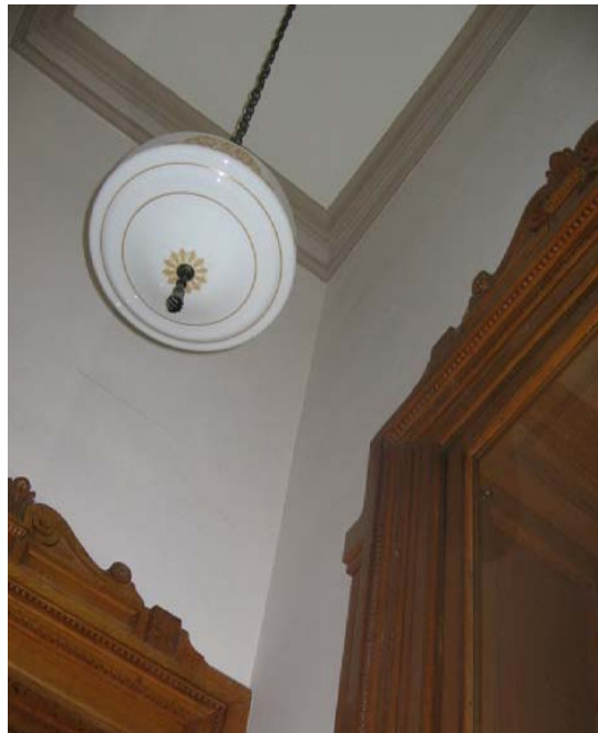
212 Lighting and trim detail
