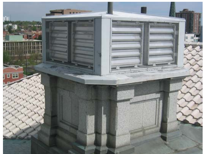
Current condition of boiler chimney
