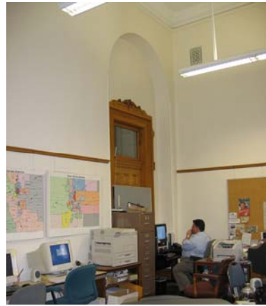
222 Wood trim and plinth
