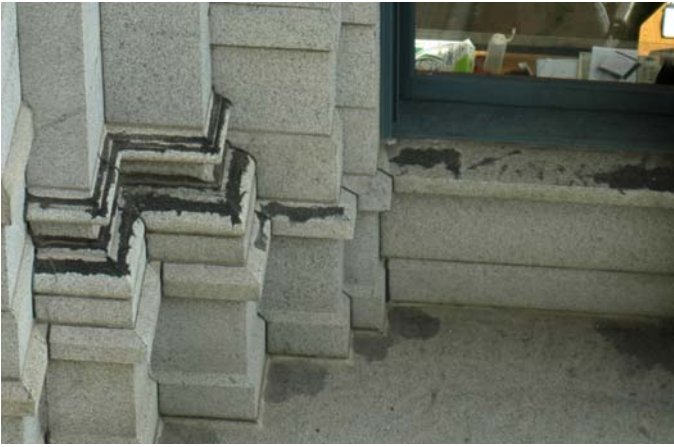
Dark colored roofing sealer
