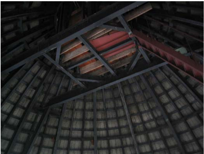
Upper Dome structure
