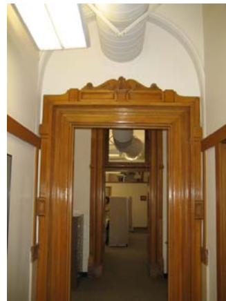
079 End of hallway looking west
