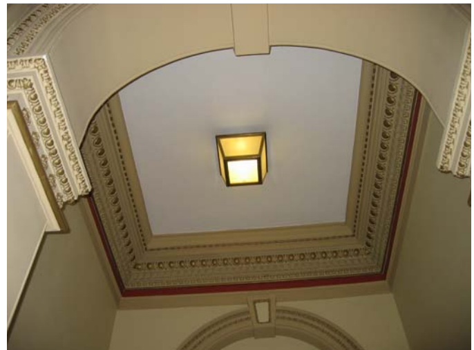
129A Light fixture and original decorative, painted cornice detail
