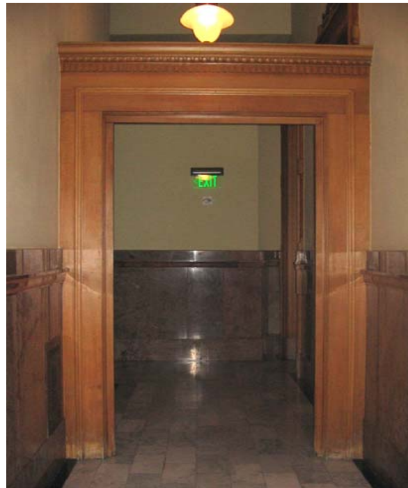
303 Non-original cased opening looking west
