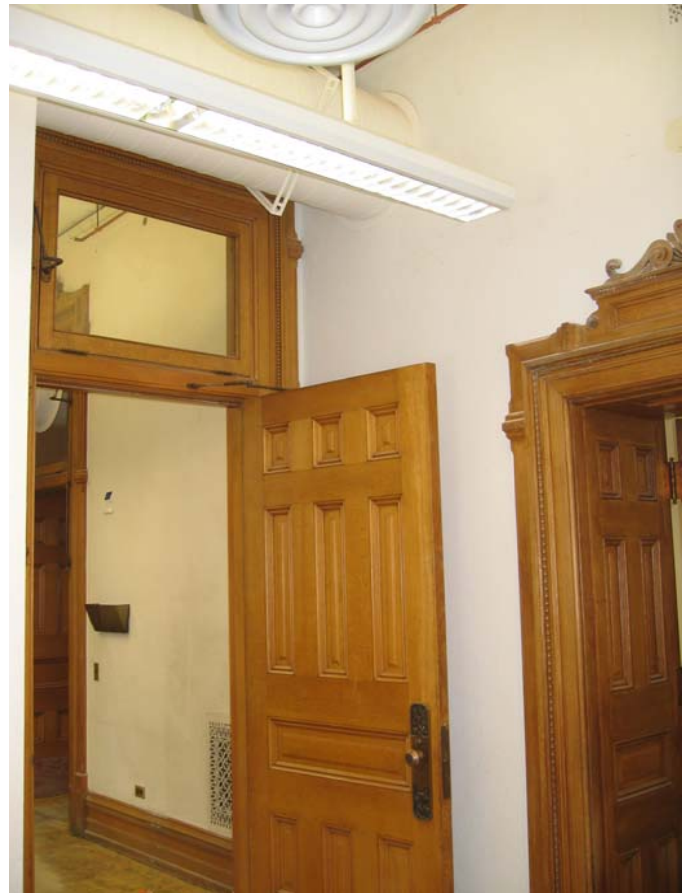
001 View of SW corner
