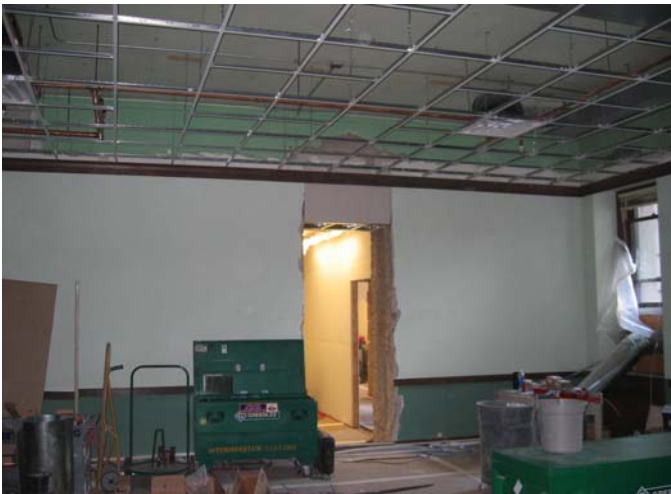
011 North wall showing newly reopened original opening
