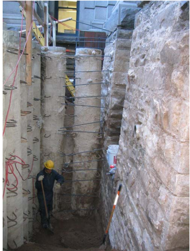
Excavation at northwest foundation wall for new exit stair
