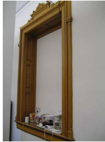
Original interior window, now within office space
