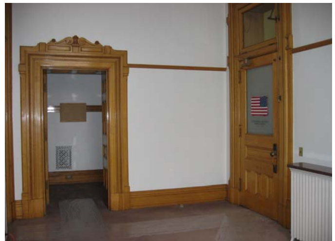
201 Northwest corner looking at Room 204 and door to corridor
