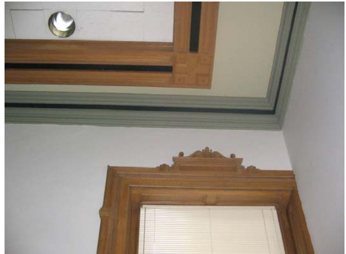
272 Cornice and wood trim detail
