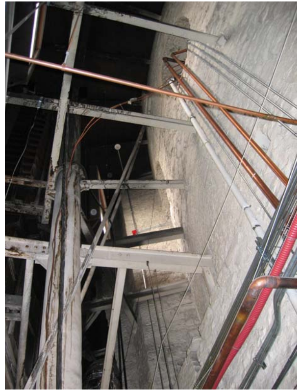
Dome Interstitial: Dome superstructure
