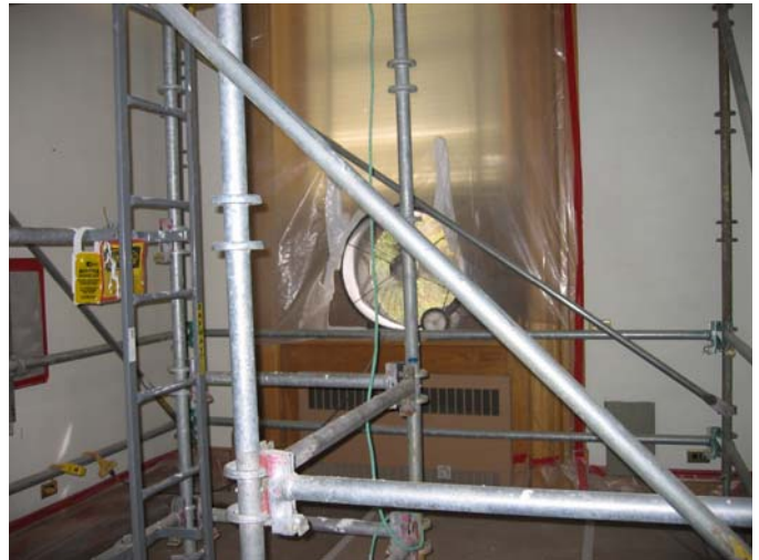
104 East window protected during construction of the Life Safety Project
