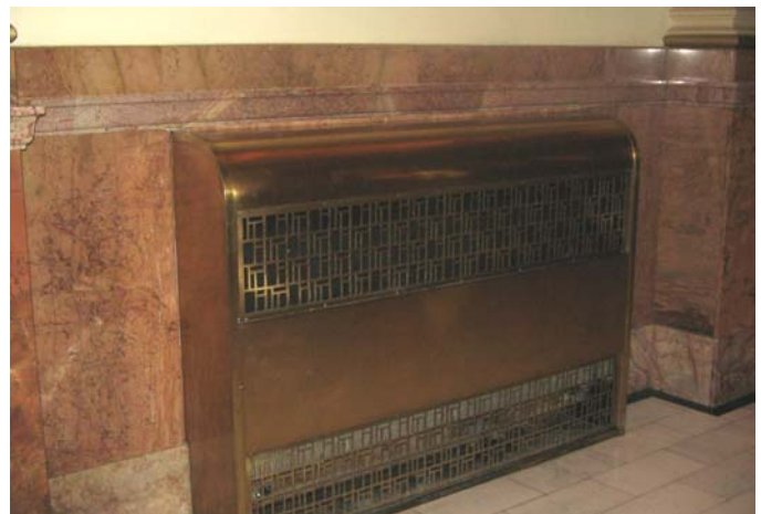
First Floor marble wainscot and radiator detail
