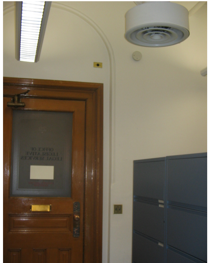
065 Archway in-fill with relocated door
