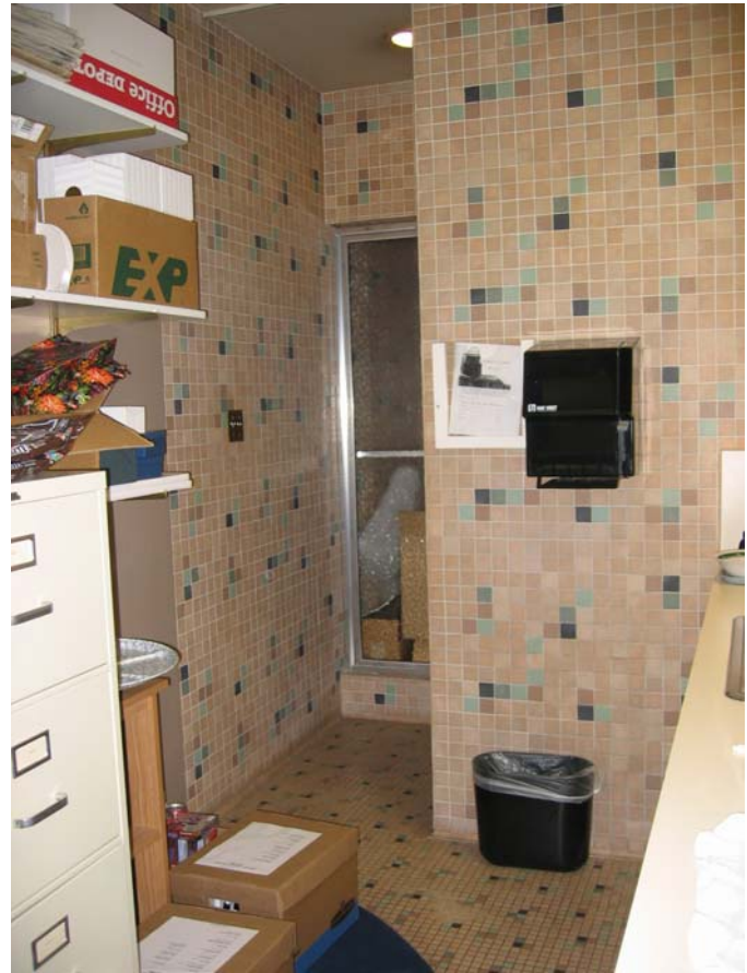
136D Tile walls
