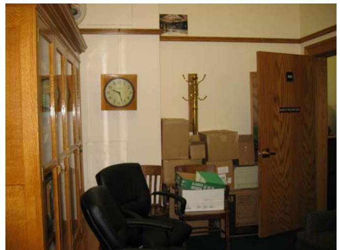
242 Picture rail and standpipe chase on the south wall
