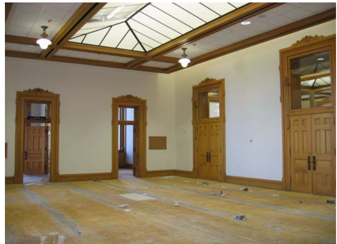
274 Southeast corner with faux skylight
