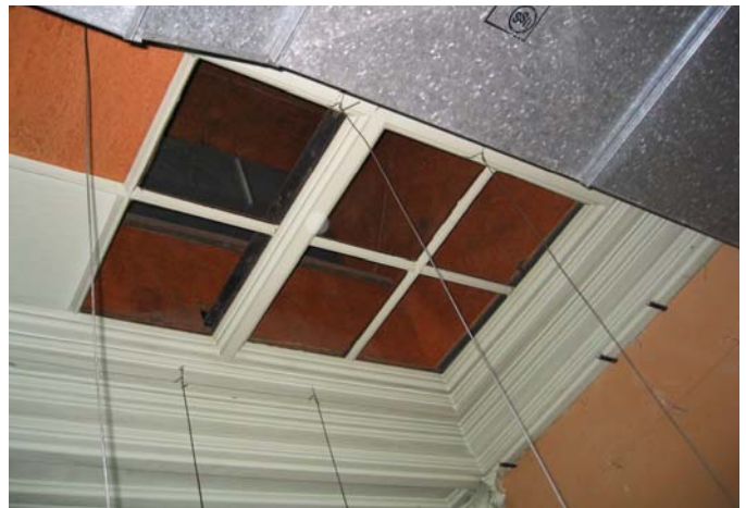
351 Original skylight above suspended ceiling.
