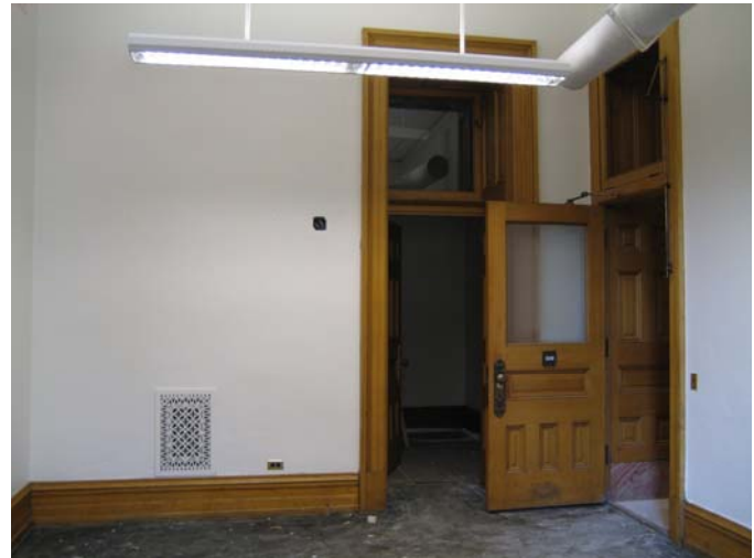
009 north west corner
