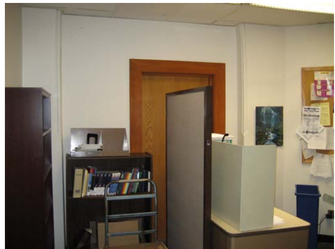
054 Existing north wall
