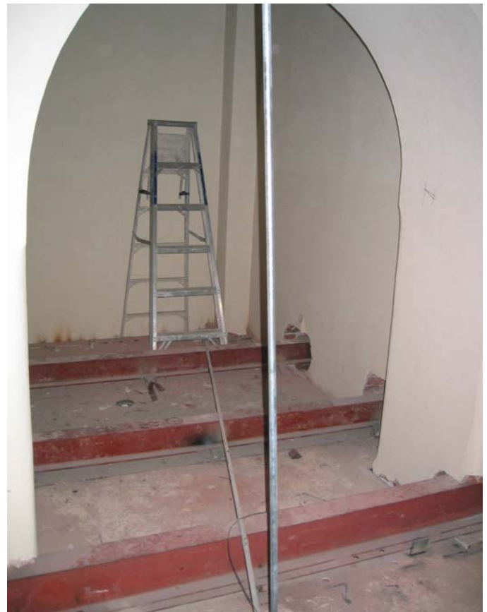
145A Space above the vault.
