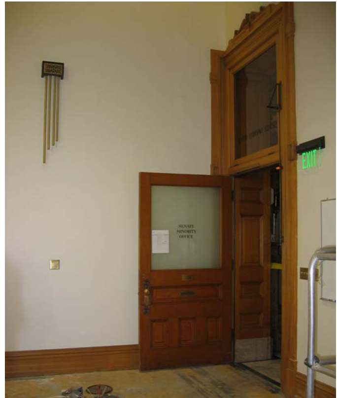
274 South wall at entry from Arcade
