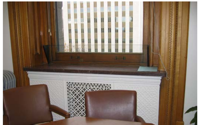
221 original cast iron radiator front at north window
