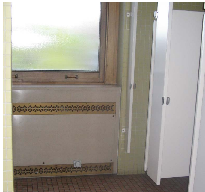
262 Window modifications and non-original metal partitions
