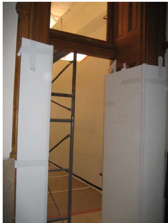
017 View of entry door from hallway 007
