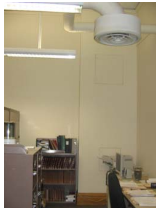
0102 Standpipe chase in southwest corner
