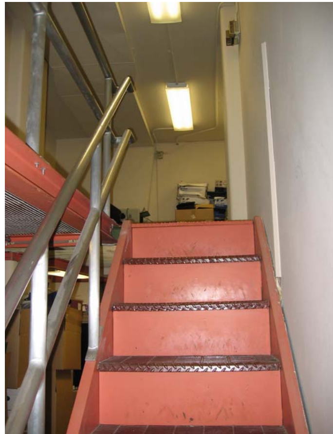
128 Stair to vault floor above
