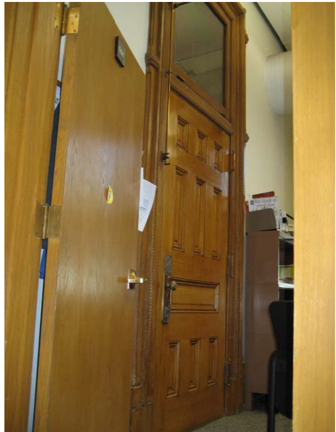
064 View looking in at south wall
