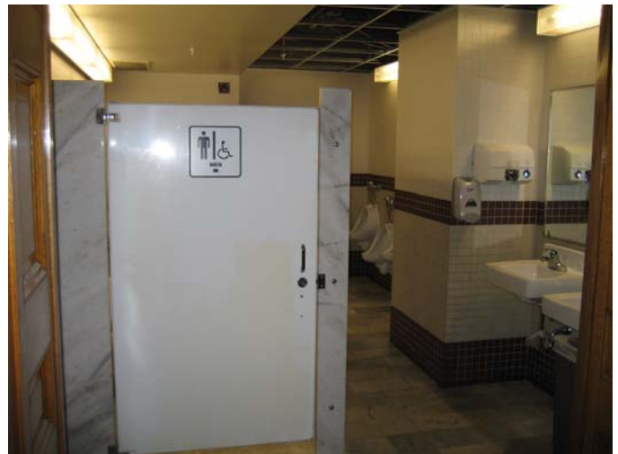
020 Existing conditions looking south from entry
