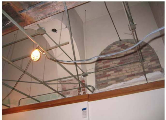
130 In-filled opening at south wall, part of a former vault.
