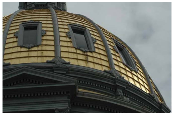
Dome painted steel exterior windows
