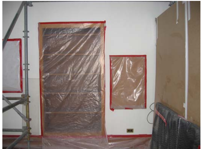
106 Bookcase on south wall infilling opening
