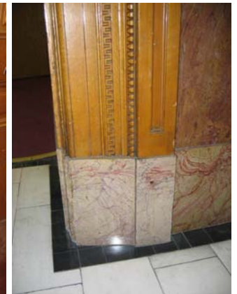
Stone plinth base
