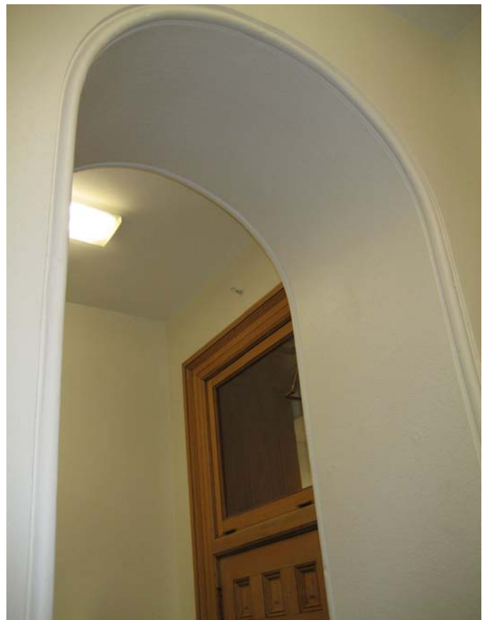
030 Arched opening on south wall looking into 031A
