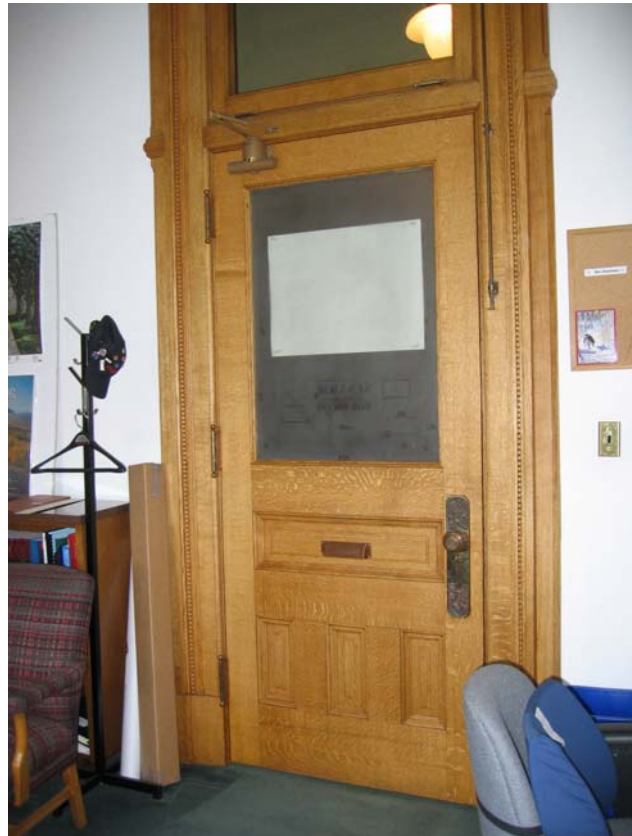
342 Door from corridor
