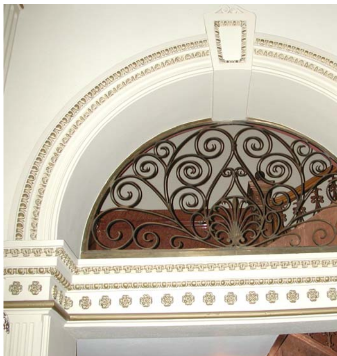
Pilaster, arch and cornice detail
