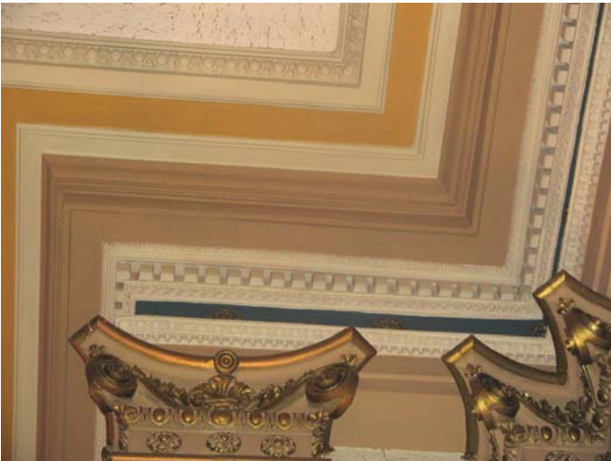
Senate Chamber plaster cornice
