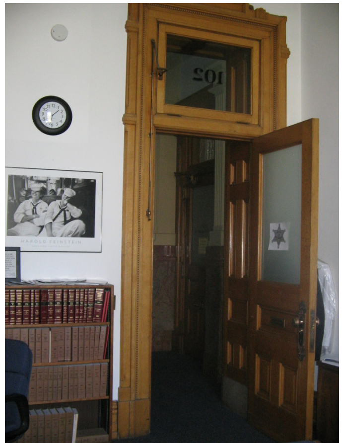
102 Entry door to Room 100B
