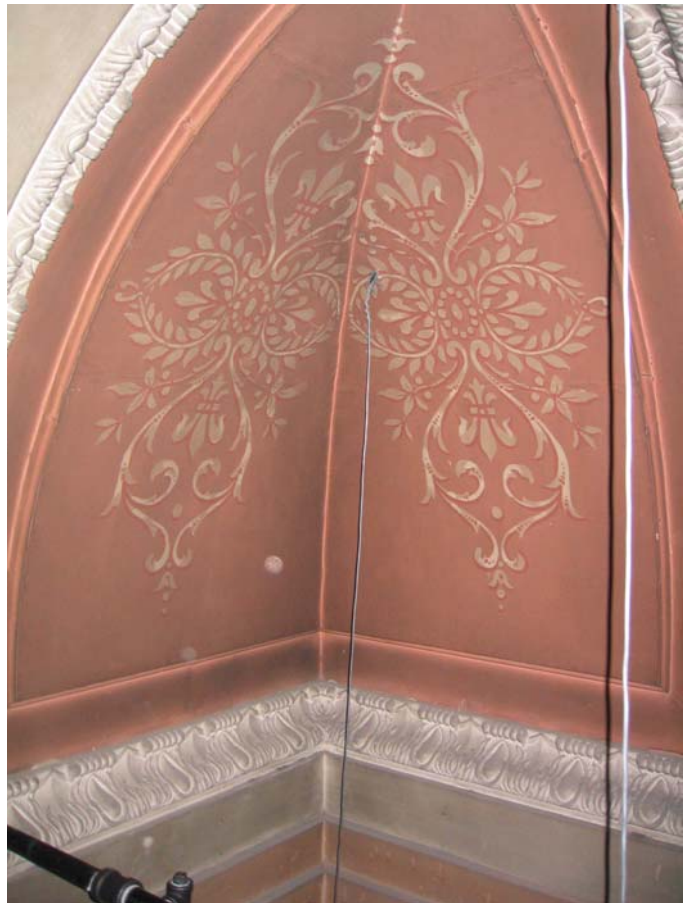
Attic: Senate Chamber interior skylight, hand painted pressed tin panels
