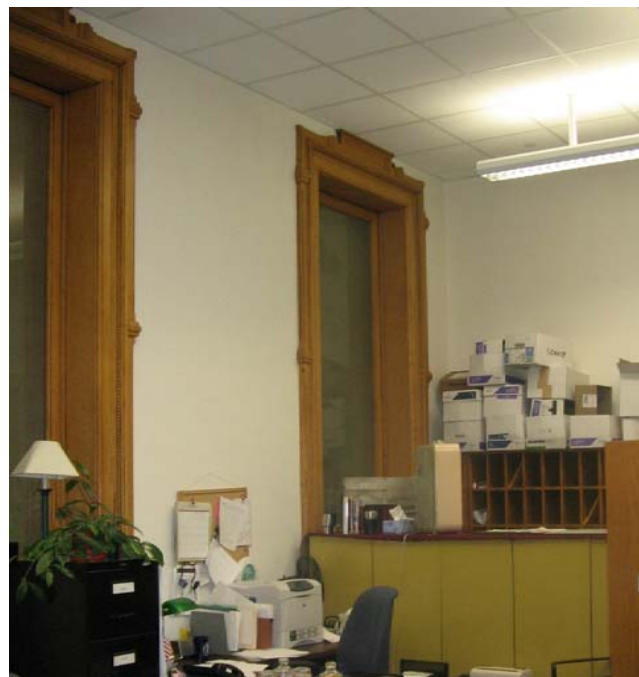
346 View of west wall
