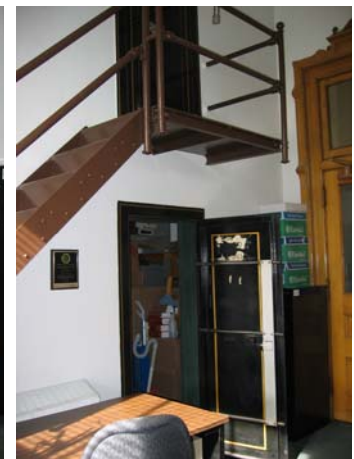
336 View of stairs to second level from Room 337
