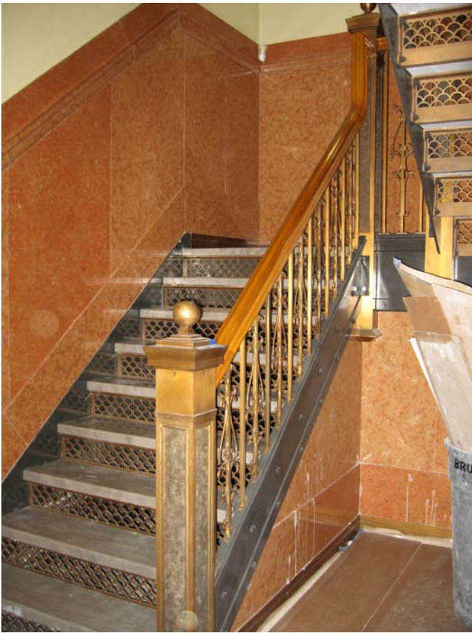
Northeast Stair First Floor during construction 2006
