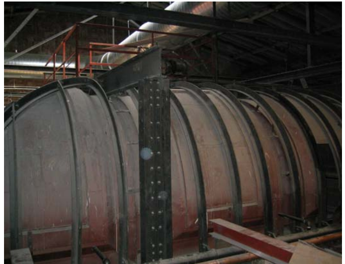
Attic: Senate Chamber interior skylight
