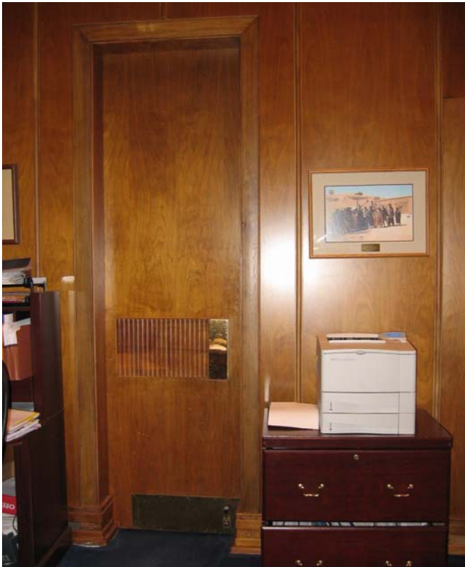
East wall at door to Room 136D
