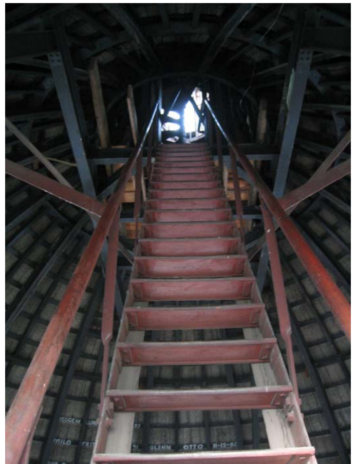
Upper Dome: Ladder to Cupola
