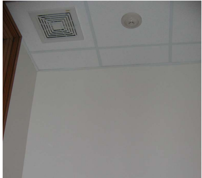
138 Existing ceiling conditions
