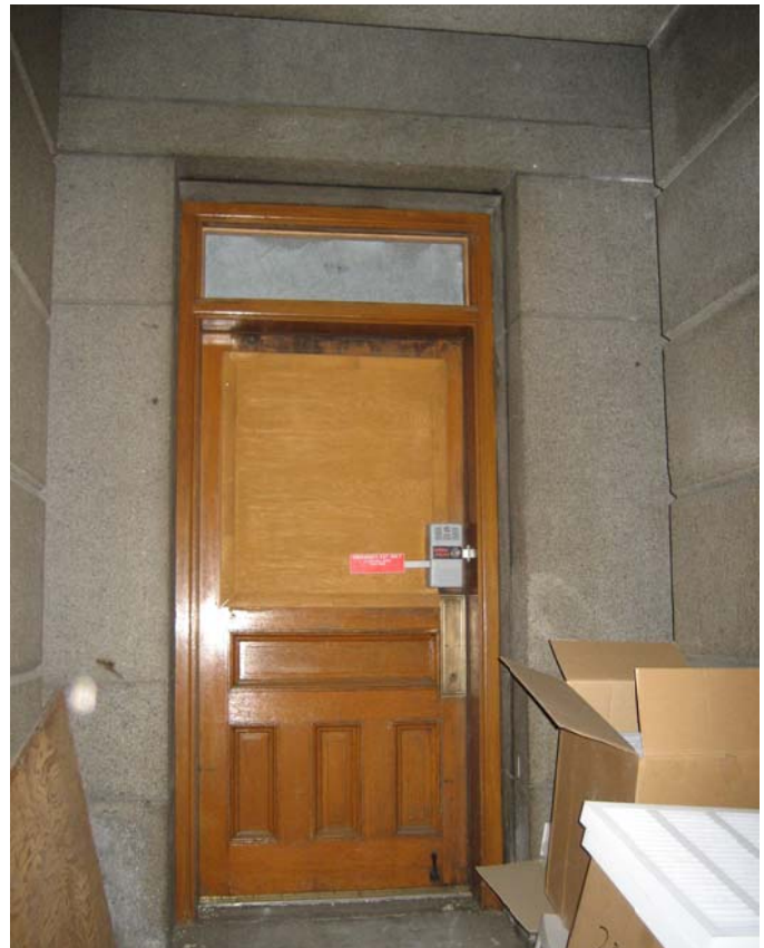
051 South wall with exit door
