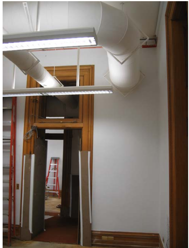
004 Entry door on south wall
