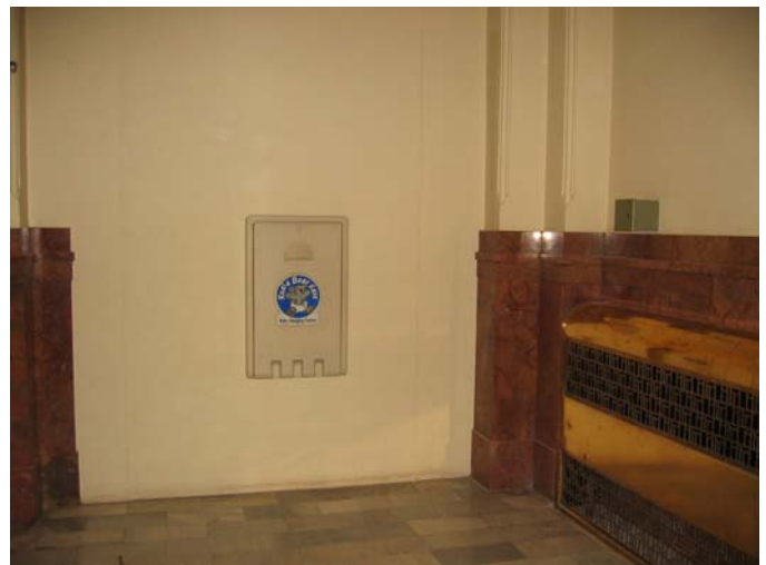
020 Vestibule area looking north
