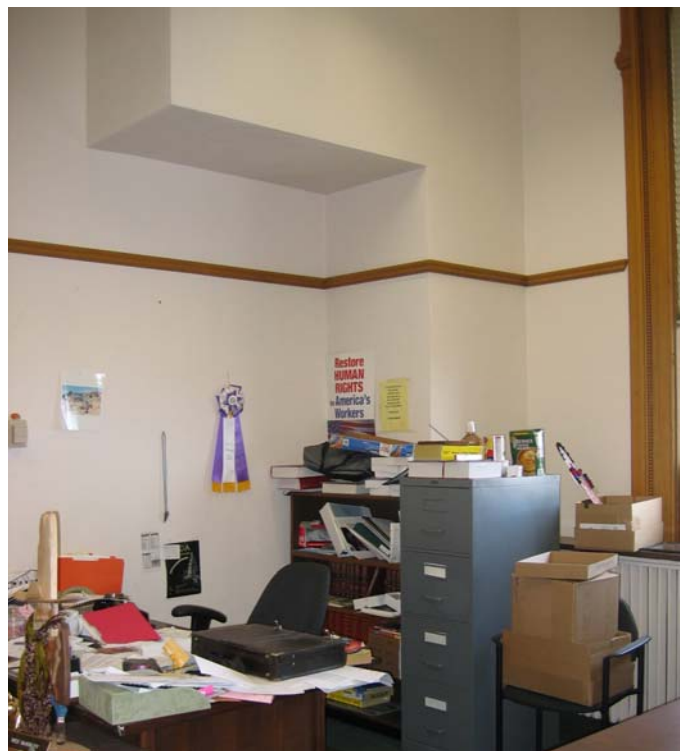
314 Mechanical Chase in northwest Corner
