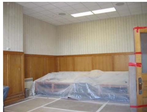
326 East wall with platform fixed seating
