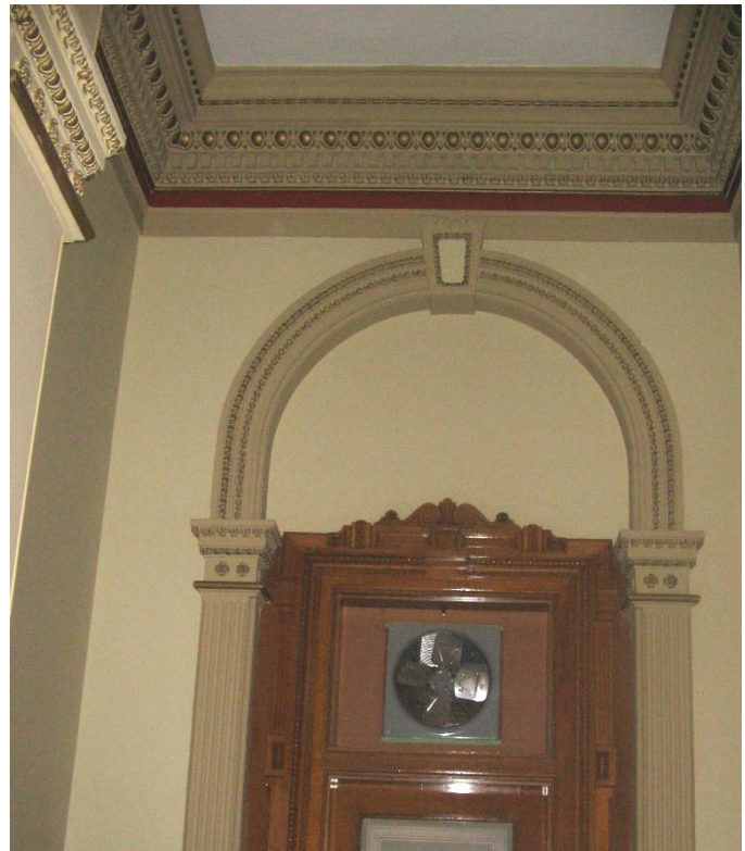
129A In-filled arched opening with relocated door
