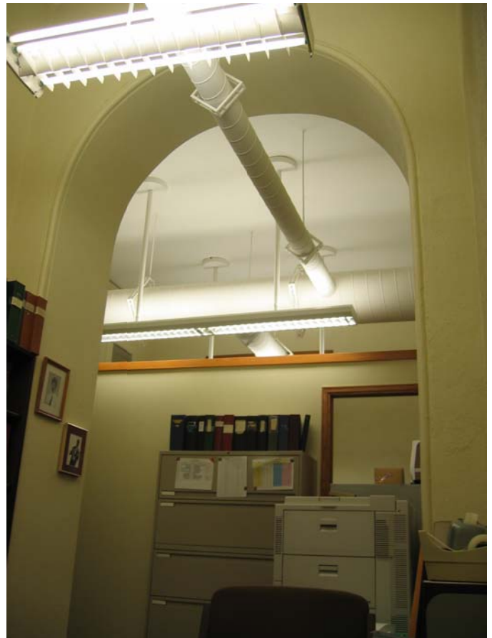
097 Looking east; original corded archway
