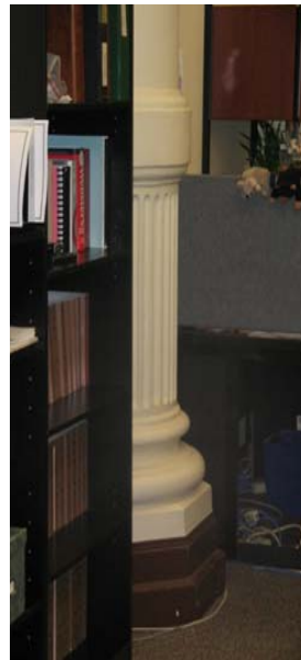
091 Cast iron column of former public corridor
