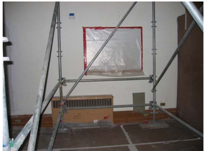
115B Non-original radiator at south wall
