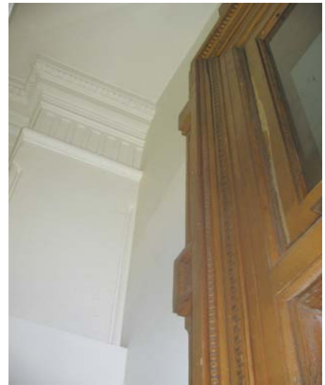
078 original plaster cornice
