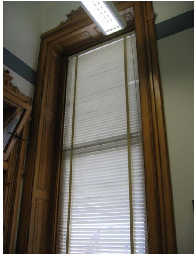
127B Window on south wall
