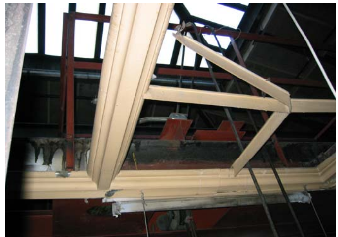
Existing coffer detail above non-original House Chamber ceiling
