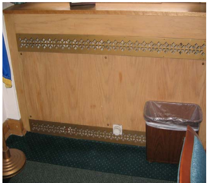
244 Non-original radiator housing detail
