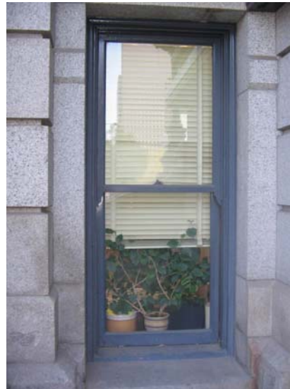
Basement exterior window
