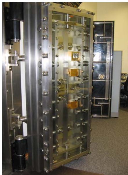
140B Non-original vault door
