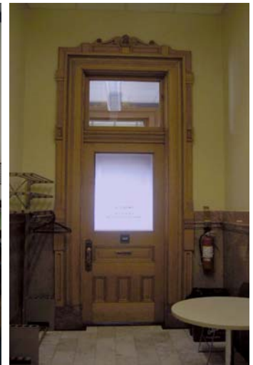
334 Door to Room 332 from Hallway 334
