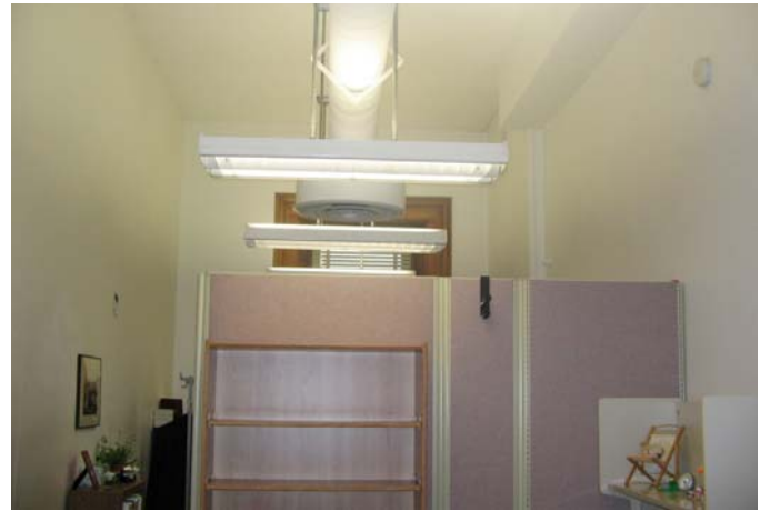
017 View looking north
