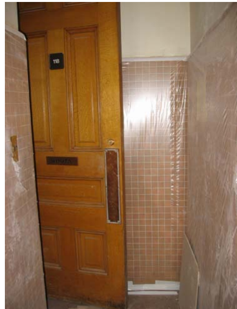
118 Entry door with push plate on corridor side
