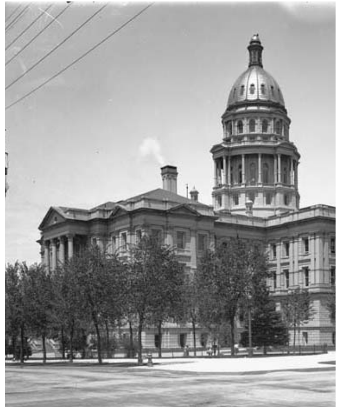
Historic Photo of Southeast corner showing the large Boiler Chimney and two smaller vents
