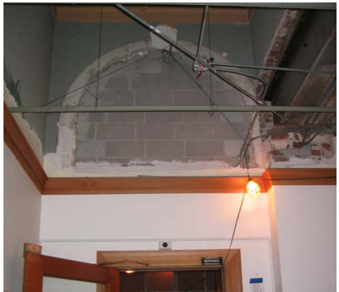
130 In-filled opening into First Floor Arcade.
