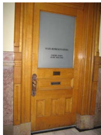
223 Entry from Arcade side
