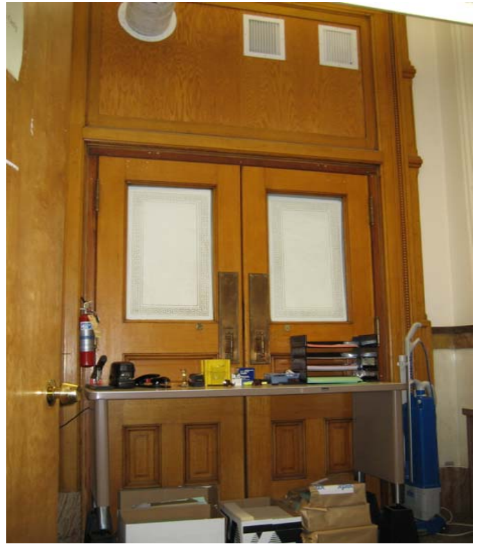
077 view at original vestibule doors
