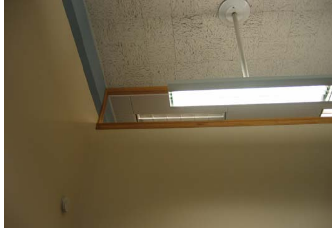
156 Clerestory window at non-original east wall
