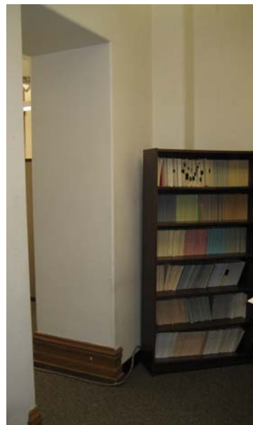
060 Opening at former vault door
