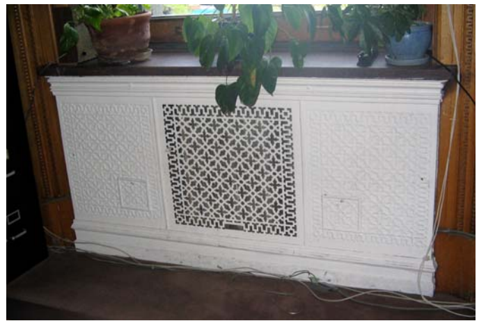
201 Original radiator housing with Cedar marble top
