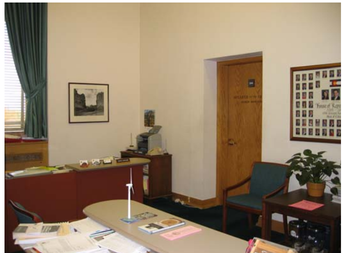
246 Non-original door and trim to Room 244
