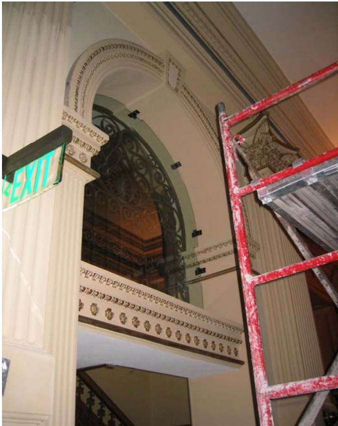
Glass installed above Second Floor Northwest Stair entry
