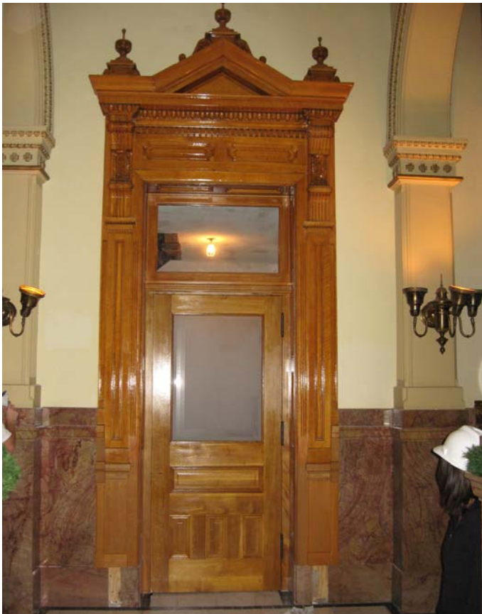
First Floor Northeast Stair after converting window opening into doorway
