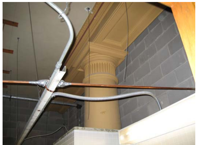
020 Original columns and cornice above the current restroom ceiling
