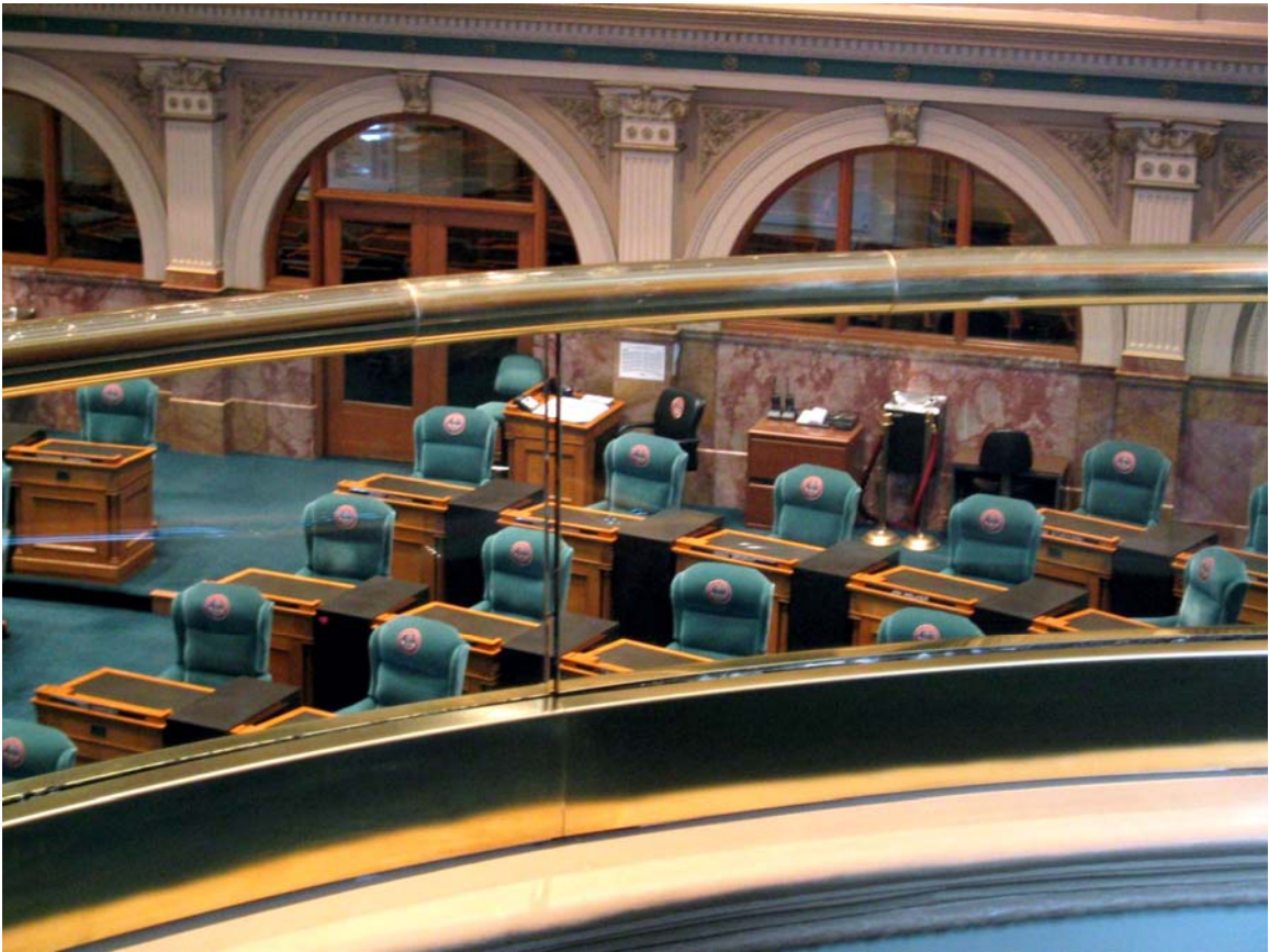
House Chamber view of entry from Gallery showing new brass and glass rail extension
