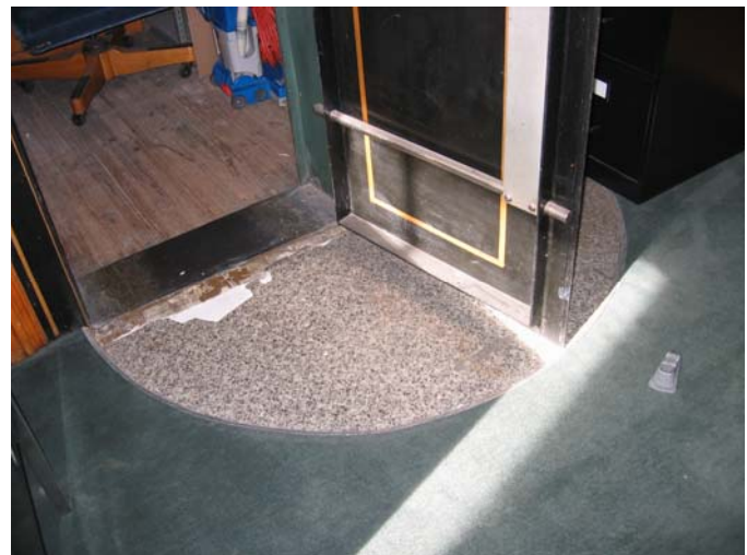
336 Vault door floor detail
