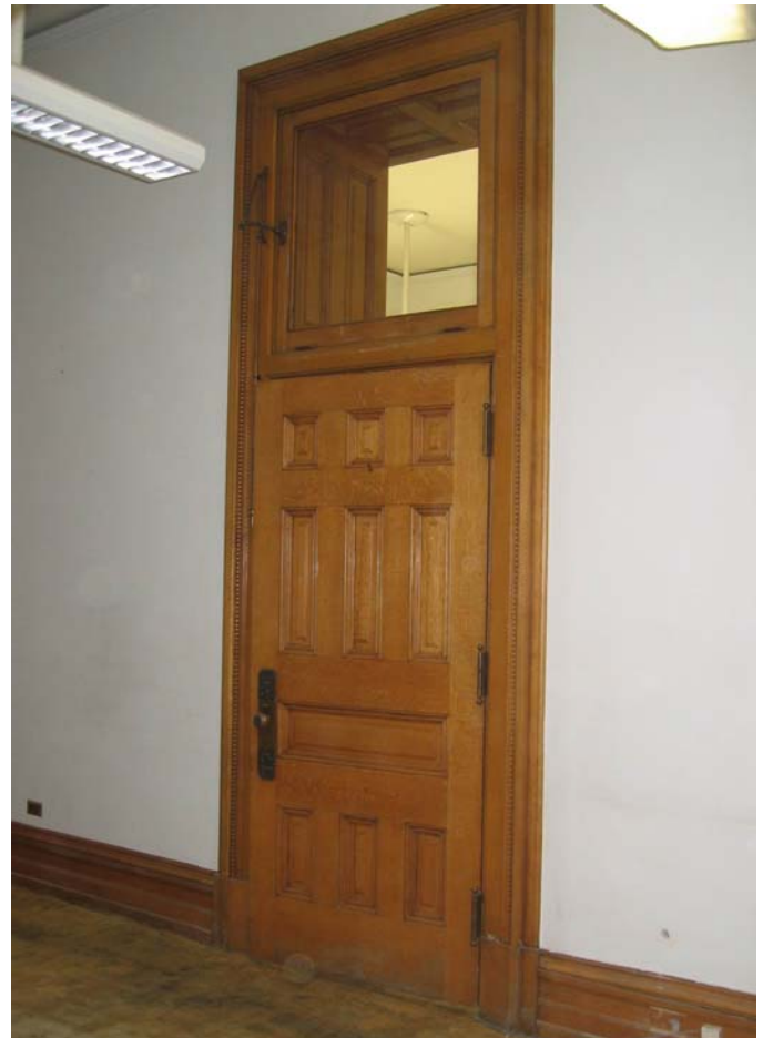
Type D2 door with transom frame style
