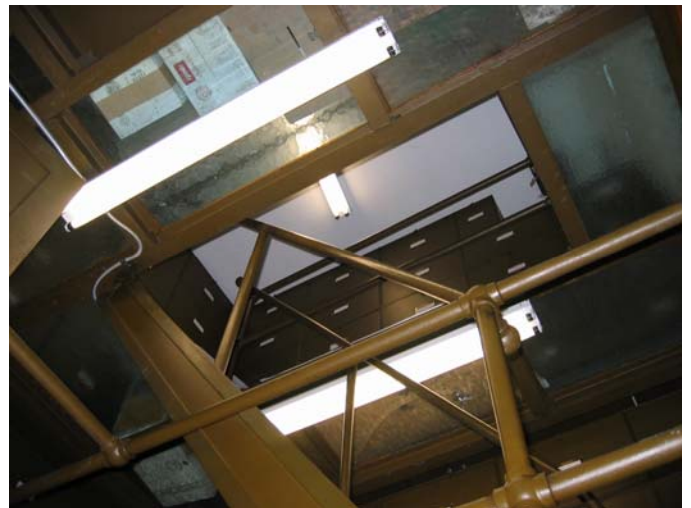
211 View up through internal stair
