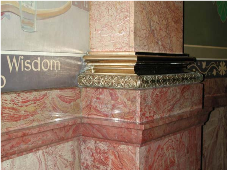
First Floor Rotunda detail of brass trim at pilasters
