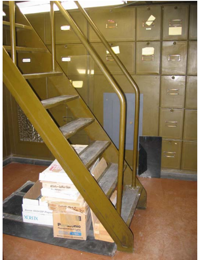
211 Bottom of internal stair
