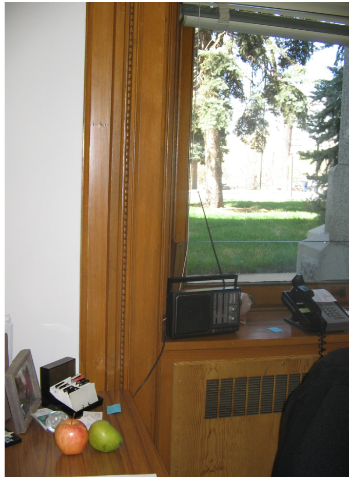
076A Exterior window detail
