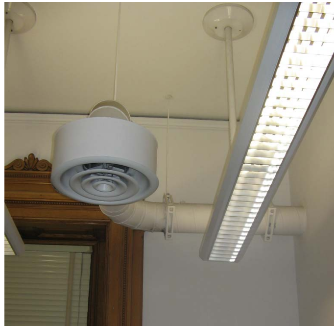
001 View of ceiling
