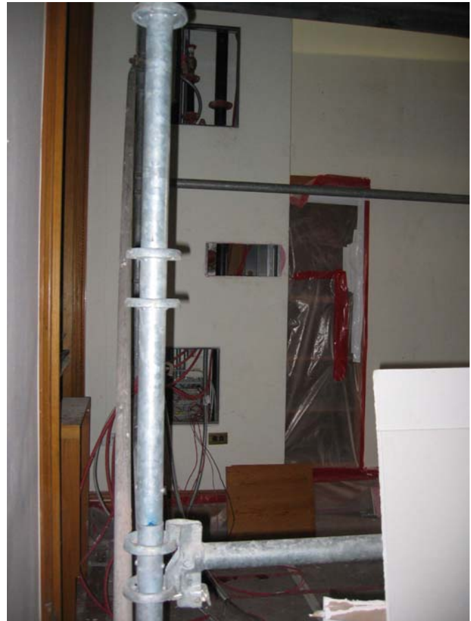
111 shaft in northwest corner
