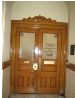
Relocated door in original west arch at Basement Rotunda
