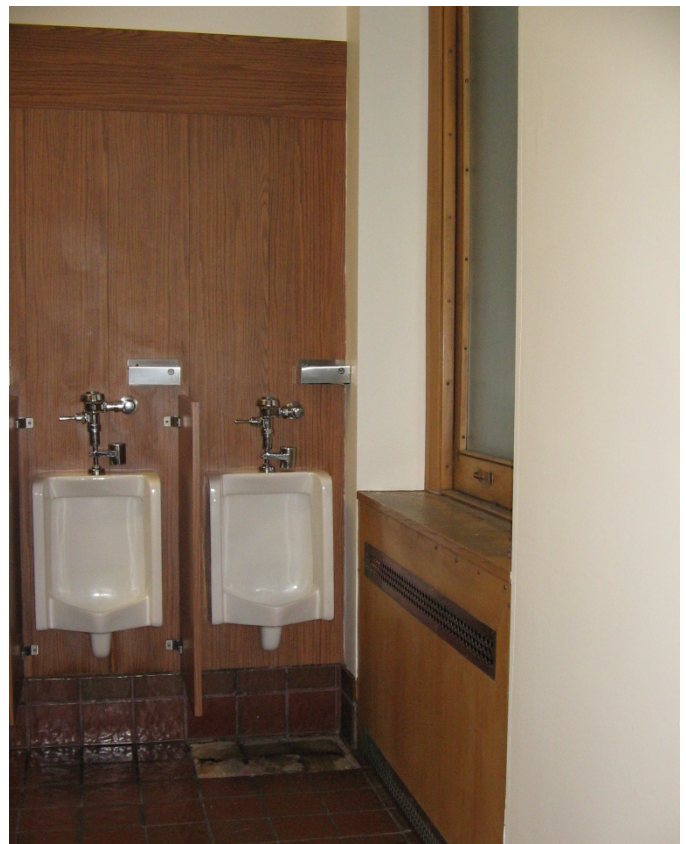
232 Plastic laminate wainscot on south wall
