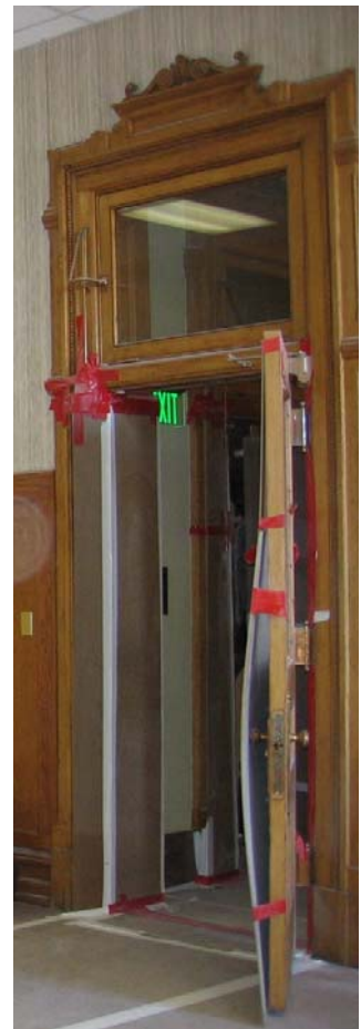
326 Entry door from corridor
