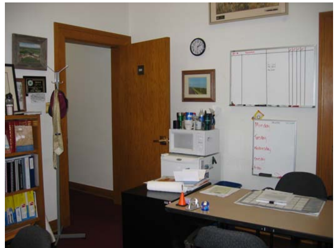
269 non-original slab door on the south wall
