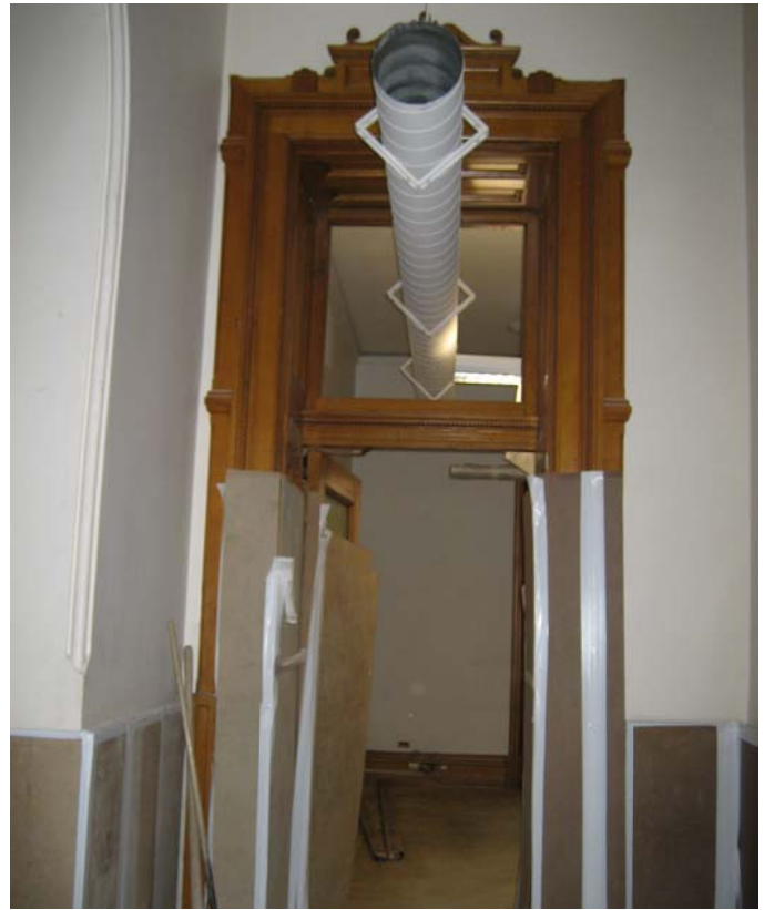
007 View of door into room 006 and a corded plaster arch
