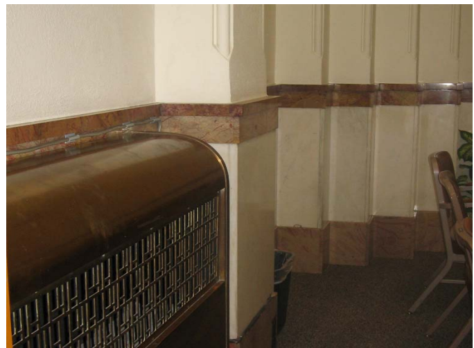
071 Stone wainscot and original brass radiator enclosure
