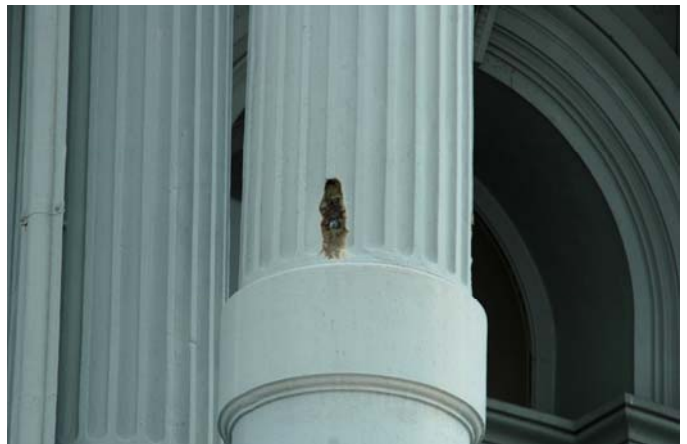
Rusting from within at column
