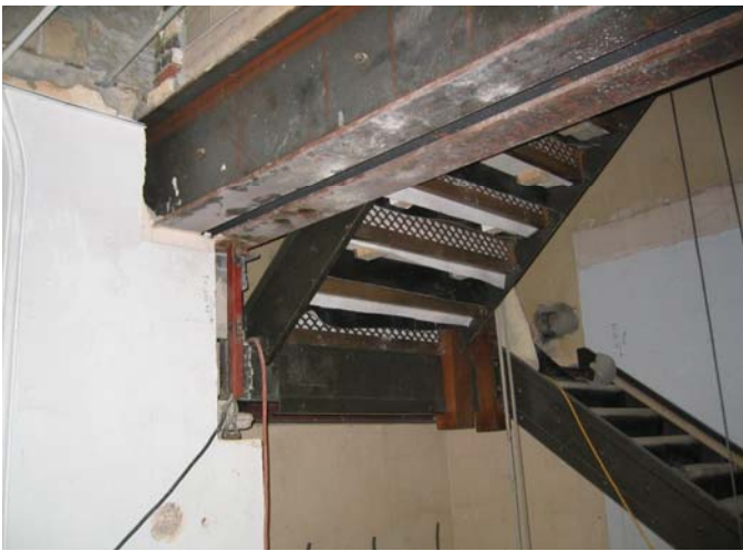
Basement Northwest Stair during construction
