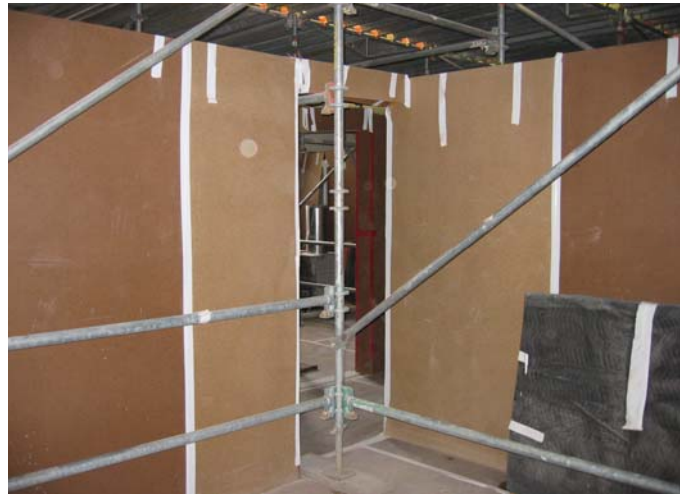
119 Southwest corner protected during construction for the Life Safety Project
