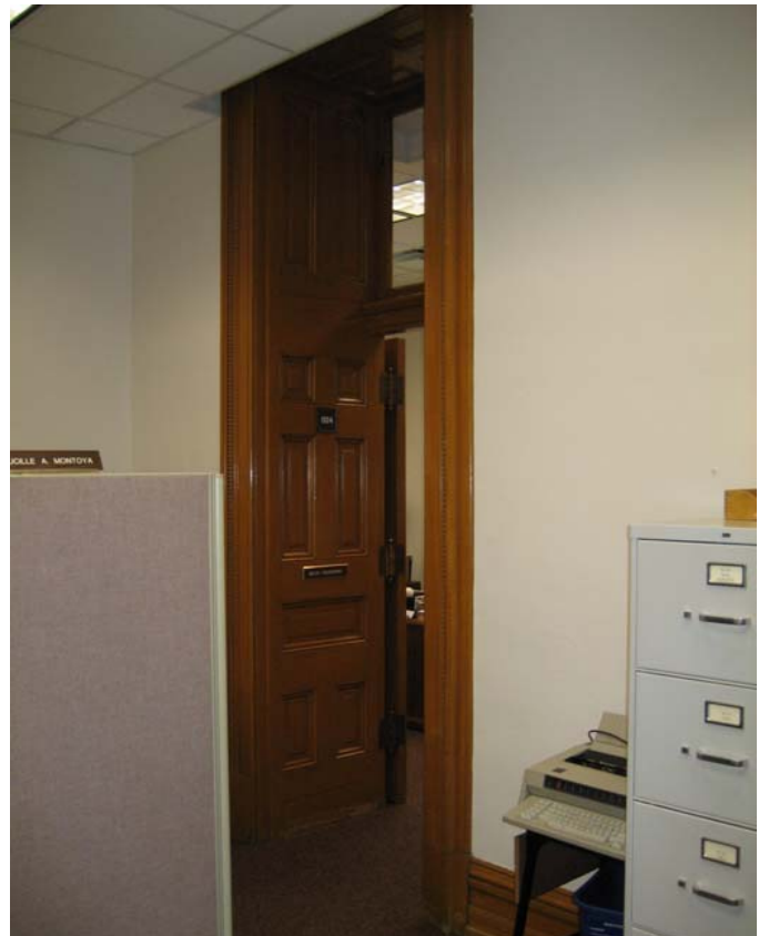
026 View of northeast corner
