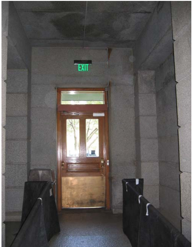
Basement North Entry Vestibule looking east
