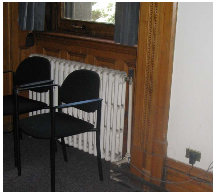
140 Existing original radiator at north wall
