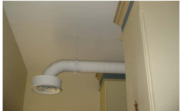
044 Ceiling showing original plaster cornice on original columns
