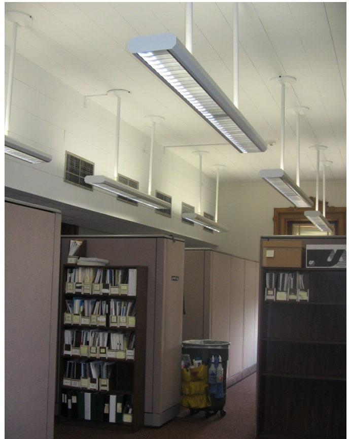
045 Added HVAC soffit to the left
