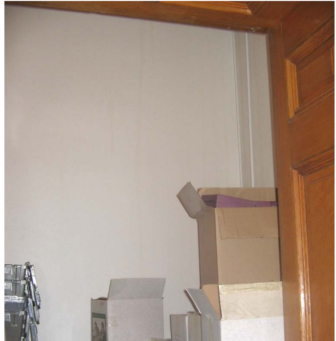
041 Looking through door
