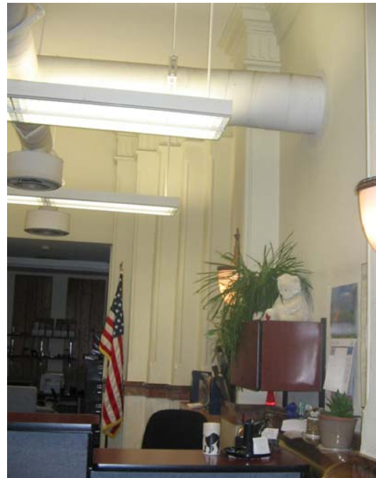
091 View looking north with corded plaster pilaster and stone wainscot of the former public corridor
