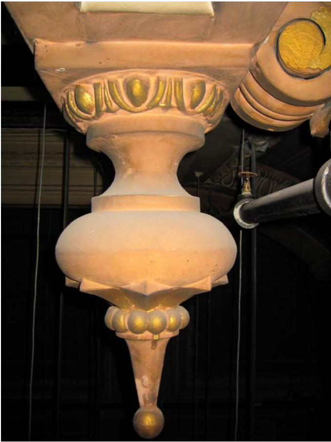
Attic: Senate Chambers Skylight, surviving drop pendant
