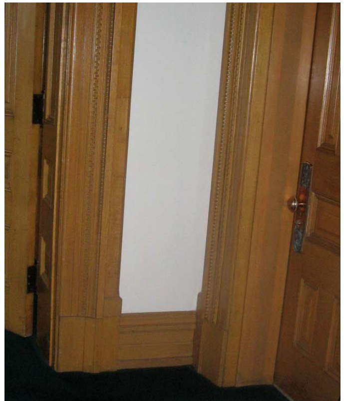
231 Door to Room 229 detail
