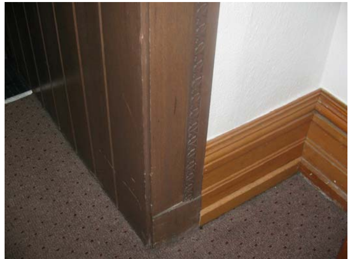
012 Non-original wood door frame and original 12” wood base
