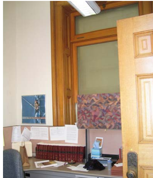
085A Interior window with original Greek key glazing
