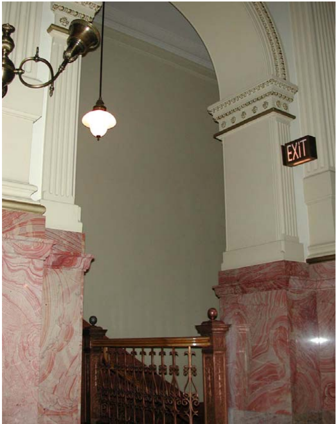
Third Floor prior to Life Safety Project improvements
