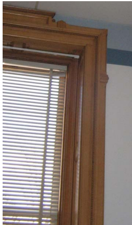
103 Window trim on north wall
