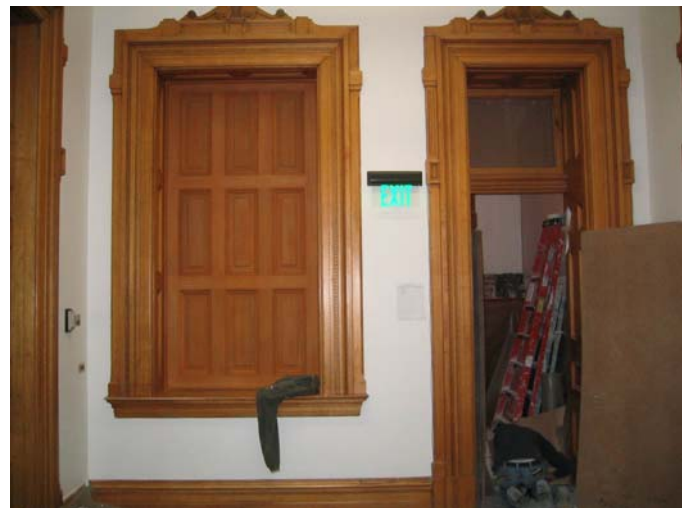
Remodeled window at First Floor Northwest Stair during construction
