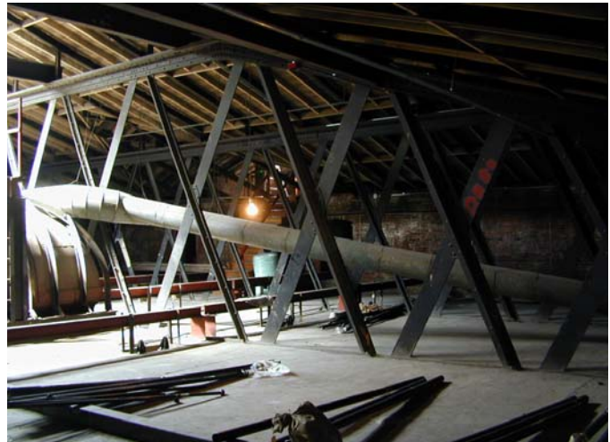
Attic: Iron trusses
