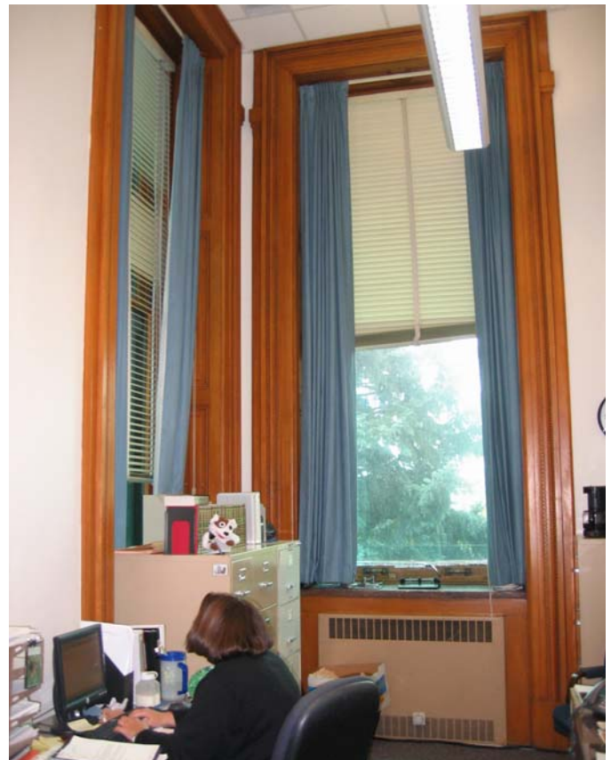
146 Exterior windows at southwest corner
