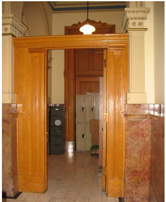
253 Looking west at in-filled door to Room 247
