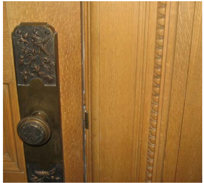
273 Restored door and trim detail
