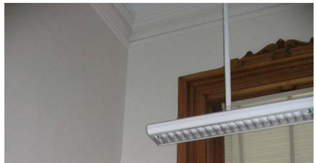
227 Wall, window and cornice detail
