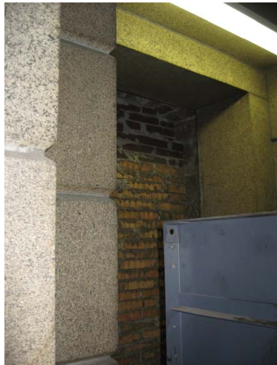
0116 Brick in-fill of original interior window
