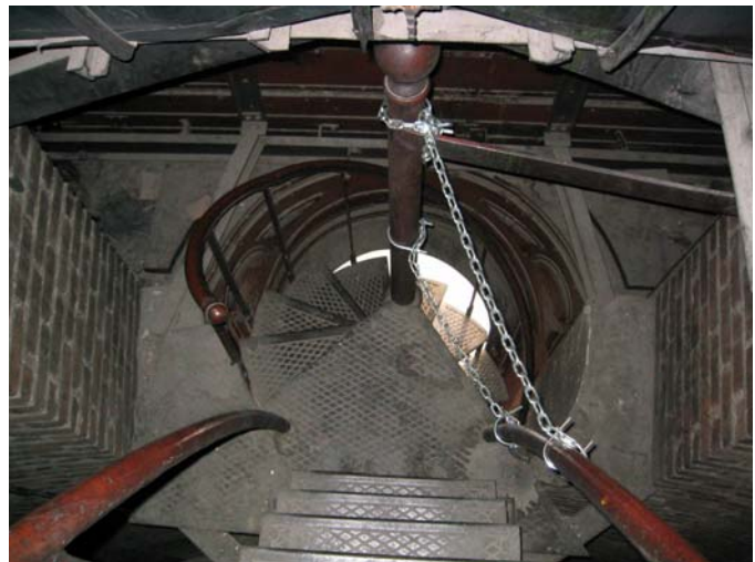
Stair to Upper Dome
