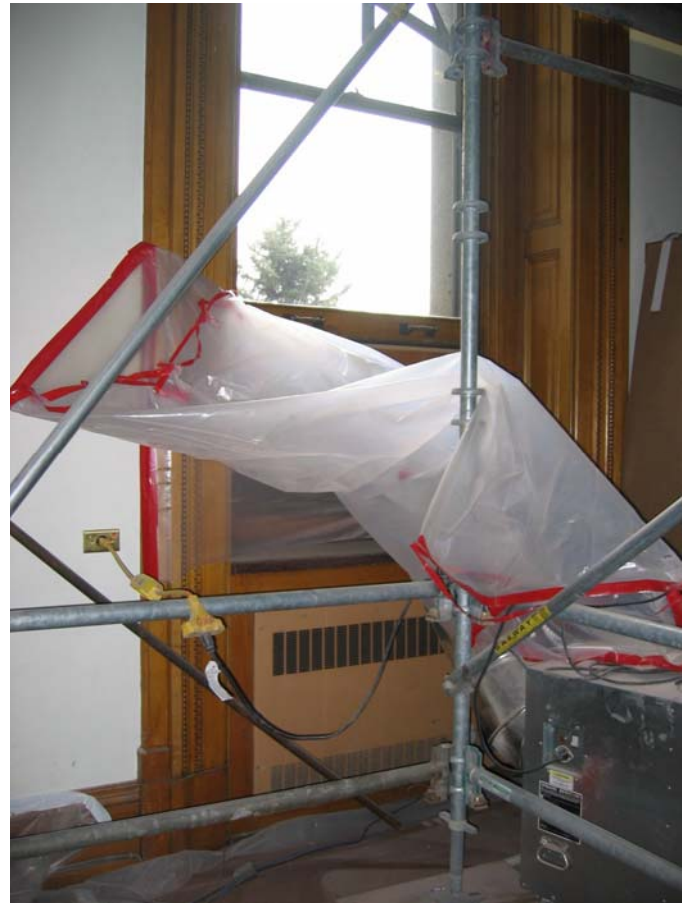
119A Window with non-original radiator
