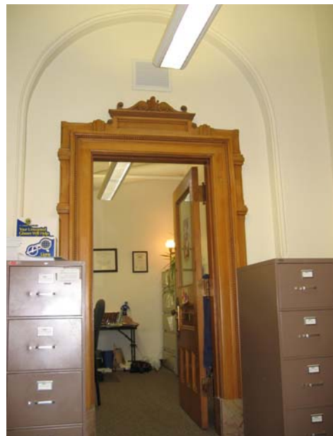
090 Looking north at former archway into 092
