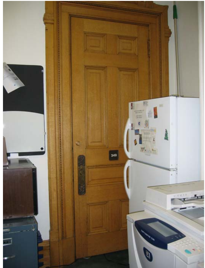
349 Entry door from Room 346
