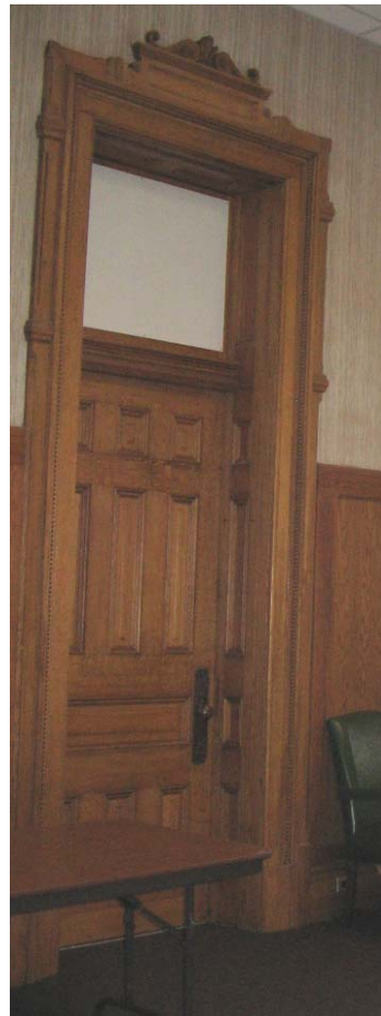
326 Interconnecting door to Room 329
