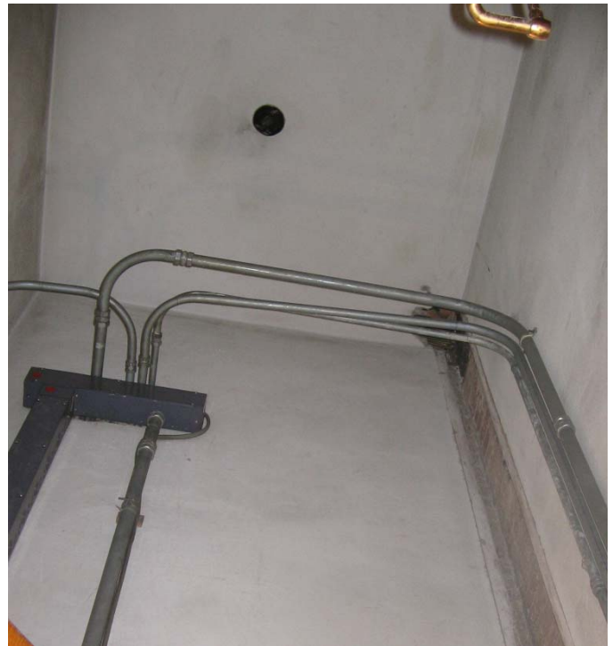
137 View of ceiling
