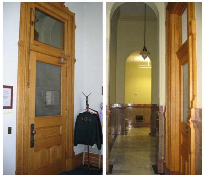
330 Door to Hallway 328 from 330 side
