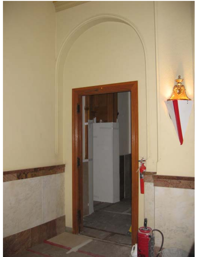
007 In-filled arch looking from Arcade
