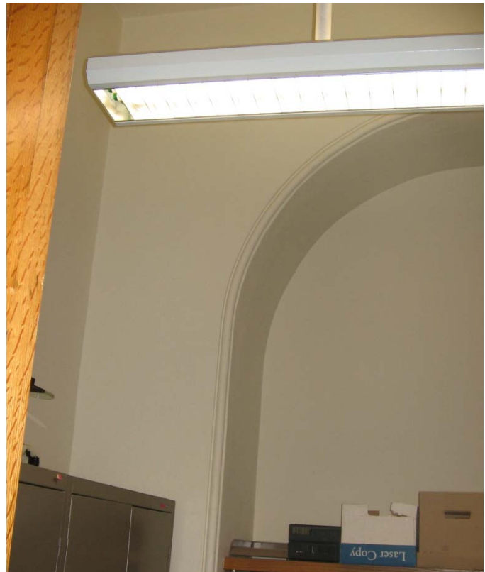
0105 In-filled arch opening in east wall
