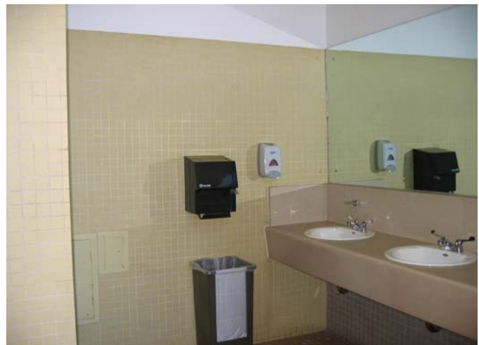
262 View of sink area
