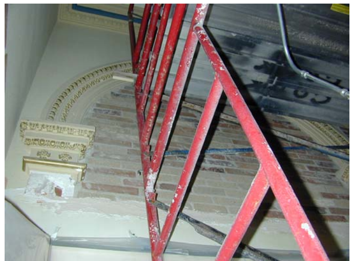
230 Remnants of former arched opening above ceiling
