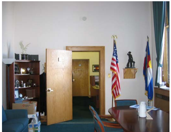
244 Non-original slab door and trim work on the south wall
