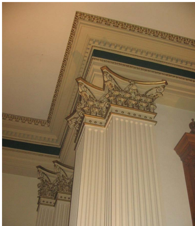
Capital detail at Third Floor Arcade
