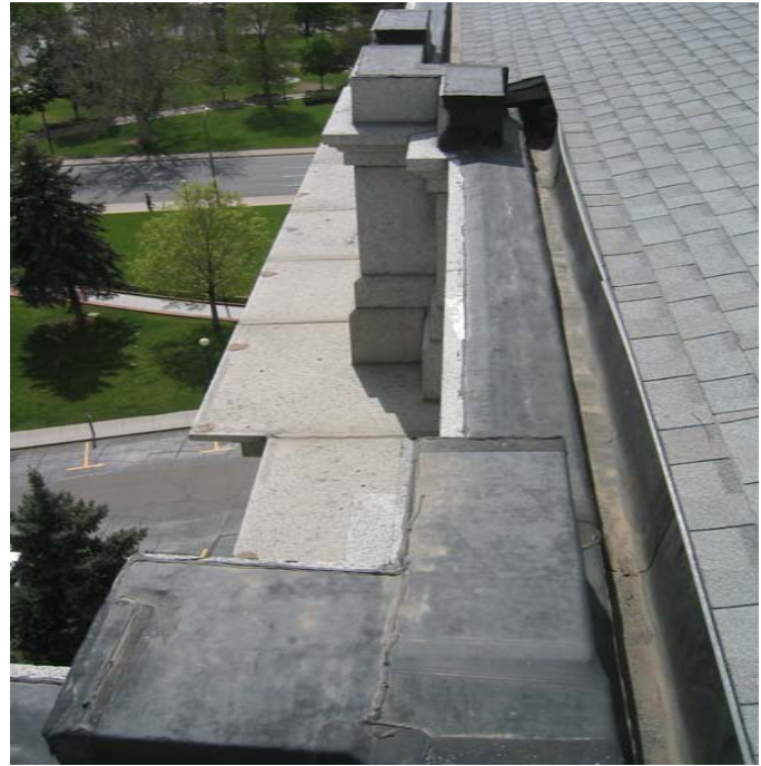
Integral gutter behind parapet wall, lined with EPDM
