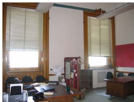
323 Existing wood trim
