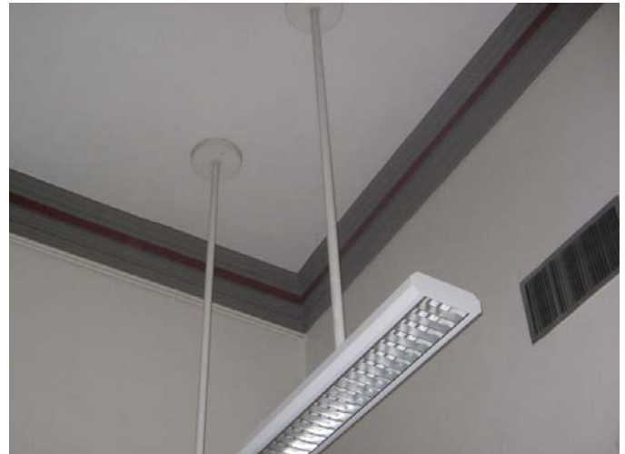
263 Existing cornice detail
