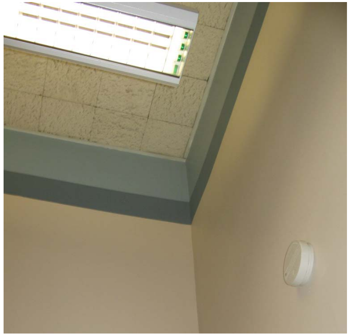
161 Existing ceiling conditions
