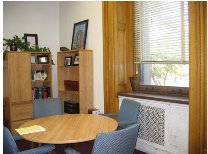
121 Cast iron radiator cover on east exterior window
