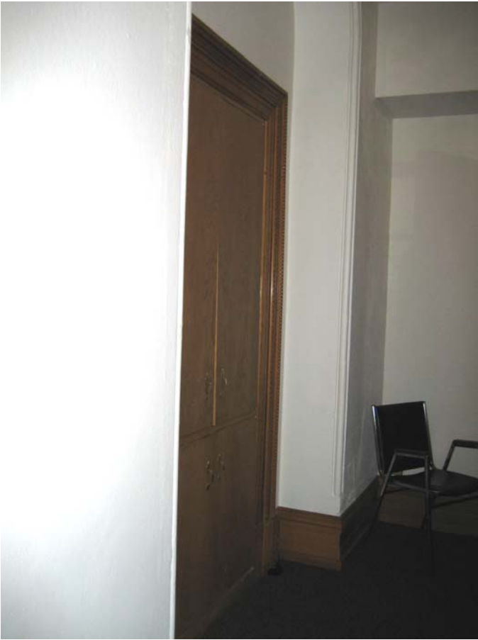
036 Cabinet installed in in-filled original archway
