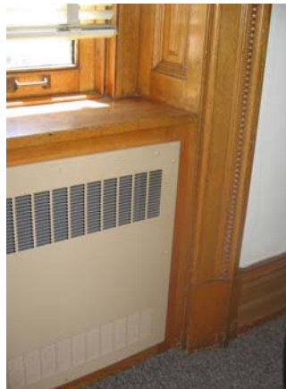
084 South wall window detail
