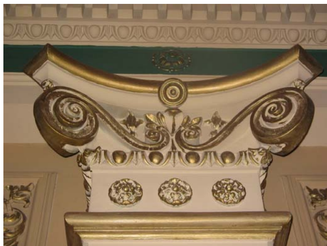
House Chamber pilaster capital detail
