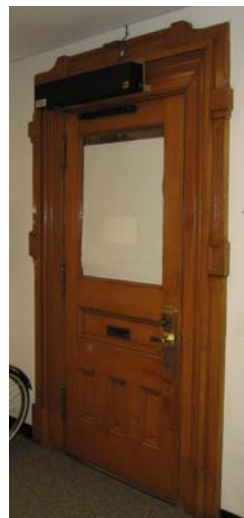
054 Interior of entry door
