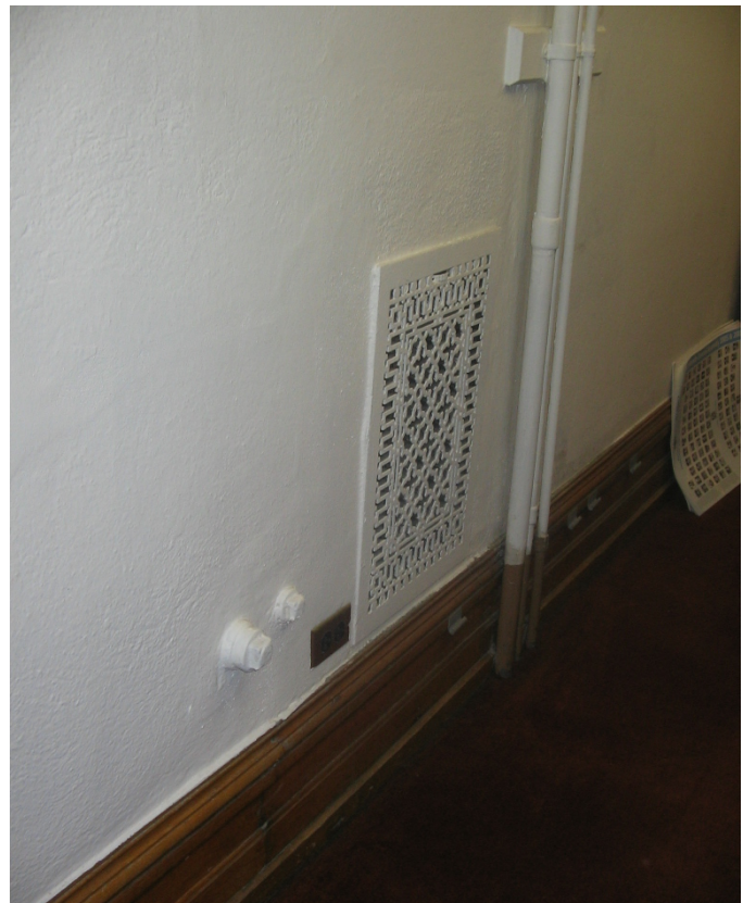
009 conduit and abandoned pipe connections
