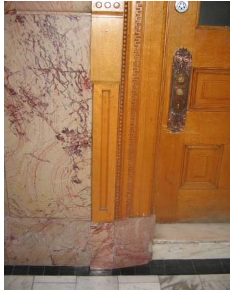
311A Existing original detailing at restroom door
