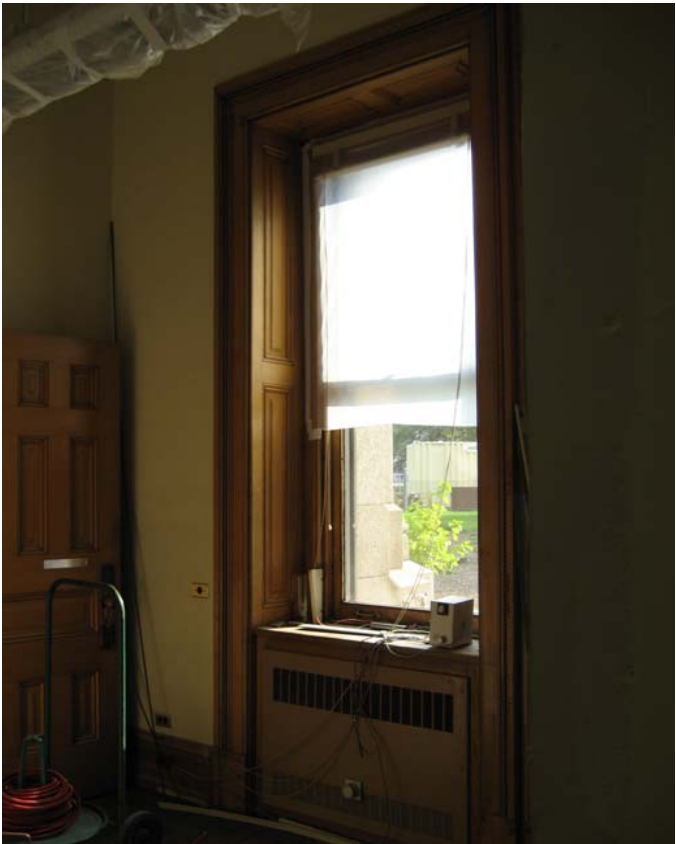
010A Exterior window on east wall
