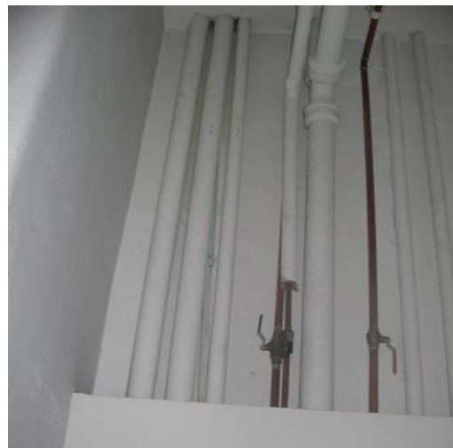
055 Exposed piping on north wall
