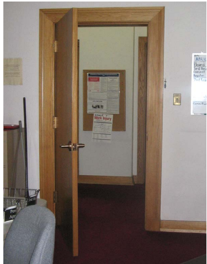
252 Non-original door on north wall
