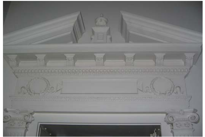
105A Original vault finishes have been painted over
