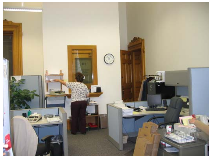
141 View of non-original transaction window on east wall
