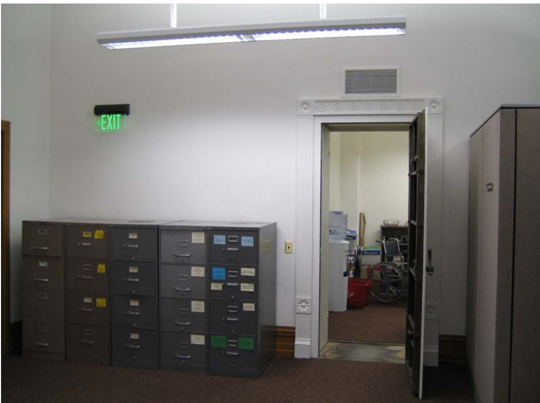
045 East wall original vault door to 045A
