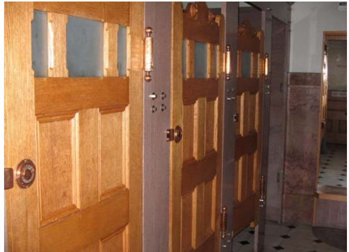
340 Original Cedar marble partitions and oak stall doors
