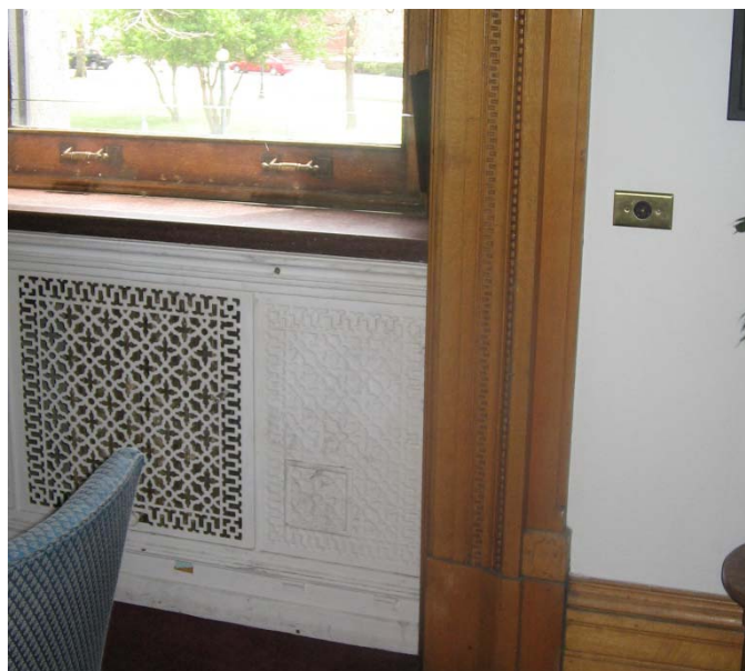
127A Radiator at exterior window with Cedar marble sill
