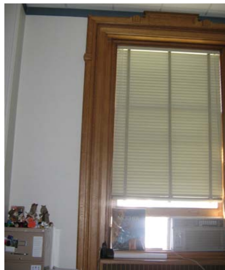
333 South wall window with corded corner
