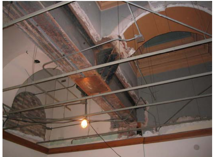
130 Steel shoring at removed column.
