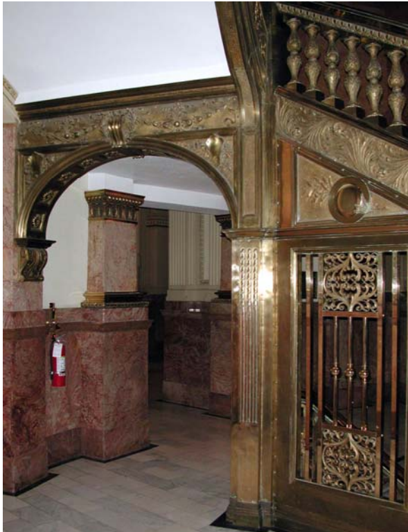
Brass arches at First Floor Rotunda grand stair
