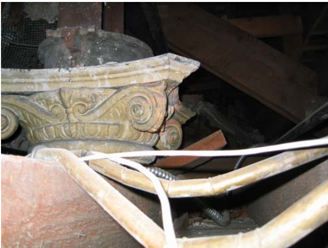
Iron column capital concealed above the House Vestibule ceiling
