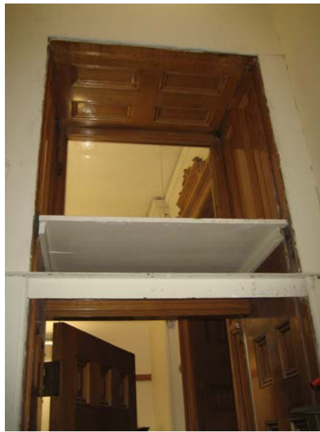
074 Remnants of original stair
