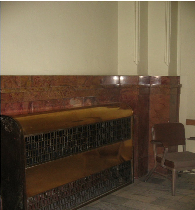
020 Vestibule looking southeast
