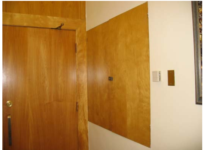
162 Cabinet on north wall, adjacent to Doors for Room 162A
