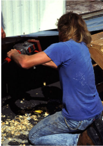
Drill holes carefully using good drill and sharp bit. Hold the drill with two hands.
