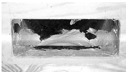
Sealing registers to the floor: This practice prevents air leakage from the crawl space or unheated basement.
