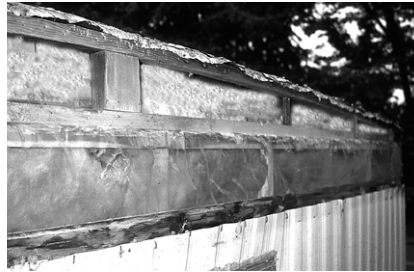
Roof cavity packed with fiberglass
