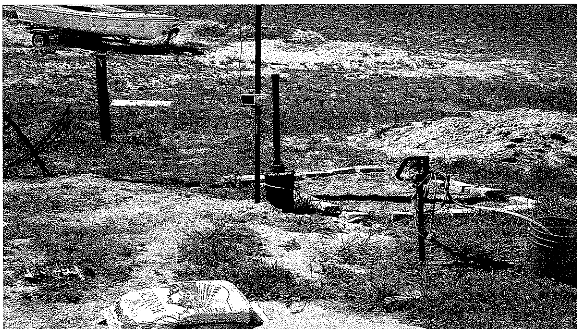
Photo 7B: Close up of well head and sample spigot.
