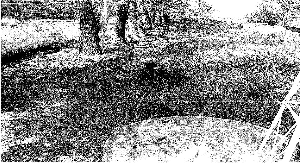
Photo 2A: Well head looking west.
