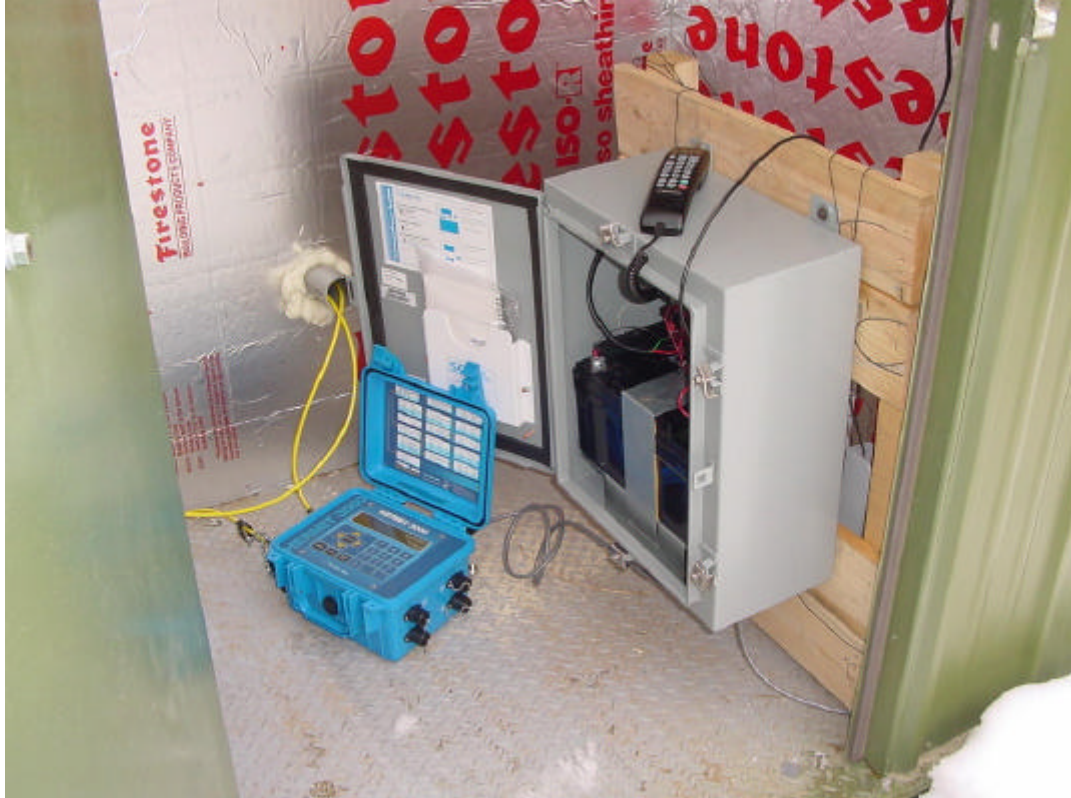
Photo 5. Hermit data logger and telemetry (temporary).
