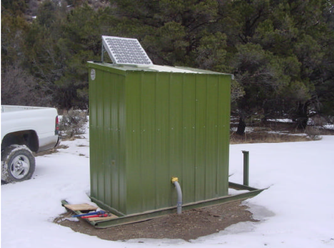
Photo 4. Basin Creek telemetry shed.
