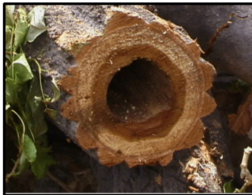
Figure 7. This cottonwood branch has a 25 percent shell, making it a potential hazard. Percent shell is measured by dividing the thickness of the healthy wood at its narrowest point (not including the reaction wood [darker ring towards the center] and the bark) by the radius of the limb (not including bark).
