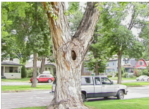
Figure 9. Structural strength is significantly compromised when the pipe-like structure of a trunk has a break in the cylinder wall.
