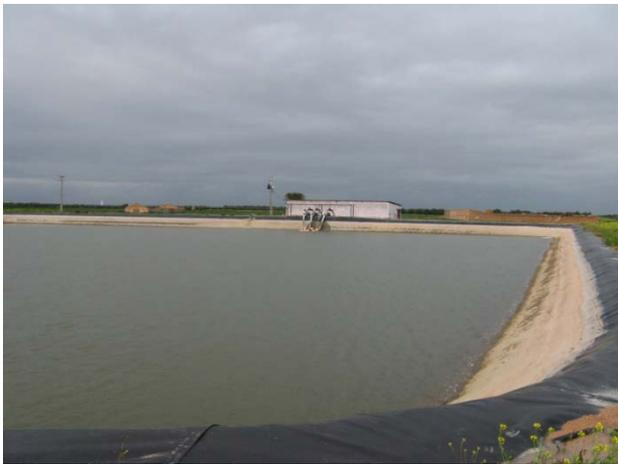
Figure 9. Water storage reservoir lined with a geomembrane. PIT, March 2009
