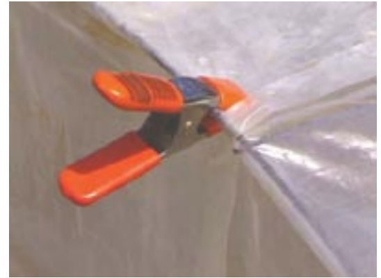
Figure 3. Hold the plastic onto the frame with small clips available at local hardware stores. Clothespins don't hold in the wind.
