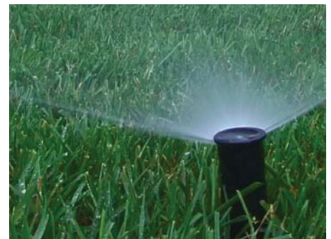
Figure 2. Make sure sprinkler heads rise above the grass height for uniform water distribution.
