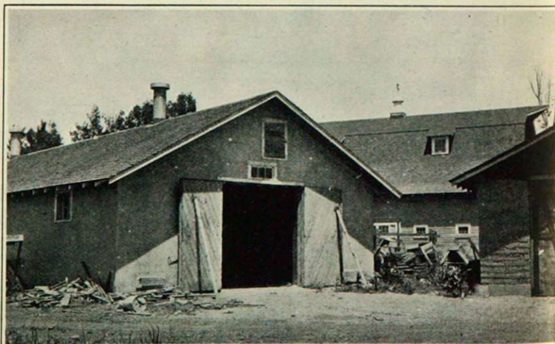
Figure 28. The walls of this root cellar are made of adobe brick and stuccoed.
