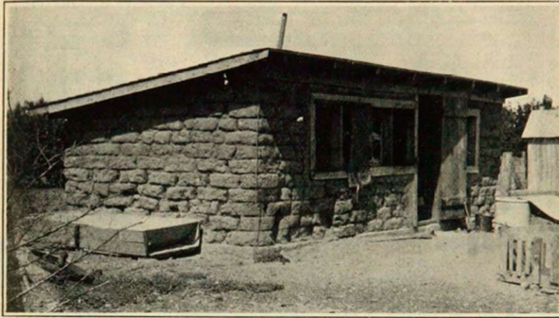
Figure 17. Adobe chicken house. Makes a house warm in winter and cool in summer.
