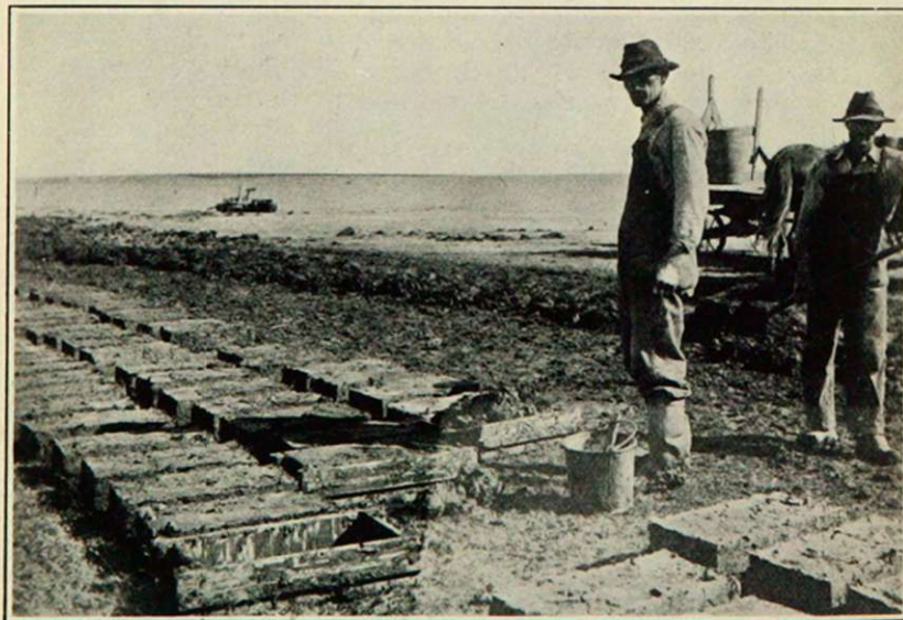
Figure 5. Molding the bricks. Notice how the bricks are molded in rows, and the position of the molds.
