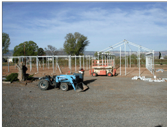
Fig. 3. Structures of the two greenhouses: the flat roof greenhouse has load bearing cables as a key structural component; trusses are the key structural component for the peak roof greenhouse. (Photo by Harold Larsen)
