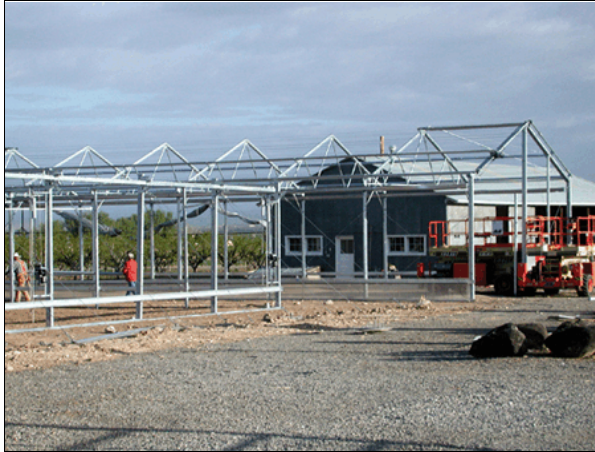
Fig. 5. A view of partially constructed greenhouses. (photo by Harold Larsen)
