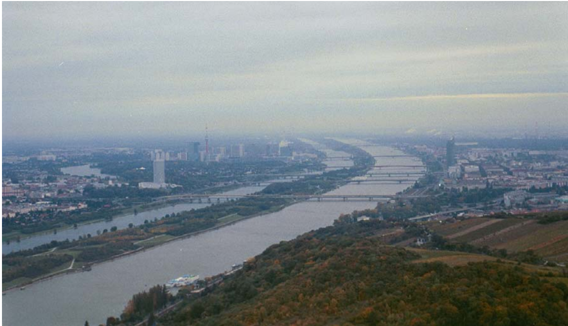
Figure 1. Phase 1 of the Flood Damage Reduction Project: New Danube in the foreground, Danube Island, and the regulated Danube.
