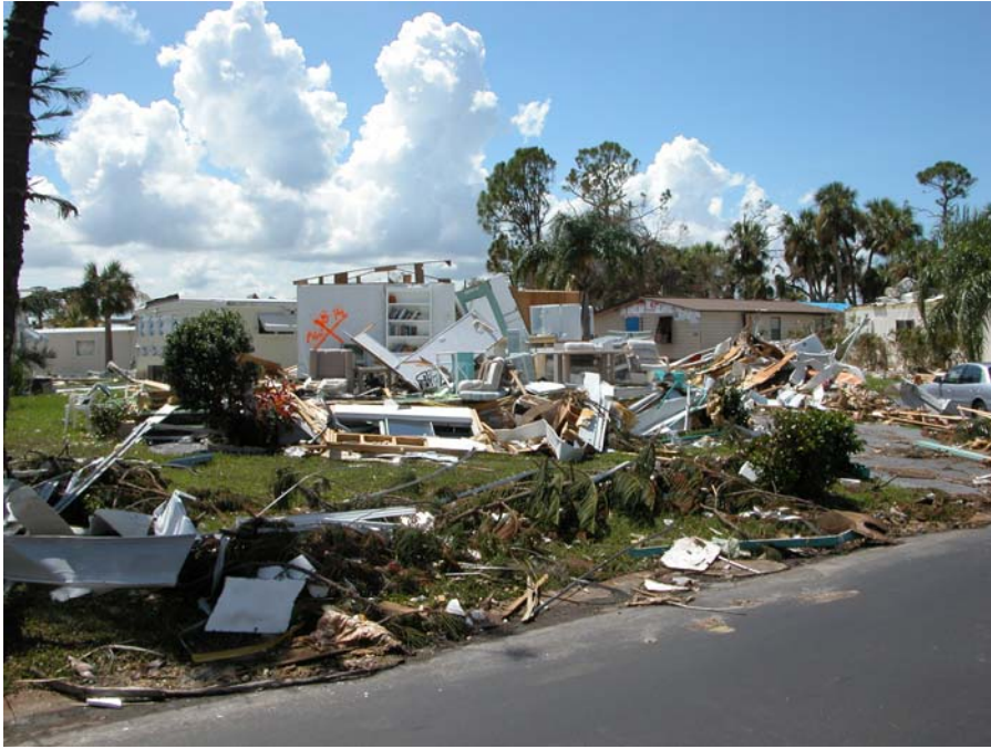
Figure 8. Differences in damage in Port Charlotte Village.
