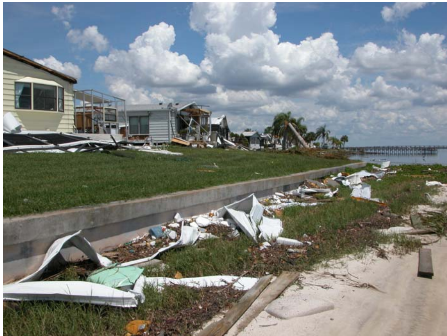
Figure 7. Harborview Park's location and damage.
