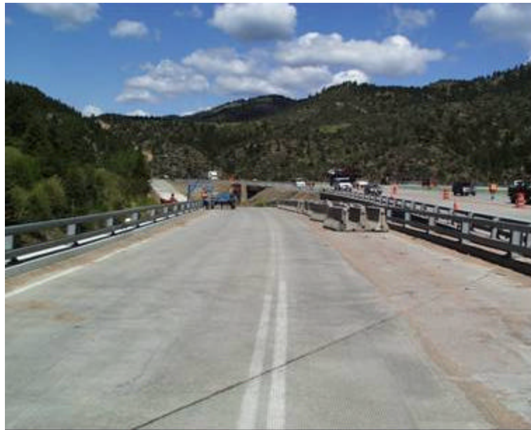
Figure F.1 F-15-BZ – the on-ramp from the frontage road to eastbound I-70
