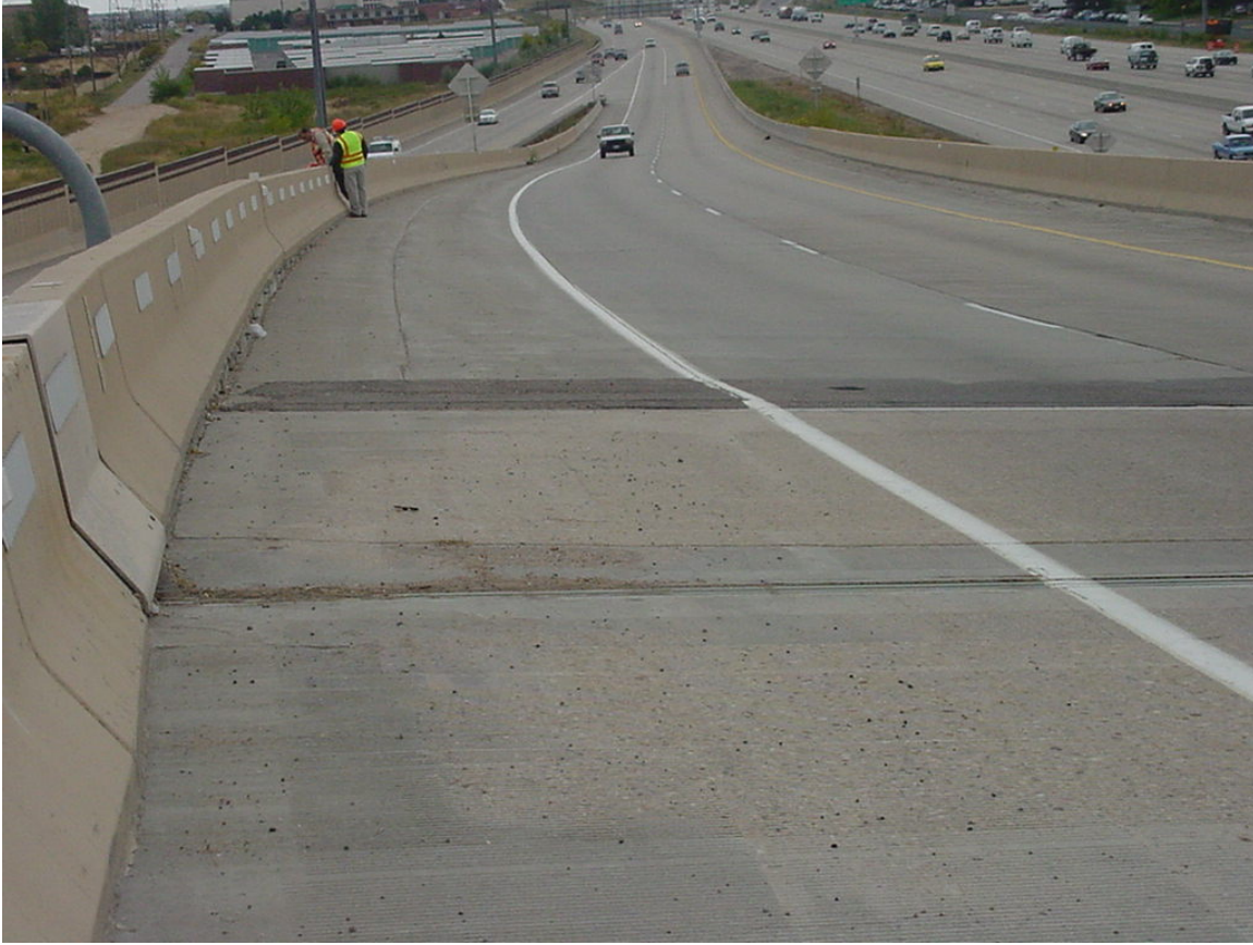
Figure C.4. The Eastern Side of the Bridge and Roadway Approaches of the I70/I-225 Interchange (Structure E-17-SW in Region 6).
