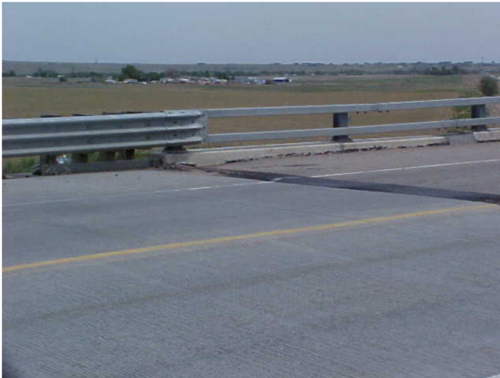
Figure C.13. Photos of Structure C-22-BT and C-21-BM in Region 4
