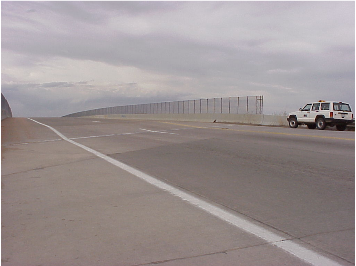
Figure C.7. The South Side of Buckley Over 1-76 (E-17-PQ, Region 6). This is a good Example of Bridge Bump Problem Generated at End of Construction.
