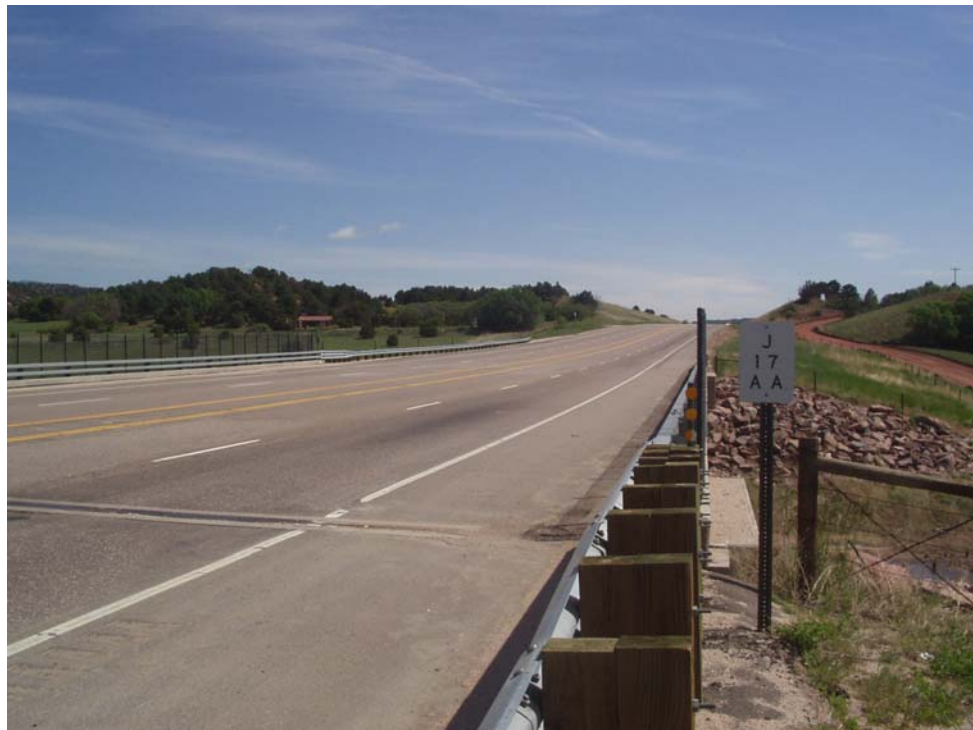
Figure C17a. Photos of Bridge Structures in Region 2 Constructed with MSE Backfill
