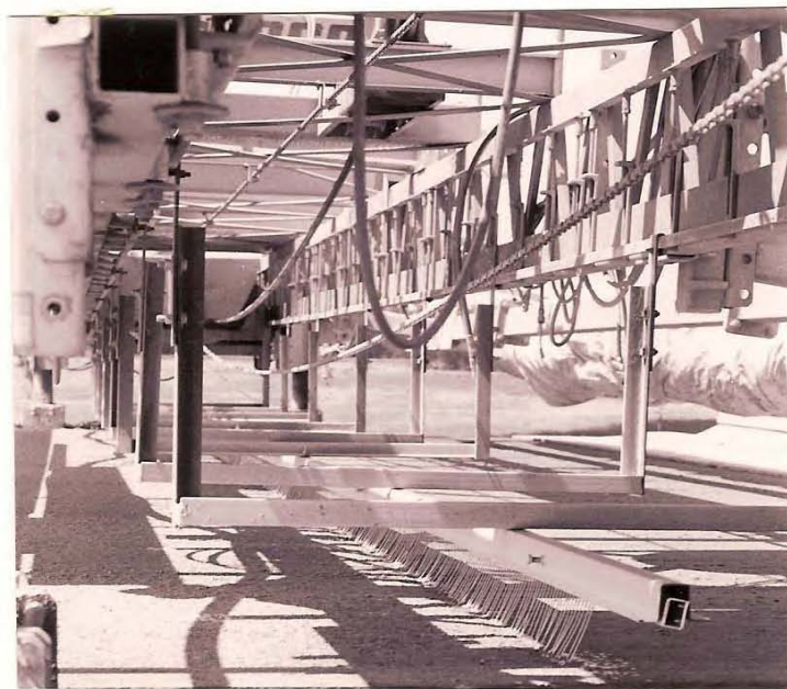
Photo 3: View of the longitudinal tining assembly
