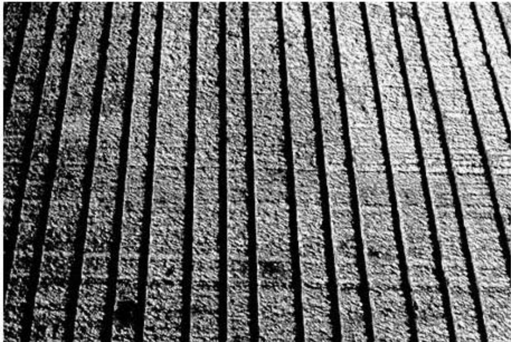
Photo 18: Close-up view of random transverse grooves with 5/8", 7/8", and 3/4" spacing
