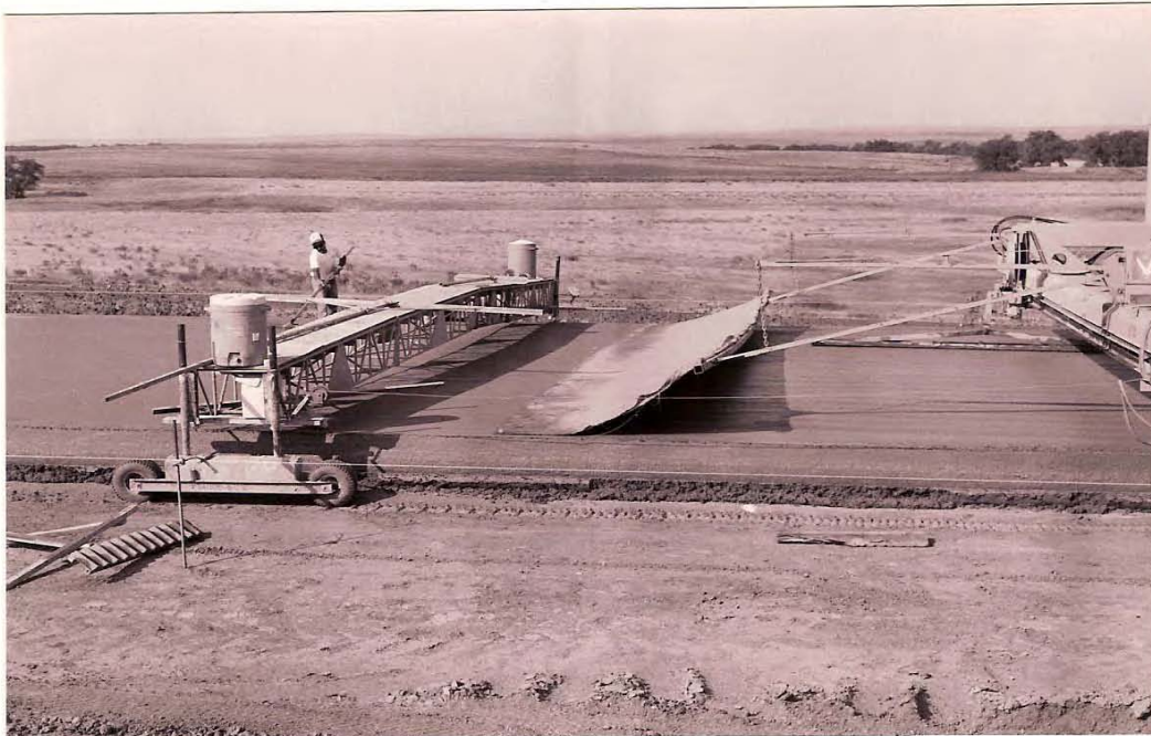
Photo 2: Burlap drag was applied to all test sections
