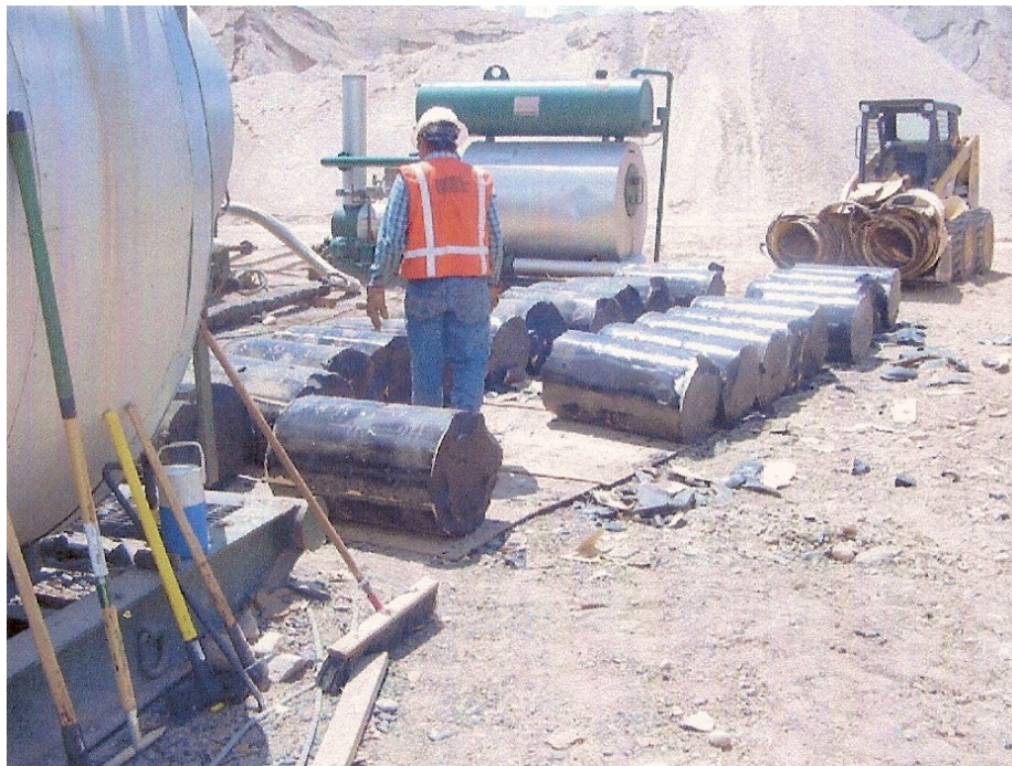
Figure 7. Trinidad Lake Asphalt Ready to Blend in Asphalt Tank
