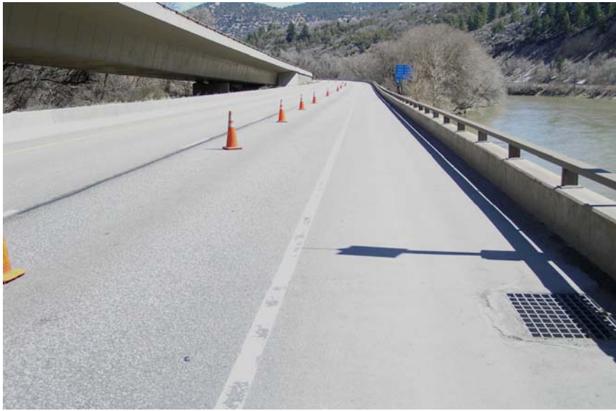
Figure 15. EB Section 3 in Excellent Condition (2005)
