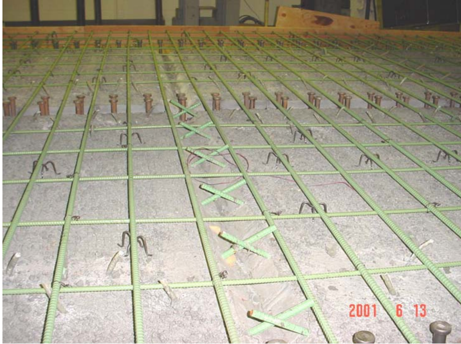
Figure 5.5 – Panel Splicing
