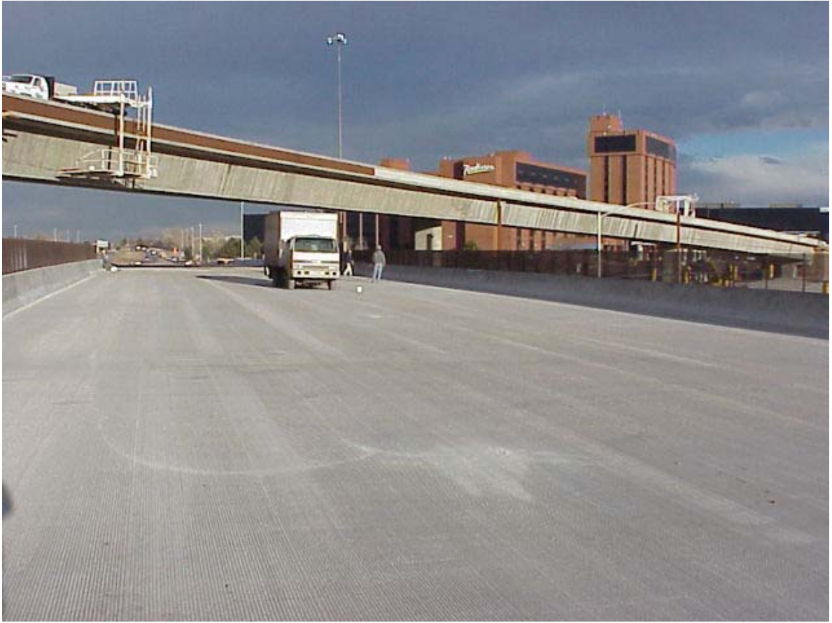
Figure 1.1 – I-225/Parker Road Bridge under Construction
