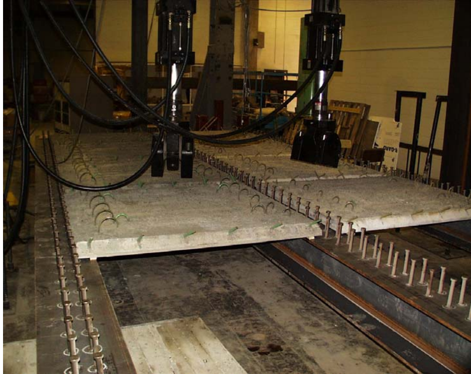
Figure 5.3 – Installation of Precast Panels
