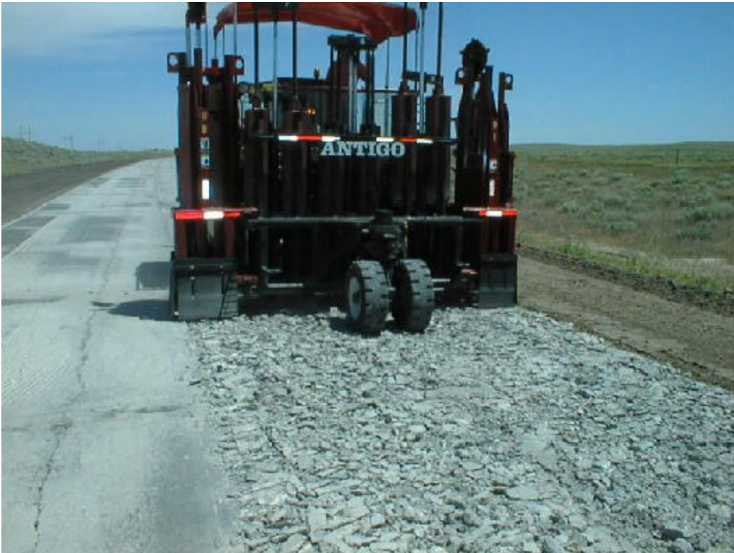
This multi-head hammer truck is rubblizing this concrete pavement.
