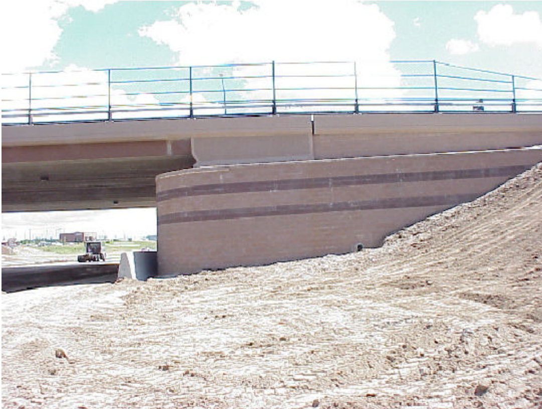
The Founders-Meadows Parkway bridge in Colorado Springs uses geosynthetic-reinforced soil walls.
