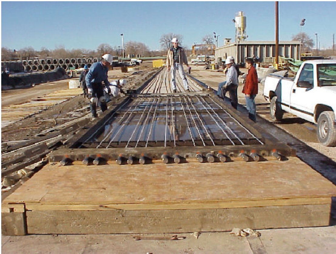
This photo shows a prestressed carbon fiber precast bridge panel. This project is the first time that CDOT has not used steel for reinforcement.
