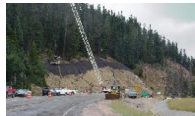
Above: Installation of erosion control materials on SH 40, west of Berthoud Pass. Left, counting the type and number of plants that are growing on the rehabilitated slope. And yes, the man is attached to a safety line.
