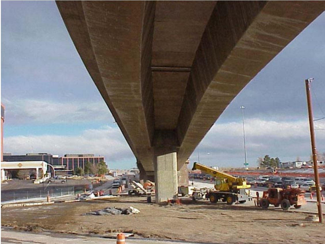
Figure 1.2 – Precast Panels Supported on Two Box Girders
