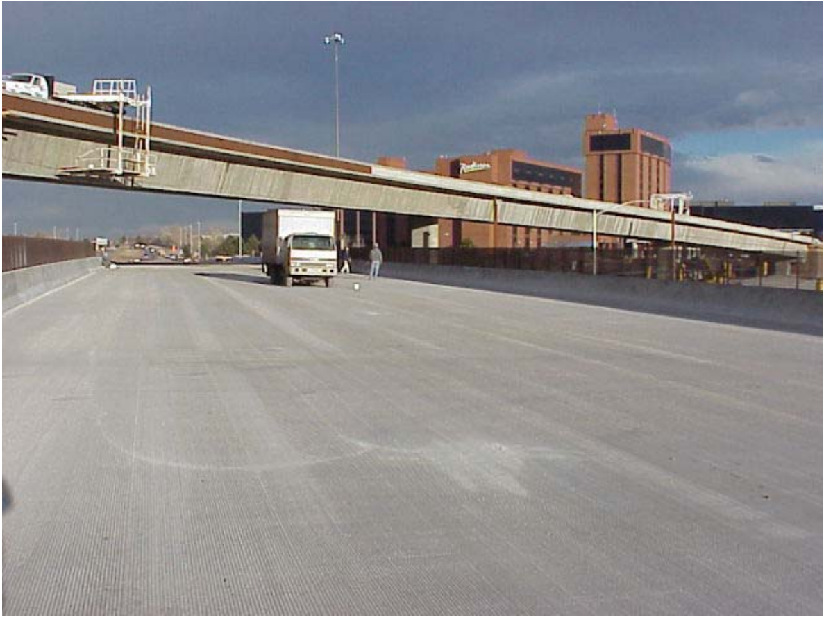
Figure 1.1 – I-225/Parker Road Bridge under Construction
