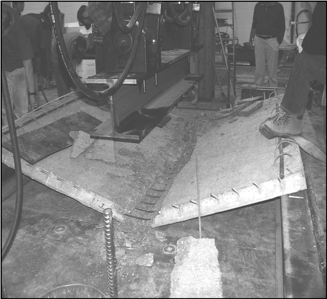
Figure 4.11 - CDOT Panel Failure
