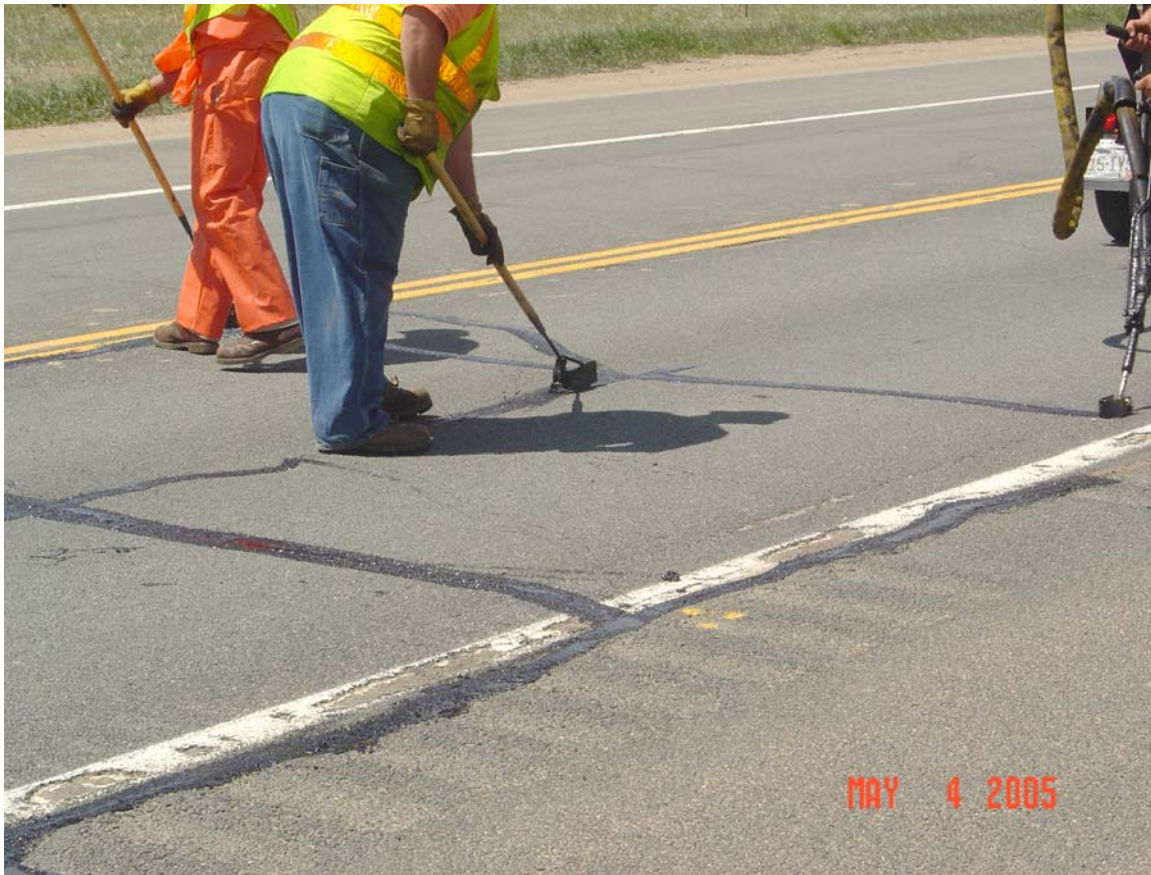
Figure 7 – Squeegee Application After Crack Pouring
