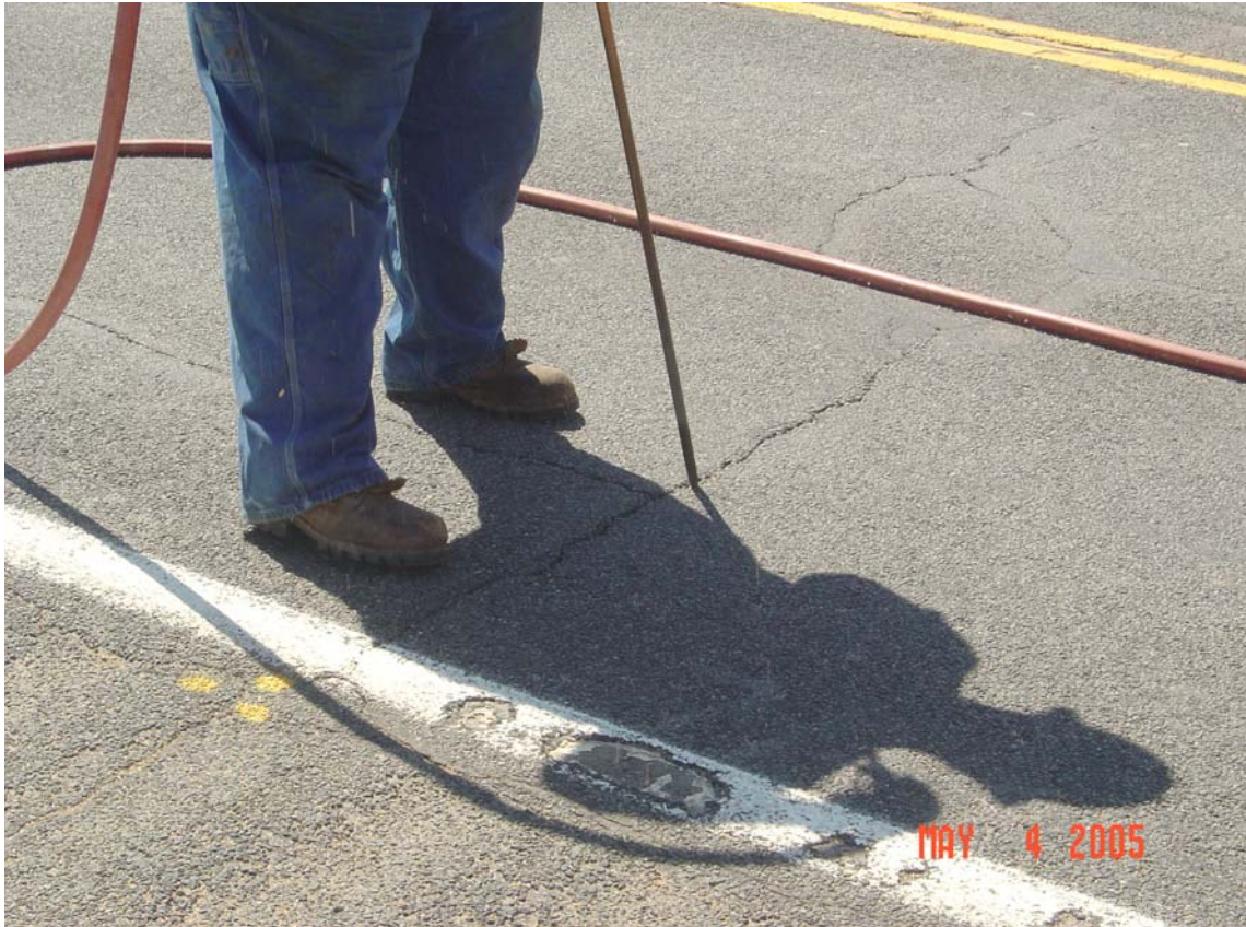
Figure 4 – Cleaning Crack with Compressed Air
