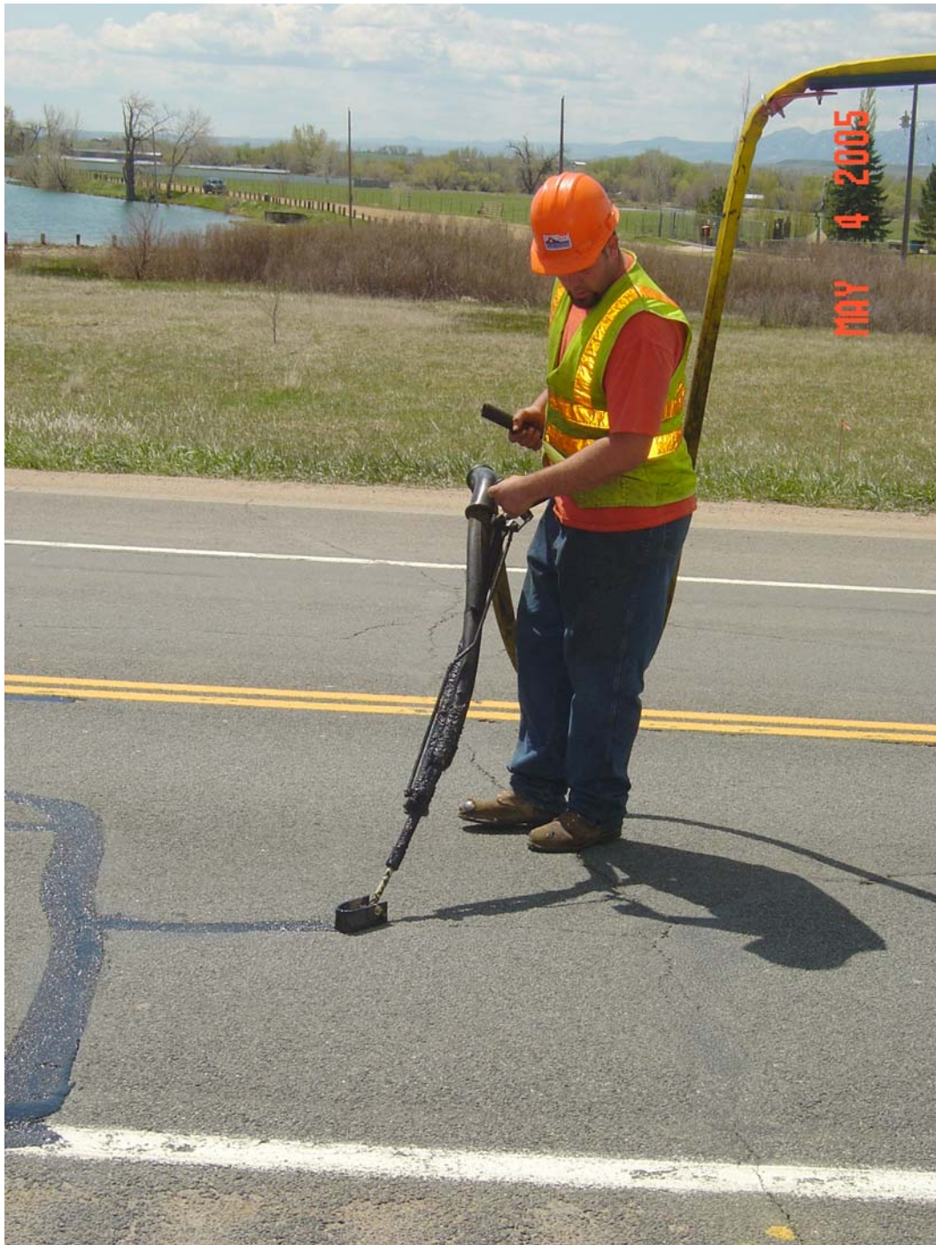
Figure 6 – Pressure Distributor for Crack Sealing
