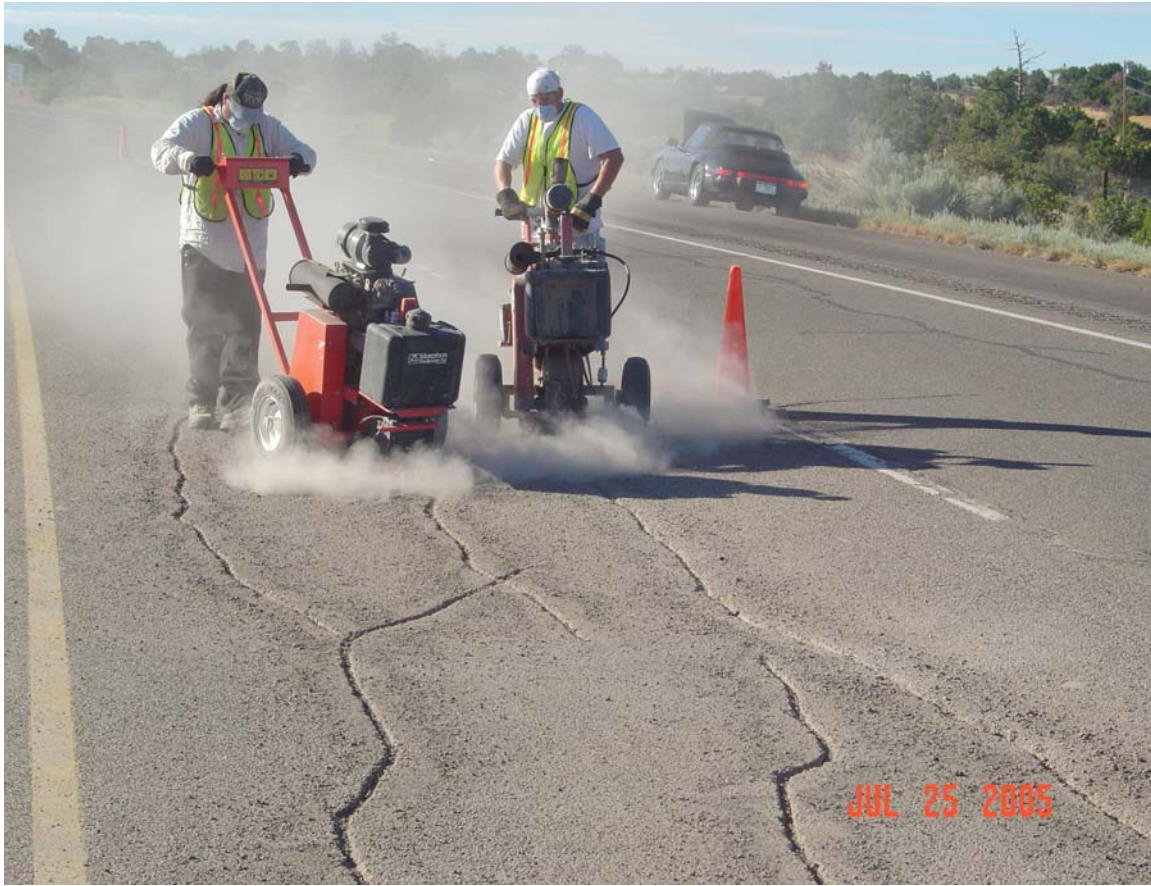
Figure 1 – Routing Cracks Prior to Crack Sealer Installation on I-25, NM
