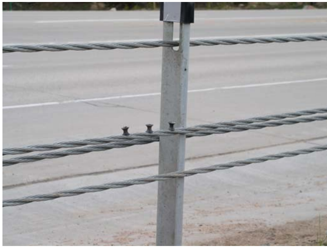
Figure 6. Cables positioned lower than design height.
