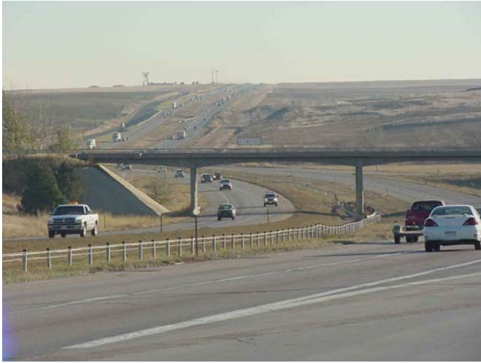
Figure 3. The I-25 – SH-56 interchange, looking south.
