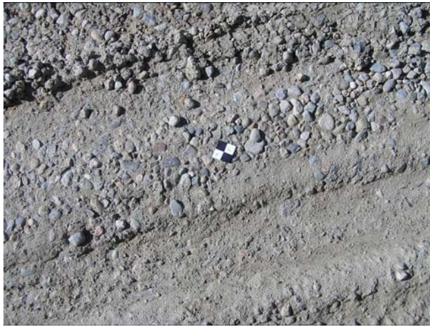
Figure 2. The Lower Straight Creek arrester bed near the entrance. The references are 1" squares.
