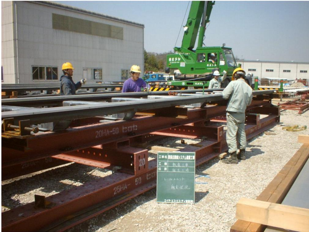
Figure 46: Levitation Rail Section Assembly Prior to Installation
