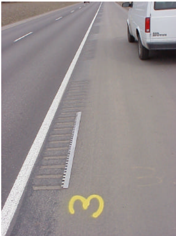
Figure A-10. Section 3 was ground in an interrupted pattern.
