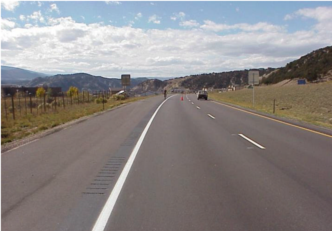
Figure 19. A cyclist on one of the new 2 inch rumble strips. This is a section of interrupted rumble strip
