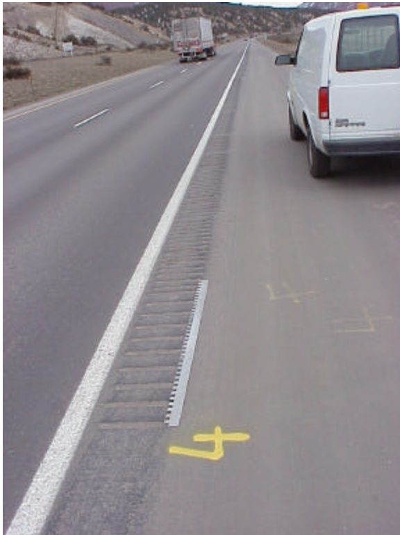
Figure A-11. Section 4 starts at the far end of the straight edge. Grooves are 2 inches wide but with only 3-inch flats between. Section 4 is continuous rumble strip.
