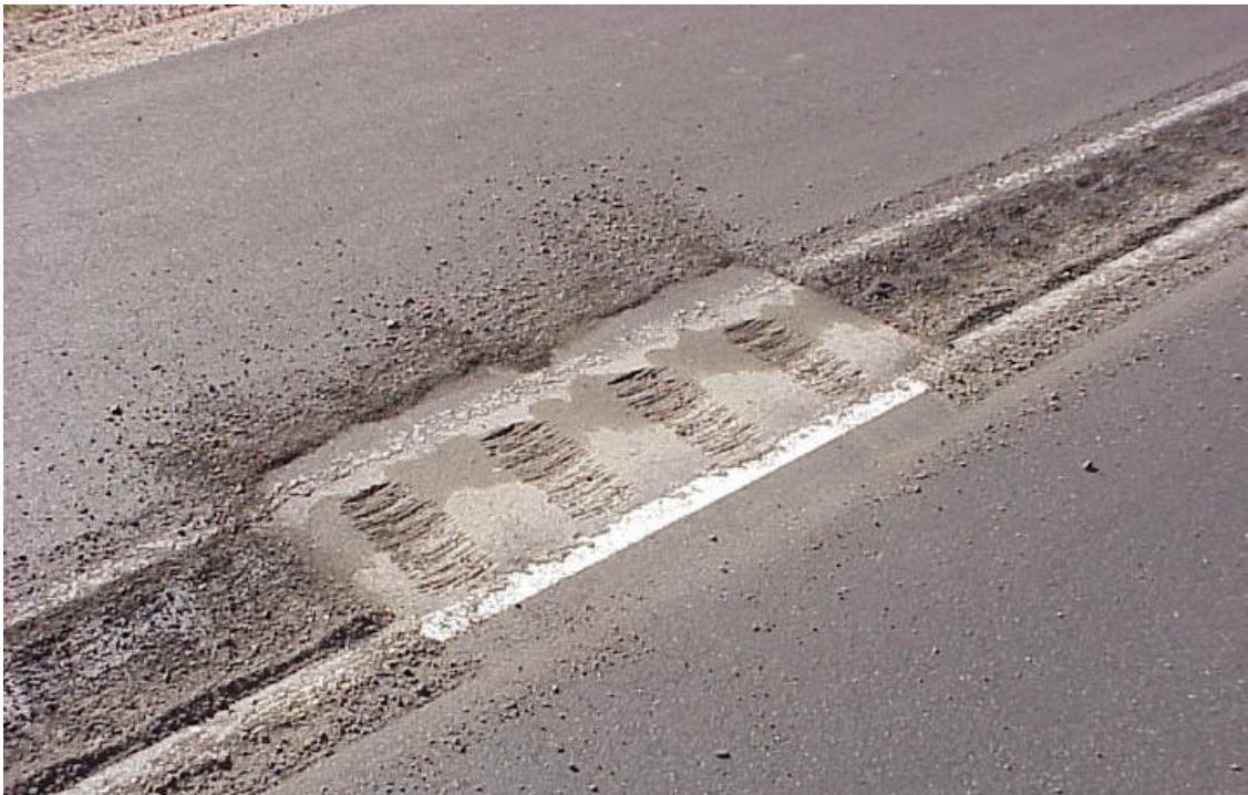
Figure 4. The standard rumble strip. This is one of the shallower sections. The operator stopped to check the grooves here. A power broom follows along to sweep the grindings off the roadway.
