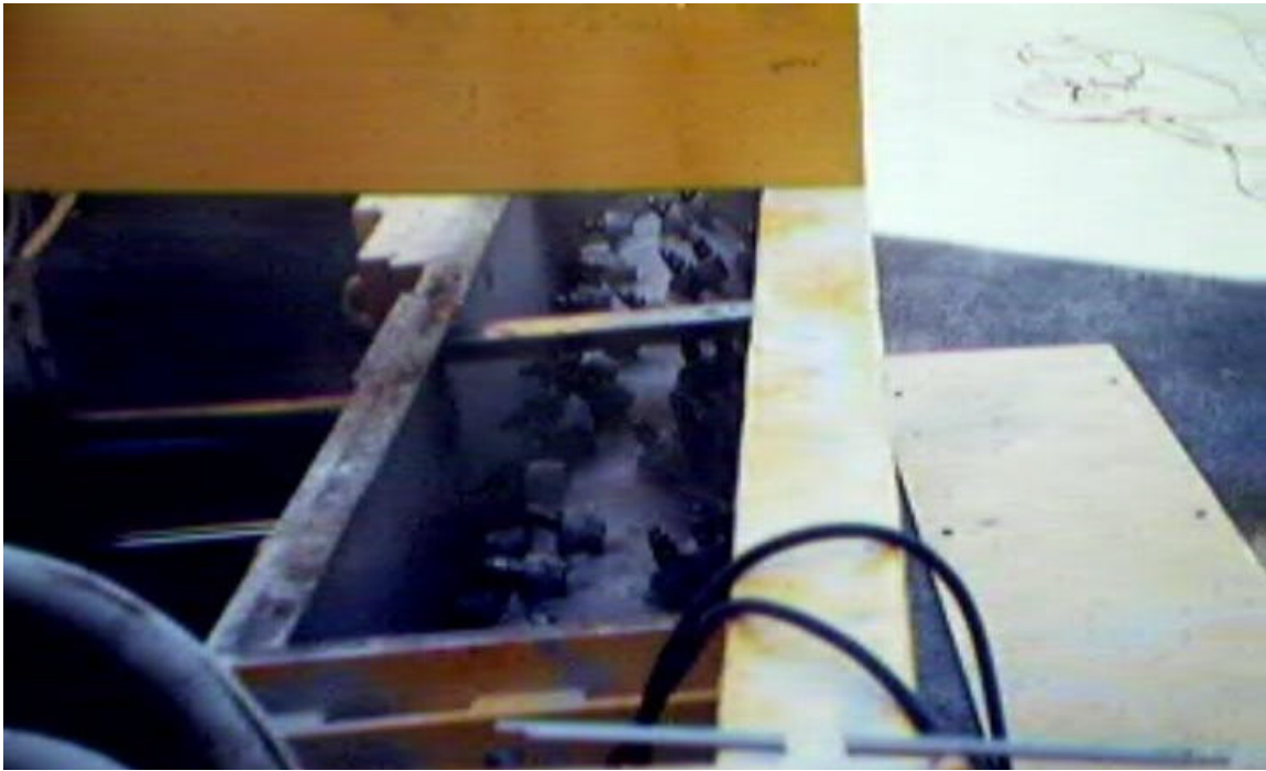
Figure 11. The grinding drum on the new two-inch-groove machine. The spaces between the sets of teeth that adjusts the spacing of the grooves can be seen. The spinning drum is lowered into the pavement and moved to the left to cut the rumble strip grooves - six feet at a time.
