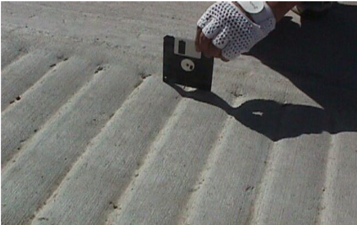
Figure 17. The concrete rumble strip on US 34 east of Greeley. This strip is 18 inches wide with grooves on about 3-1/2" centers. The light below the floppy disk shows the depth of the groove - about 1/2" which is at the low end of the allowed range of 1/2" to 1".
