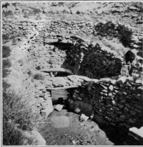
This illustration shows the spring above the Pueblo of Mishognovi, Arizona, where water originates to irrigate terraces shown in the next following illustration. These Hopi Indian irrigation works in modern use are the counterpart of ancient construction being uncovered in the sands of the southwestern deserts.
