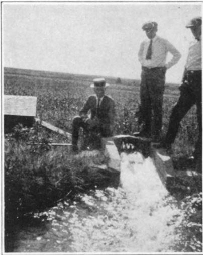
Supplementary irrigation by pumping the underflow in a creek bottom in the dry land region. Illustration shows outlet pipe of pumping plant on Beaver Creek, ten miles south of Brush.
