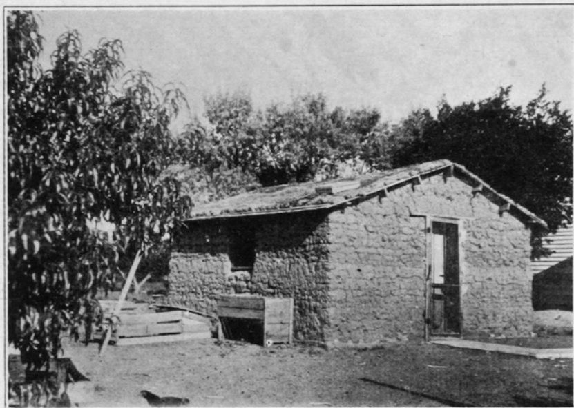
Type of adobe farm storage house on Cheyenne Wells Dry Land Demonstration Farm.
