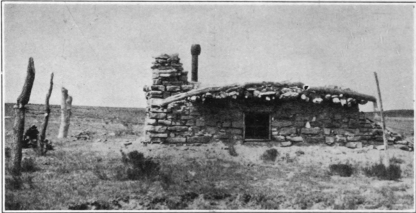
A homesteader's first habitation in southern Colorado. Dugout with superstructure, built from un-trimmed stones picked up in bed of dry water course.
