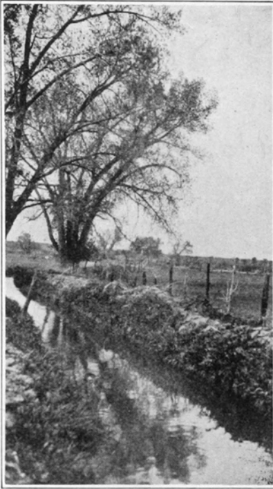
A lateral ditch carrying water from the main canal to the fields.
