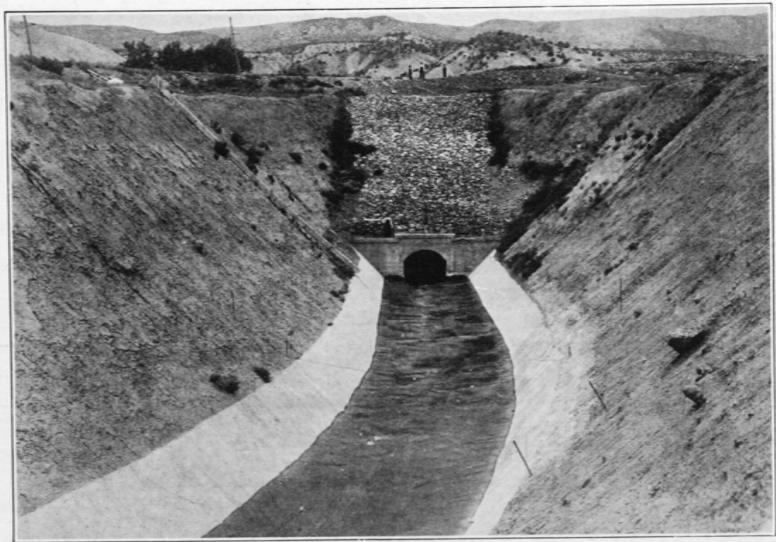
Outlet of the Gunnison Tunnel.
