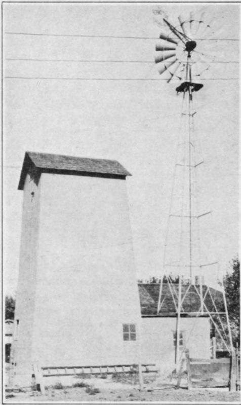
Windmill tower and tank for domestic water supply on Cheyenne Wells Demonstration farm.
