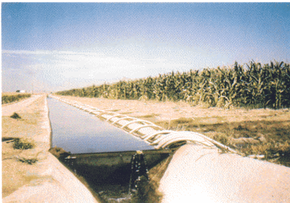
Concrete lined ditches reduce seepage losses.
