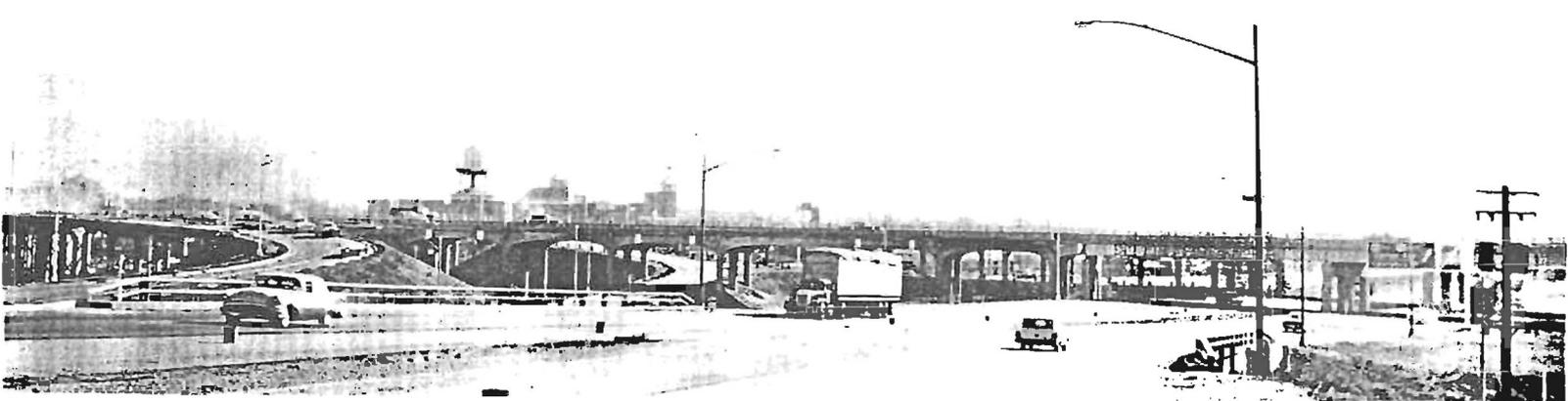
**SOUTHBOUND TRAFFIC** (middle photo) leaves the Valley Highway via a ramp which loops beneath the West Colfax viaduct, the Valley Highway and the Larimer viaduct and connects directly with the Lawrence structure. An exit direction sign informs motorists of the turnoff 1,000 feet before they reach the exit. The sign in this photo is partly covered pending opening of the complete facility.
