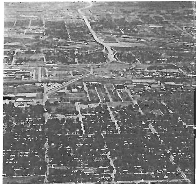
THE FUTURE CONTINUATION of Interstate 70 is shown in the lower right photo as the route proceeds westerly from the East 46th Ave. interchange in the center of the picture. The route runs diagonally toward the left of the photo and then follows West 48th Ave. to Federal Blvd., which extends across the bottom of the photo. The kink in the East 46th Ave. Freeway near the top center of the photo is overemphasized because the picture was taken with a telephoto lens.
