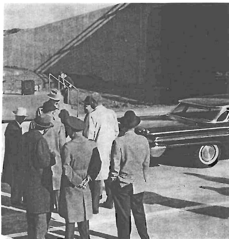
FEDERAL, STATE AND CITY OFFICIALS gathered in 1961 to dedicate the jet runway overpass, north of Stapleton Field, which goes over the six lanes of the East 46th Ave. Freeway, as shown in the photo above.
