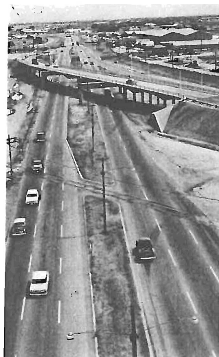
THE OVERPASS CONNECTING COLORADO BLVD. WITH INTERSTATE 80-S AND US 85
