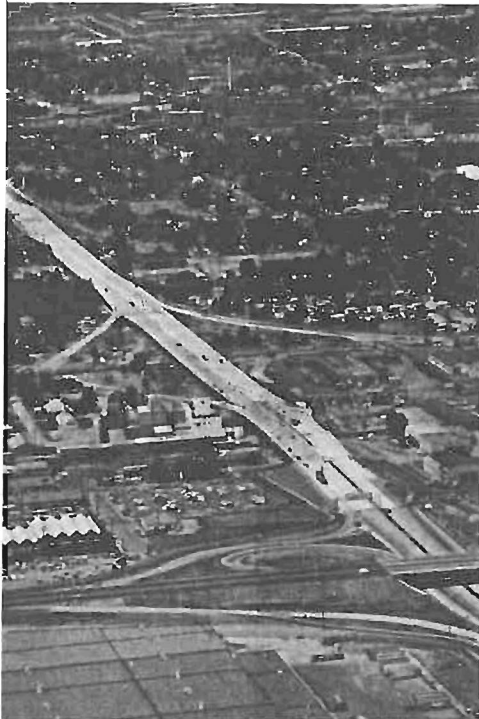
THE STEELE-ST. VASQUEZ BLVD. INTERCHANGE
