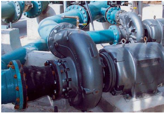
Figure 15: Reaction Turbine (PAT)
