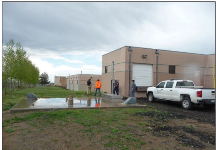
FIGURE 1: PRV VAULT (FOREGROUND) AND WATER TREATMENT PLANT
