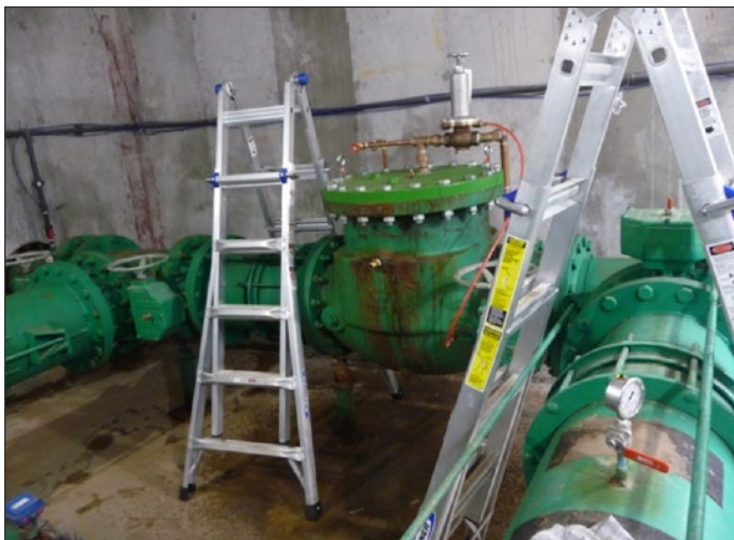
FIGURE 2: PRESSURE REDUCING VALVE
