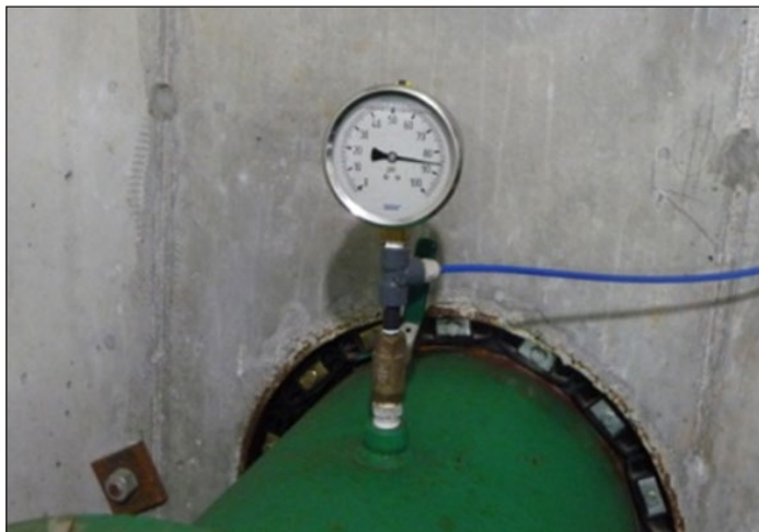
FIGURE 4: STATIC PRESSURE - PRV VAULT
