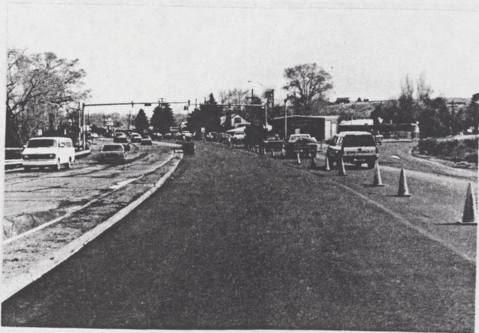
The Gilsonite test section was placed at the UnawEEP intersection.
