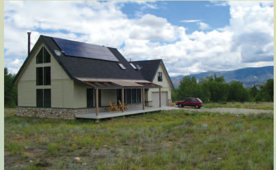
Photovoltaic solar installation on an extremely energy-efficient home in Nathrop, CO. Architect: Keith Krebs. Utility: Sangre De Cristo. Installation and photo: Standard Renewable Energy.
