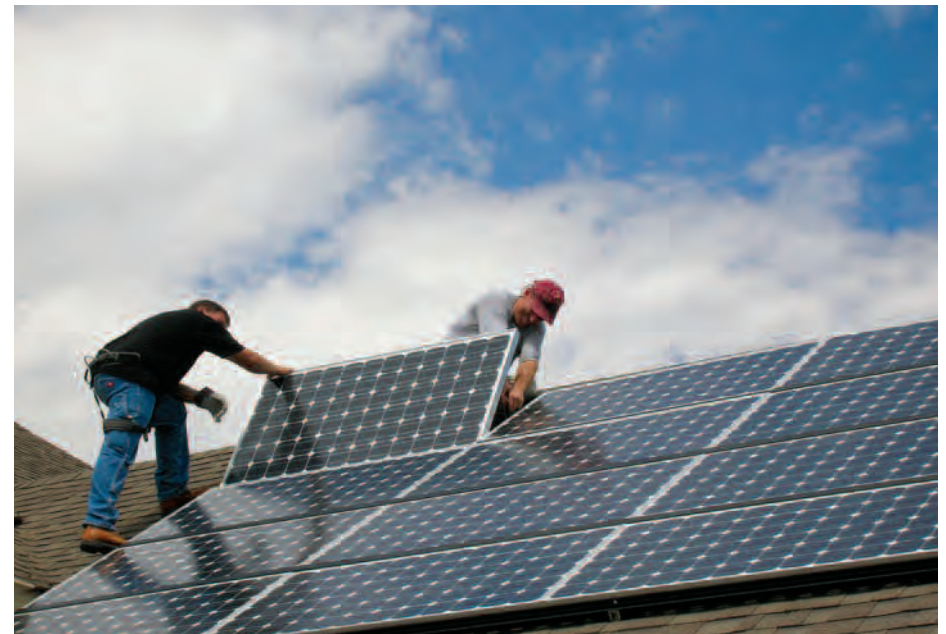
Installing a PV system. Photo: Novan Solar.
