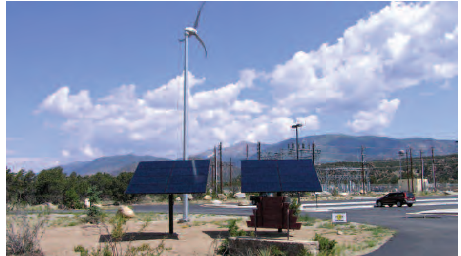
Electrical cooperative Sangre De Cristo, with help from a local energy expert, is partnering with the GEO to provide solar and wind incentive programs for its members and has installed a small wind turbine and solar-electric demonstration on its property.
