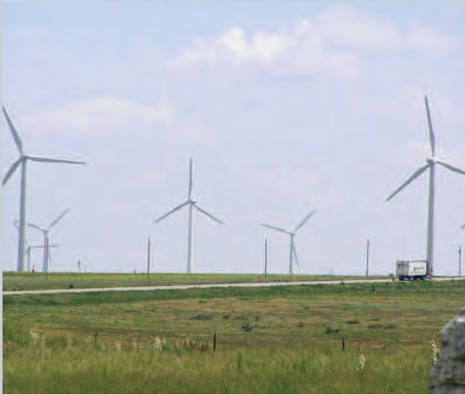
The Colorado Green wind project near Lamar. Photo: Rebecca Cantwell.
