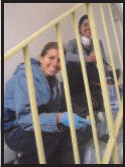
Sanding a railing.
