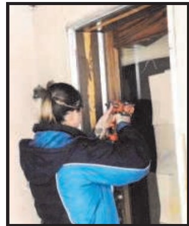
Installing weather stripping.
