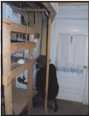
Insulating the water heater.
