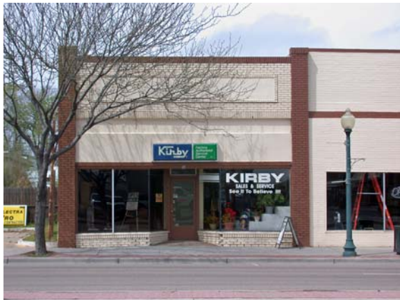
2. 205 North Main 5PW.305 Motor Supply Company ca. 1926
