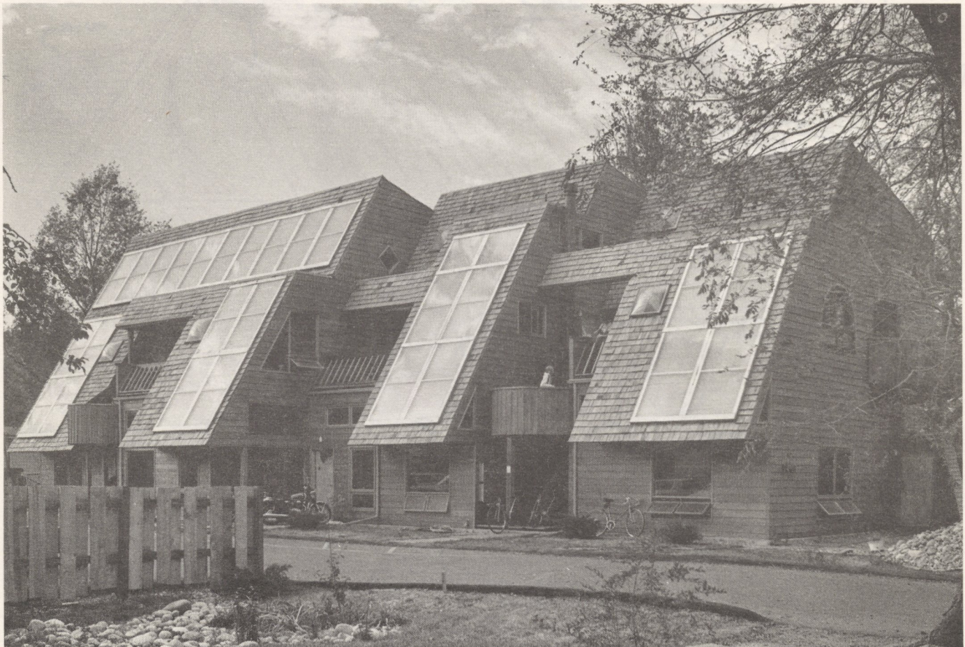
The solar system on the 19th Street Student Solar Housing in Boulder has high efficiency collectors which provide hot water for baseboard convector heating. The student apartment complex was built in 1976 with the assistance of the Department of Housing and Urban Renewal (HUD) Solar Demonstration Program.
