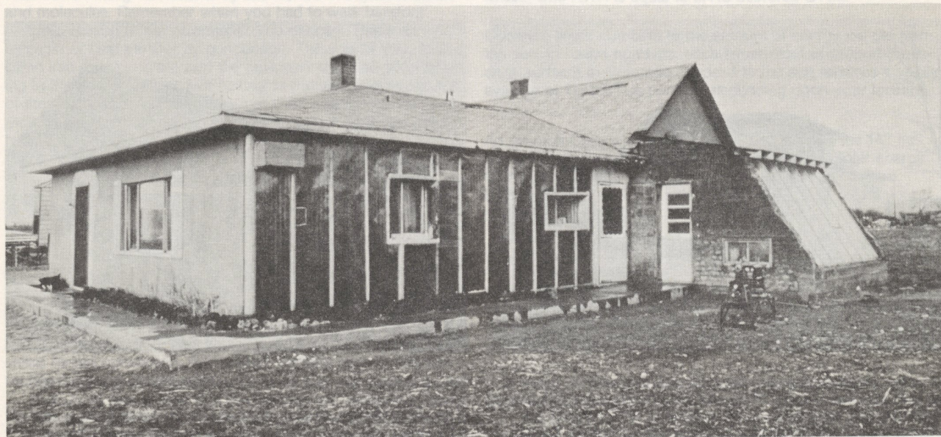
Frank Valdez's greenhouse is made mostly of recycled materials from the adobes down to the 100-year-old nails. It's a do-it-yourself, labor-intensive and inexpensive project.
