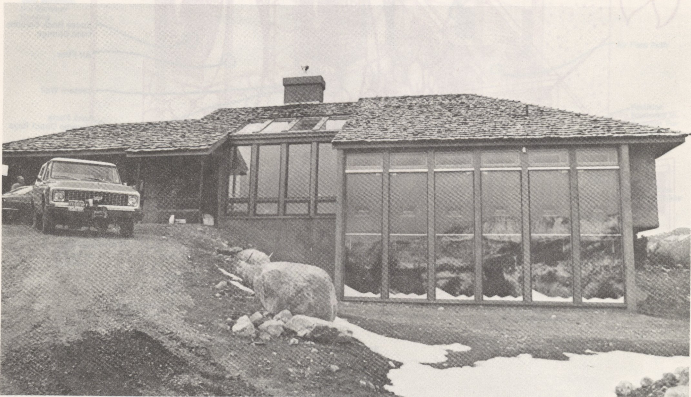
The home of Paul and Betty Pixler in Durango is totally heated by a Trombe wall and solarium, supplemented by a woodstove.
