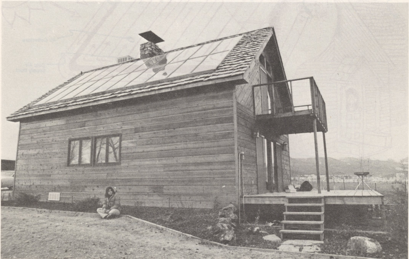
The home of Mr. and Mrs. Beau Foulk in Hotchkiss is heated by a commercially available active air collector system with eutectic salt trays for heat storage.
