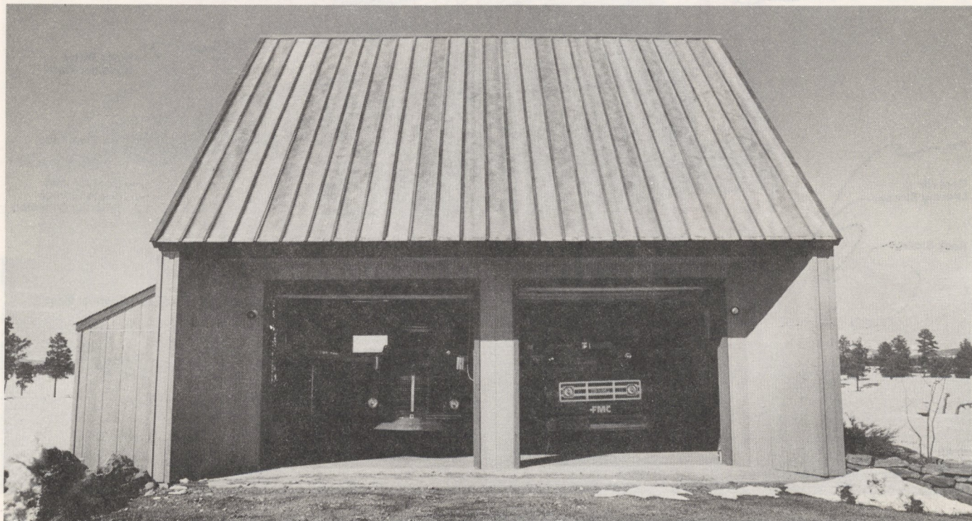
The fire station in Pagosa Springs is about 70 percent solar-heated by a fan-powered air collector built into the roof.
