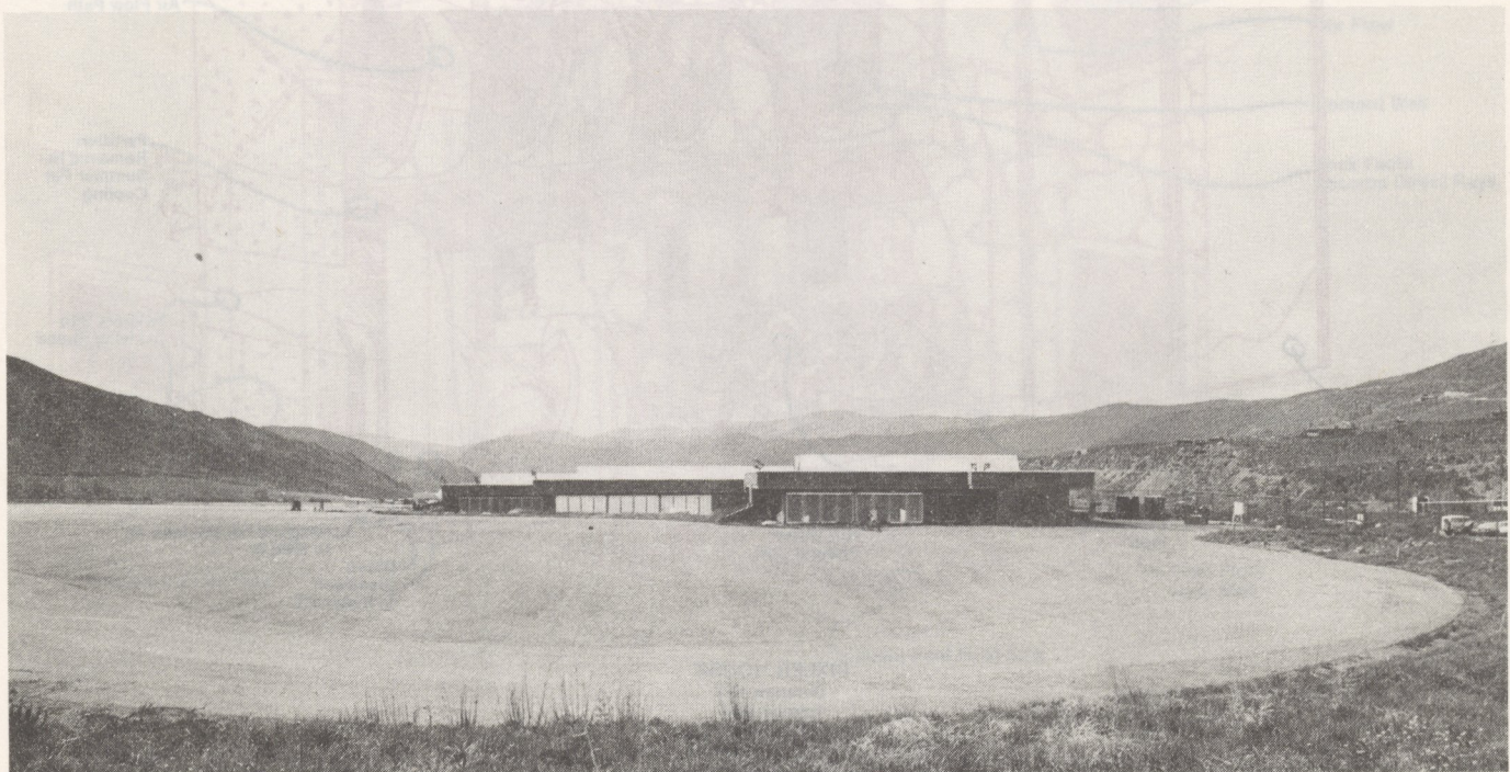
The Pitkin County Airport in Aspen is heated by a direct gain passive solar system with movable insulation.
