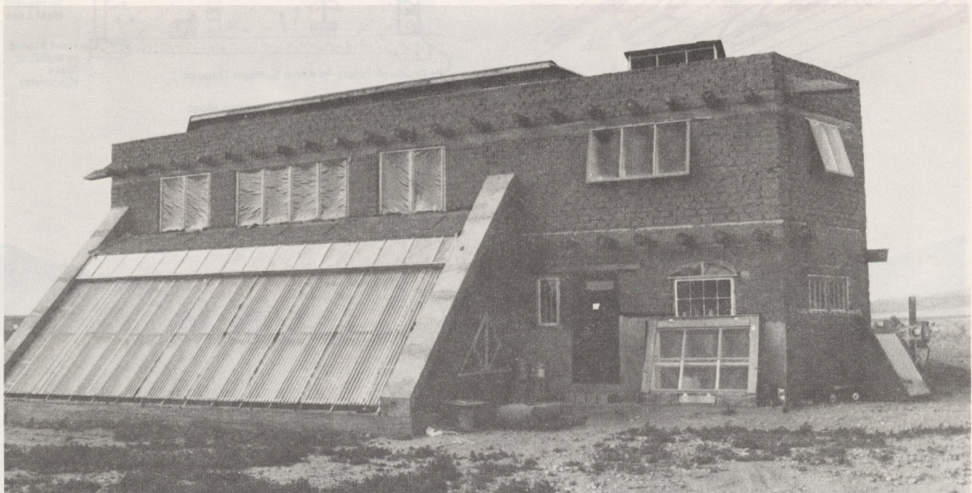
The home of Arnie and Maria Valdez in San Luis is a massive adobe structure with a greenhouse, solar water heaters, a solar food dryer and a woodstove.
