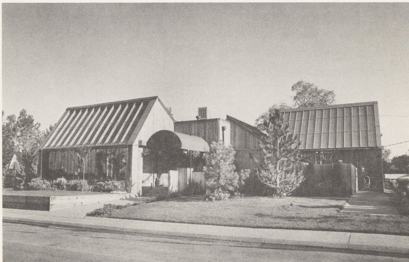
Rick's Cafe in Denver combines active and passive solar systems for heating, dishwashing and ventilation.
