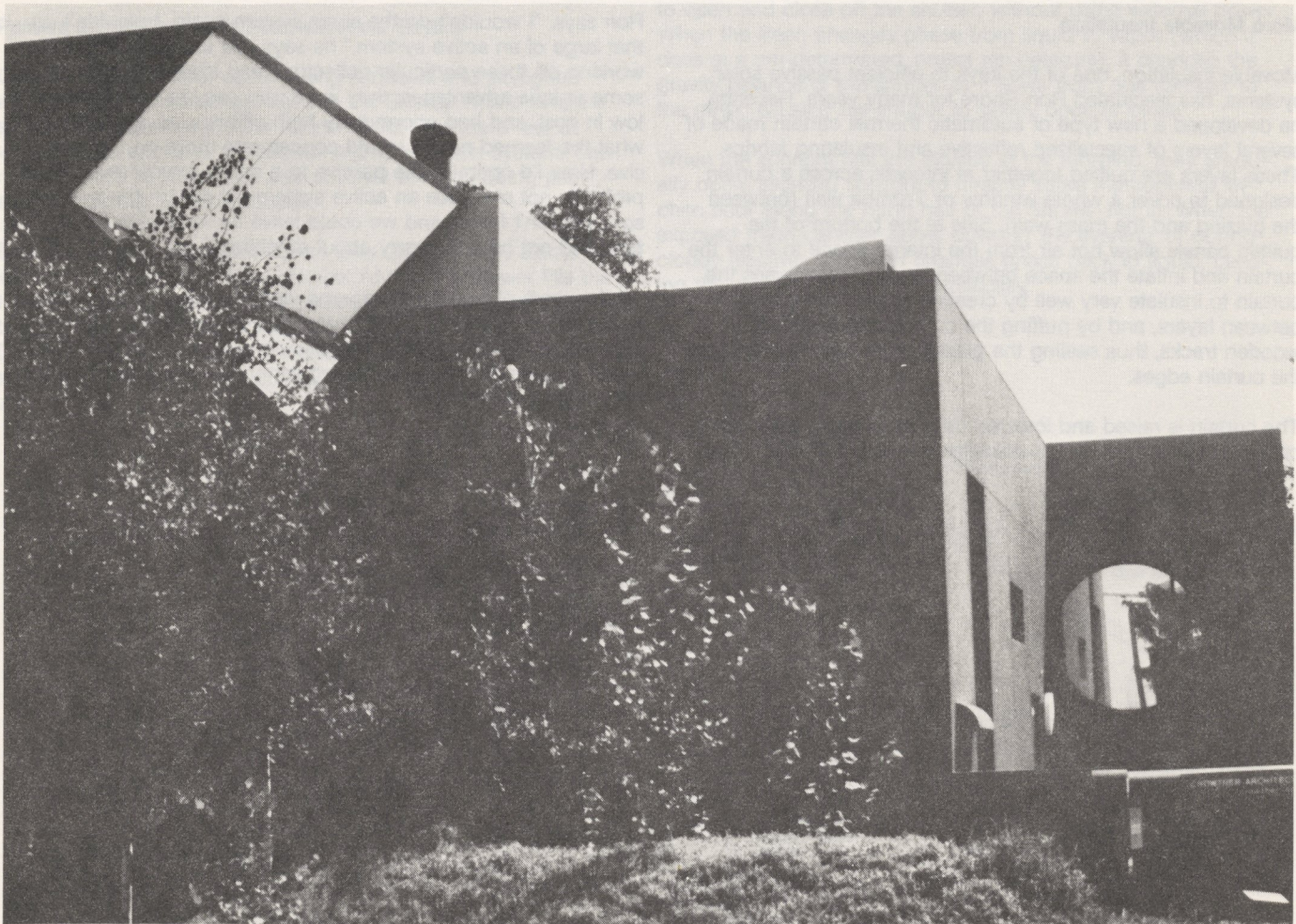
By intelligent design which uses the energy of the sun, the wind and the earth, Dick Crowther has reduced the amount of electrical energy required to heat his Cherry Creek office building in Denver by 80 percent.
