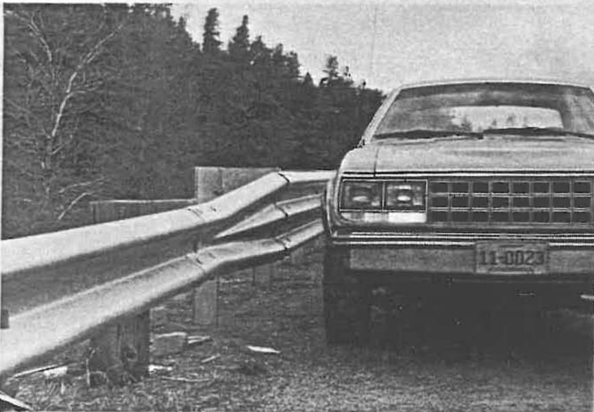
Photo 4. Thrie-beam to w-beam transition at lower end of Hesperus project.
