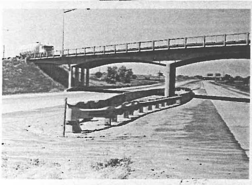
Photo 6. Type 3F on I-76 at milepost 16.95. End treatment transitions to concrete jersey barrier.
