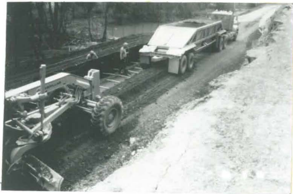
FIGURE 5 - PLACING BACKFILL SOIL TO COVER THE REINFORCING STRIPS
