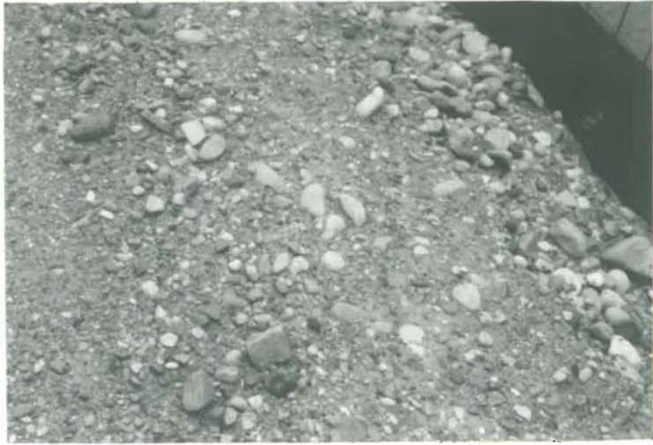
FIGURE 6 - CLOSE UP OF THE BACKFILL MATERIAL
