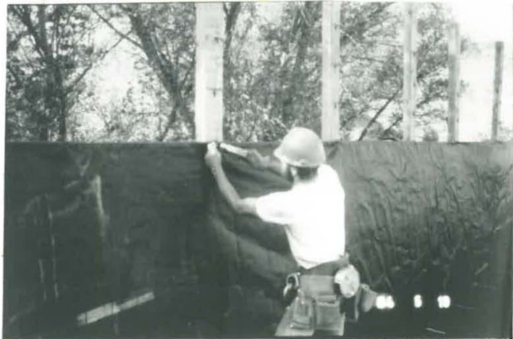
FIGURE 3 - NAILING THE REQUIRED GEOTEXTILE FABRIC TO THE FASCIAL WOODEN FRAME
