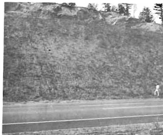
October About 40% Plant Cover Gullys Appearing In Slope
