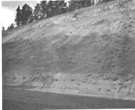
Mid June A Few Weeds Formed Very Little Erosion Protection
