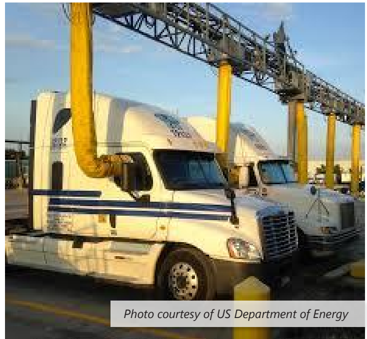
FIGURE 4-10 EXAMPLE OF OFF-BOARD TRUCK STOP ELECTRIFICATION
