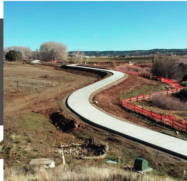
Wilson Gulch multiuse path along US 160 Photo Credit: CDOT
