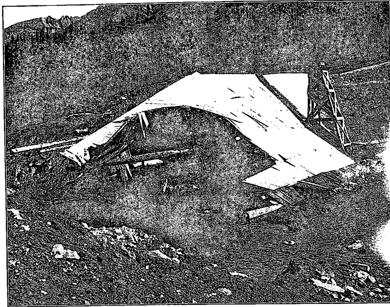
MIDDLE RESERVOIR OF TELLURIDE POWER COMPANY. Upper face of dam from break. October 2, 1909.
