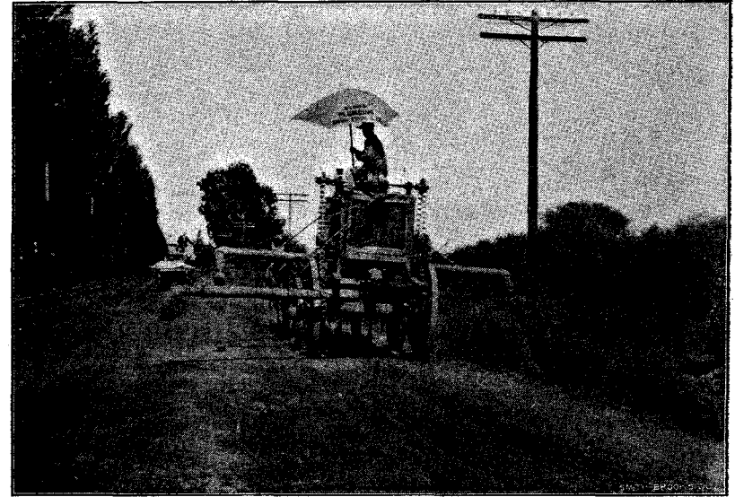
CALIFORNIA ROAD SPRINKLER.
