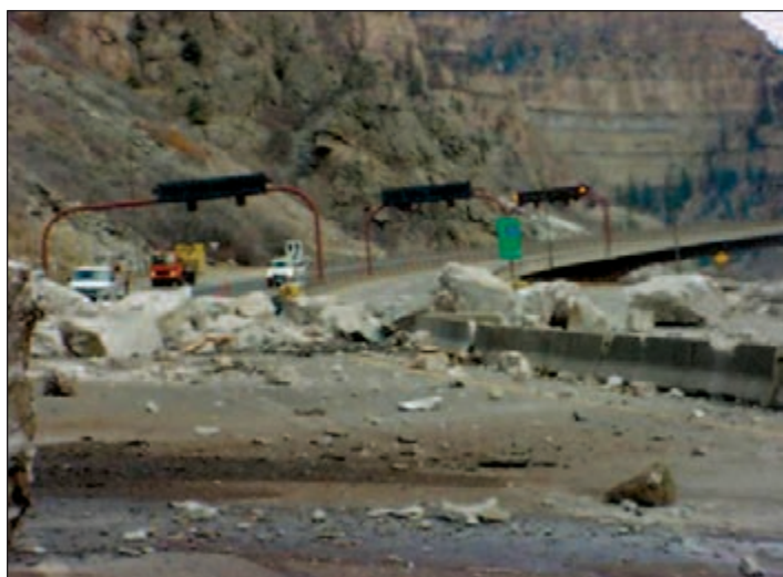
Figure E: Huge blocks of sandstone litter both east and westbound I-70.
