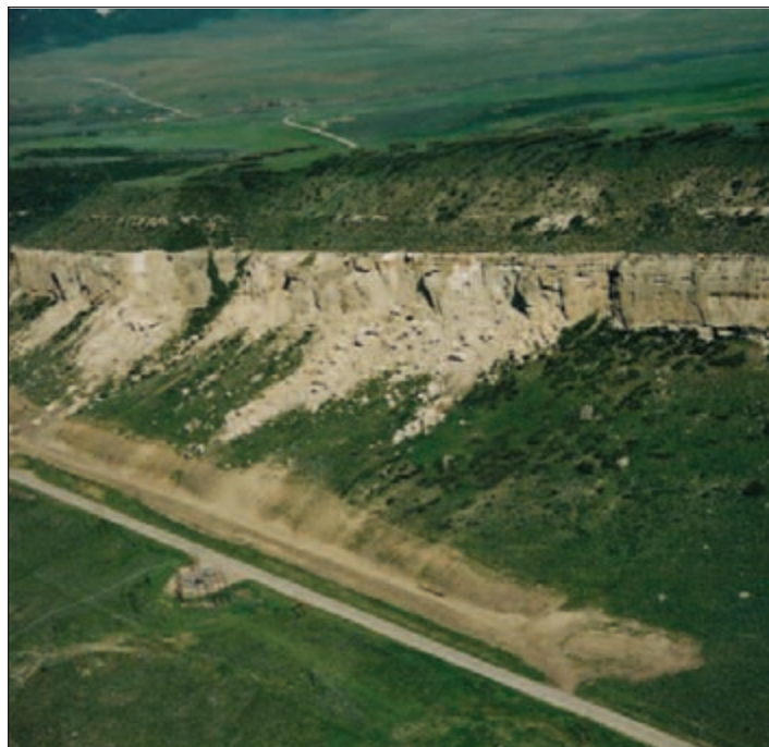
Figure J: Subsidence of the Foidel Creek Mine resulted in rockfall in the Twentymile Sandstone cliff face. Note rockfall ditch and berm above roadway. (Photo courtesy of Colorado Division of Reclamation, Mining, and Safety.)
