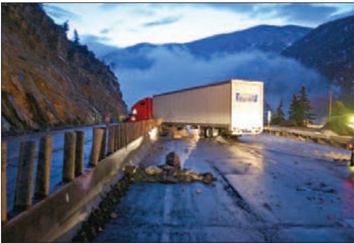
A semi-truck collided with a fallen rock on Interstate 70 near Georgetown in April, 2004. Fallen rocks around bends in the highway or night-time rockfalls may not be visible to drivers, and can lead to accidents. (Photo by CDOT, 2004)
