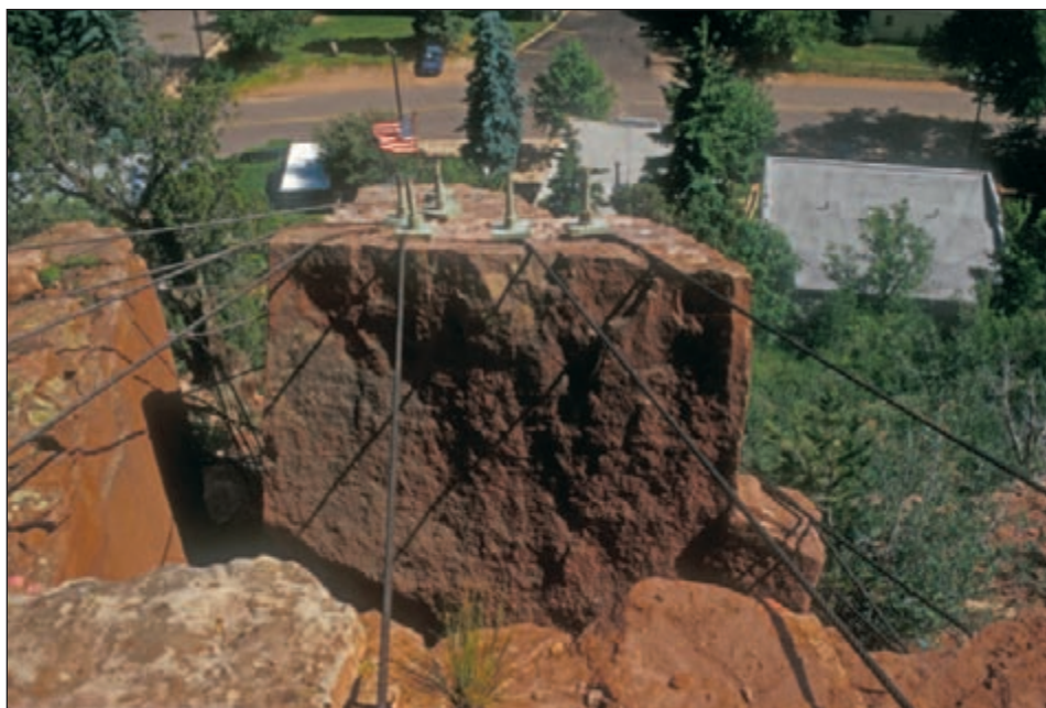
Figure I: After the rock was stabilized, additional cables were physically attached to the top of the rock block and secured to surrounding stable rock. (Photo by Jon White.)
