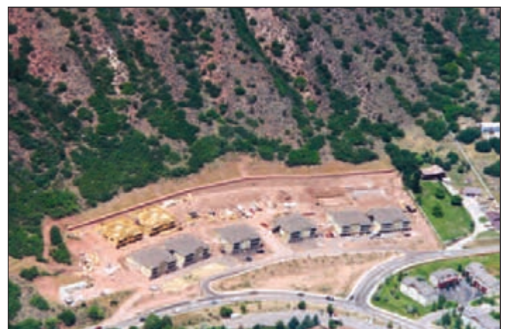
Figure C: This newer development in west Glenwood Springs constructed a rockfall impact wall above their townhomes to protect against both rockfall and mudslides (debris flows). (Photo by Jon White.)
