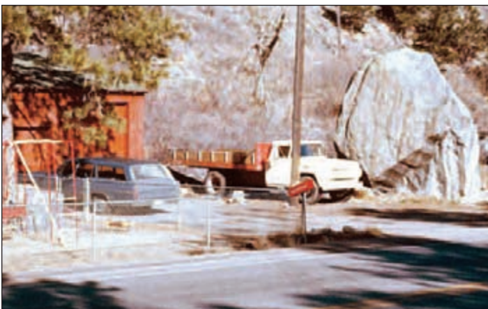
The large rock (right) fell from cliffs above before this home was built. A similar boulder falling on the house would do considerable damage; however the 1976 Big Thompson flood devastated the canyon and the house first. (Photo by V Matthews)
