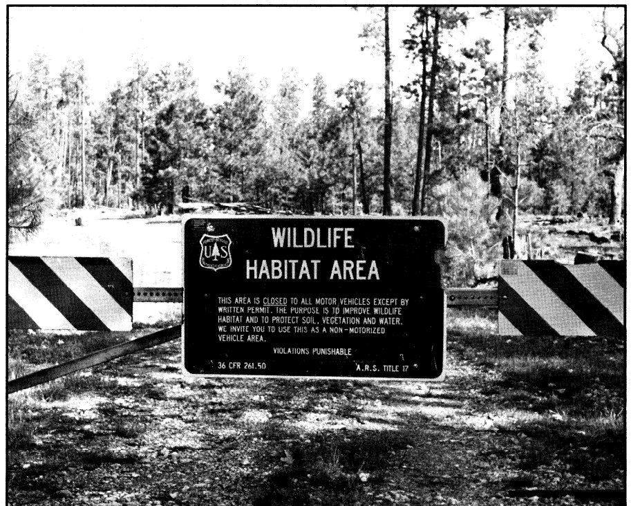
Fig. 22. Road closures may be permanent where access is no longer needed or seasonal, such as only during winter to avoid disturbance in critical roosting or feeding areas.
