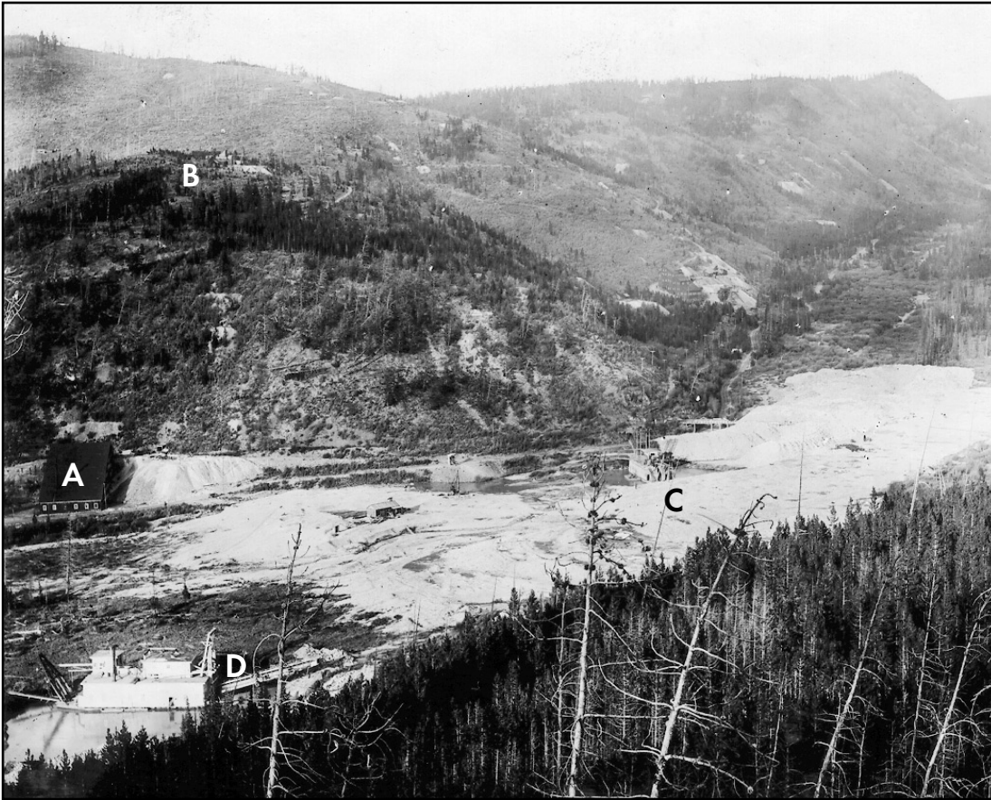
Union Mine and Mill in French Gulch, Summit County, 1909; A) Union mill and adit; B) Union shafts; C) Reliance dredge; and D) Reiling dredge
