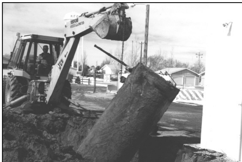
Removal of underground storage tank at a state facility PHOTO BY TY ORTIZ
