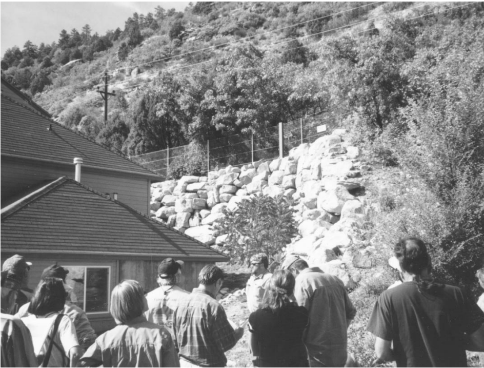
Geologic Hazards Field Trip, Durango GeoConference: Field trip leader, David Trautner of Lambert & Associates, describes a rockfall fence at the Mercy Housing Project in north Durango
